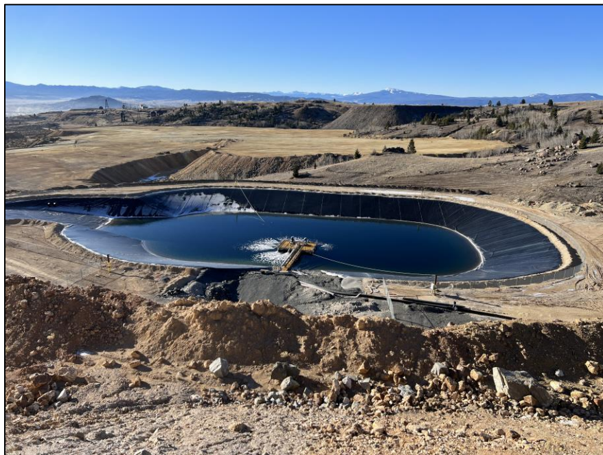
PHOTO 4 – November 28, 2023 – WED Extraction Pond and Dewatering System.
