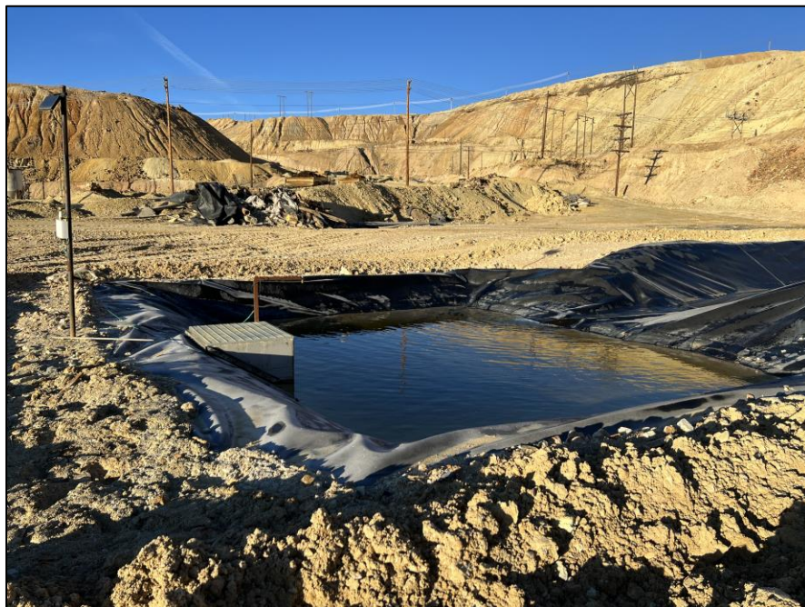
PHOTO 2 – November 28, 2023 – Seep 10 Stilling Pond
