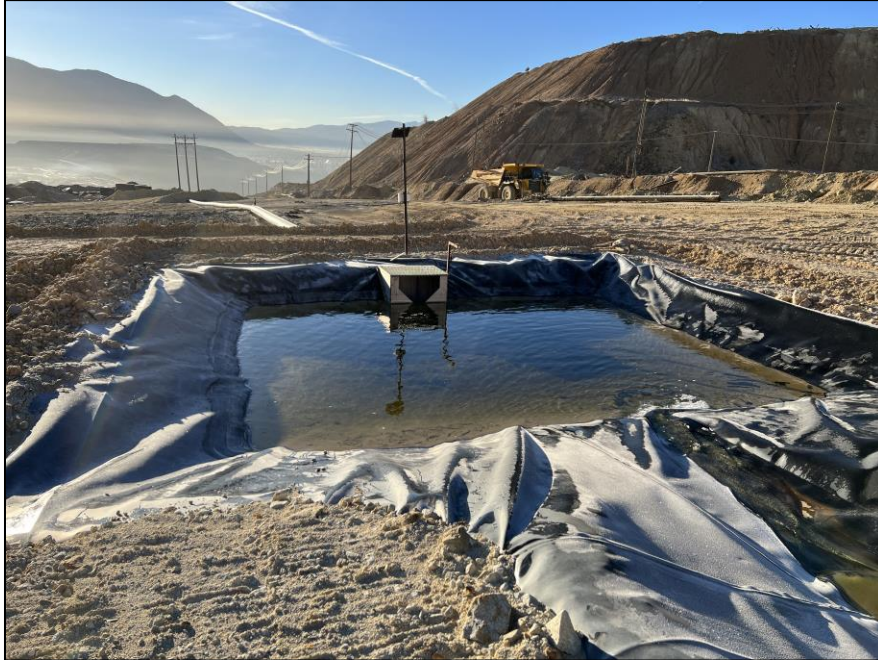
PHOTO 3 – November 28, 2023 – Seep 10 Weir.
