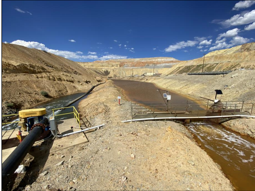
PHOTO 1 – August 29, 2023 – BPPS Transfer Pond (left) and HsB Weir (right).
