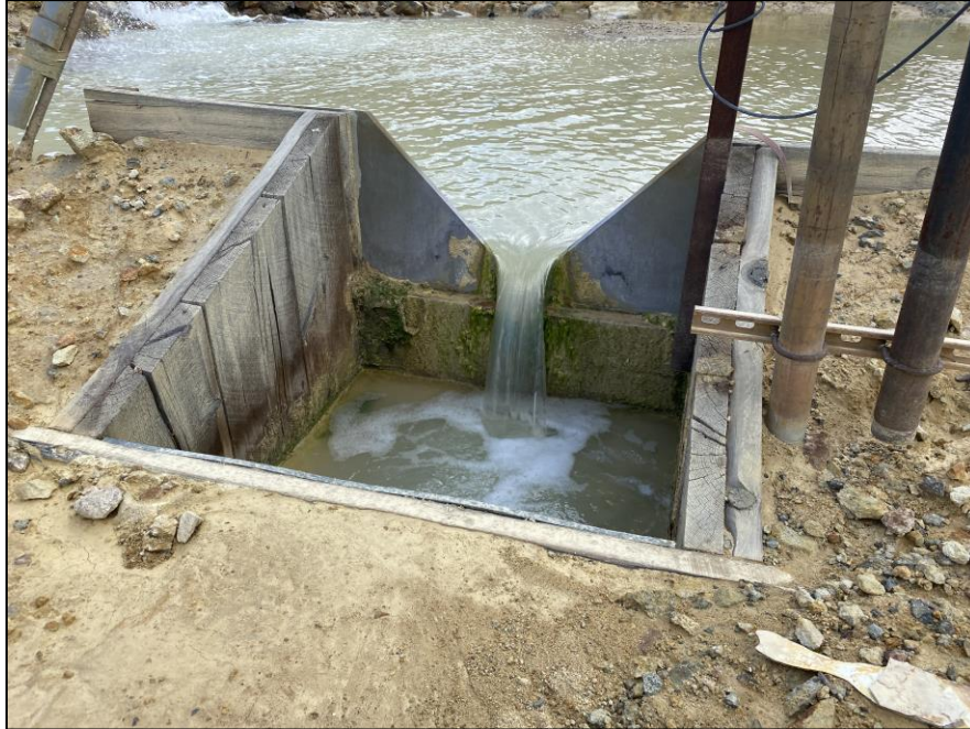
PHOTO 3 – August 30, 2023 – Seep 10 Weir.
