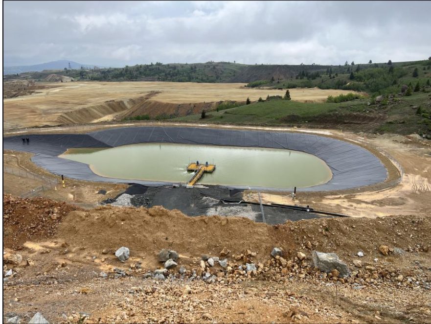
PHOTO 3 – June 12, 2023 – WED Extraction Pond and Dewatering System.
