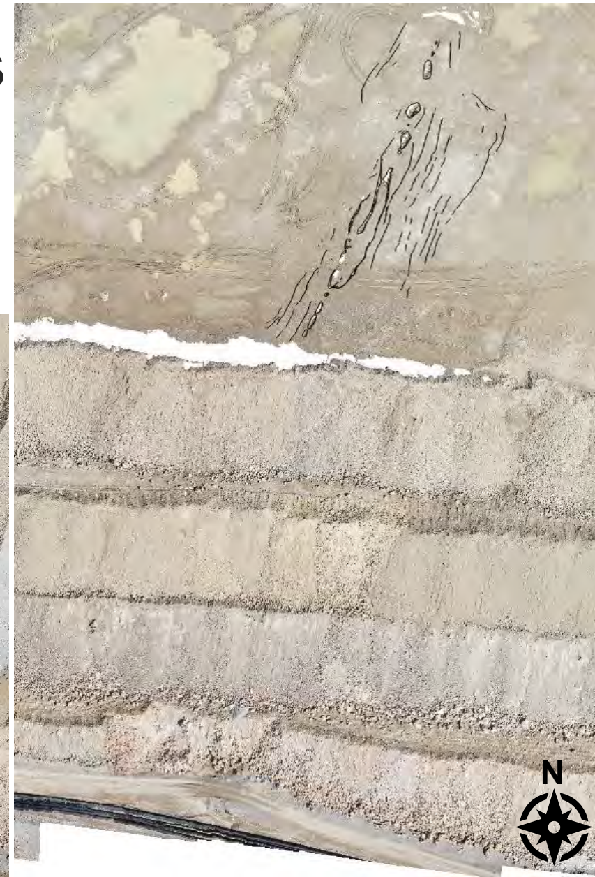
Downstream Slope of CPA Embankment (April 28, 2023)
