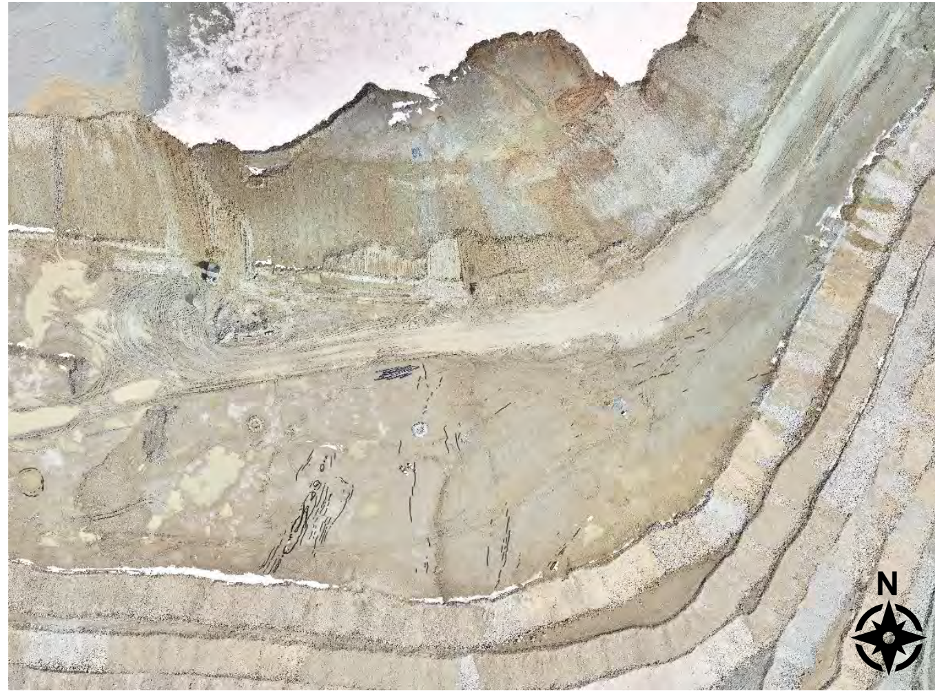
Upstream Slope of Rockfill Surcharge (April 28, 2023)
