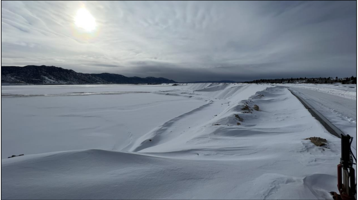
Photo 7.1 Tailings discharge adjacent to the West Embankment – March 1, 2023.
