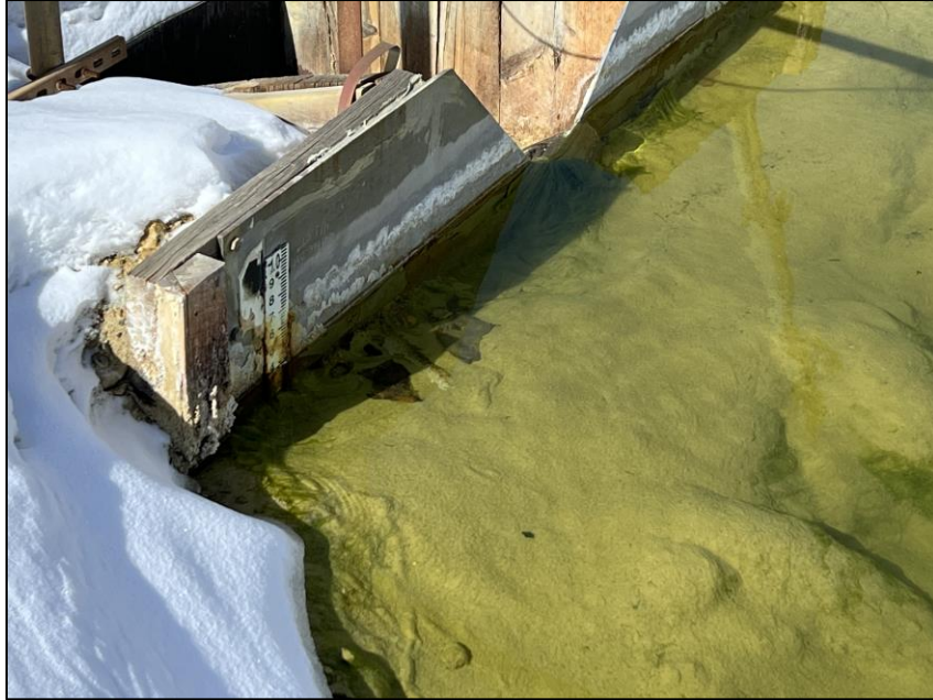
PHOTO 3 – March 1, 2023 – Seep 10 Weir and Staff Gauge, reading slightly below 0.4.
