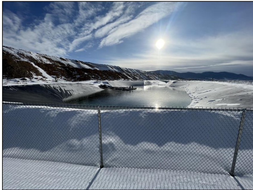
PHOTO 4 – March 1, 2023 – WED Extraction Pond and Dewatering System.
