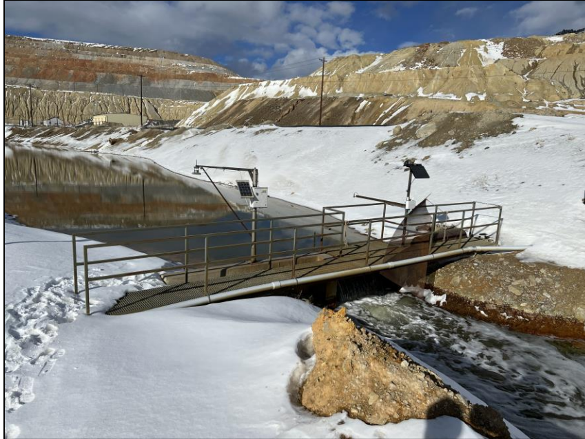
PHOTO 1 – March 1, 2023 – Flow through HsB Weir.
