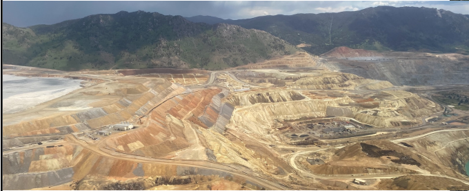
Aerial view looking East along East-West Embankment towards Horseshoe Bend (HsB)
