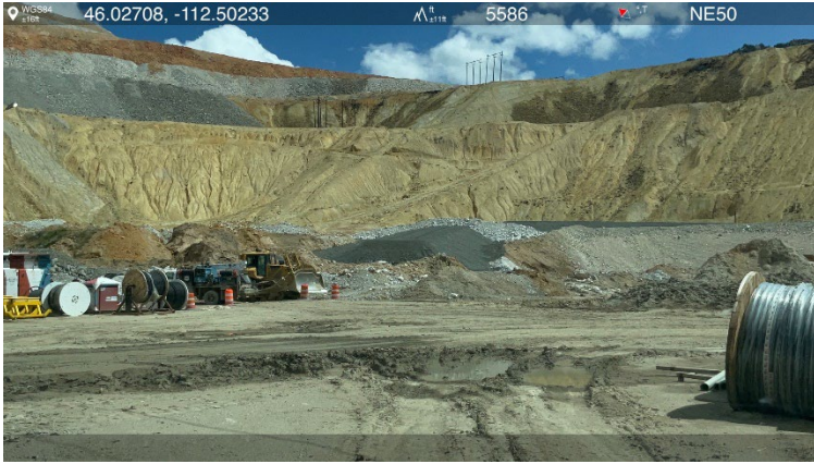
Photo 12- The 3-layer rock drains are being constructed on top of the foundation drainage layer, some portions have not yet been constructed. Photo 13- The foundation drainage layer continues to be constructed prior to placement of Pipestone drain rock.
