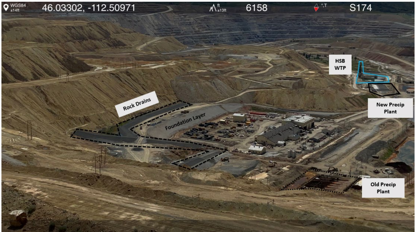
Photo 11- The HSB overlook near Tailings Booster Station #3, major features from the report are outlined and labeled.
