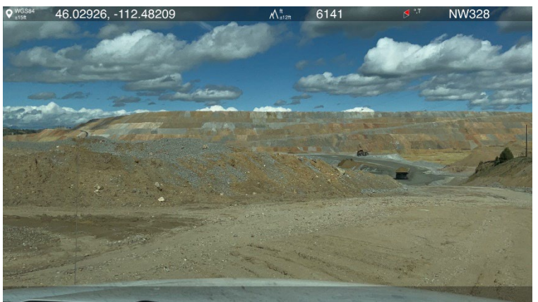
Photo 3- The backside of the highwall and soil salvage area in Photo 2 (from Interstate 15, northbound). Photo 4- Haul trucks moving non-ore rock, only small portions of the YDTI embankment crests have not been constructed to the 6,450 ft elevation.
