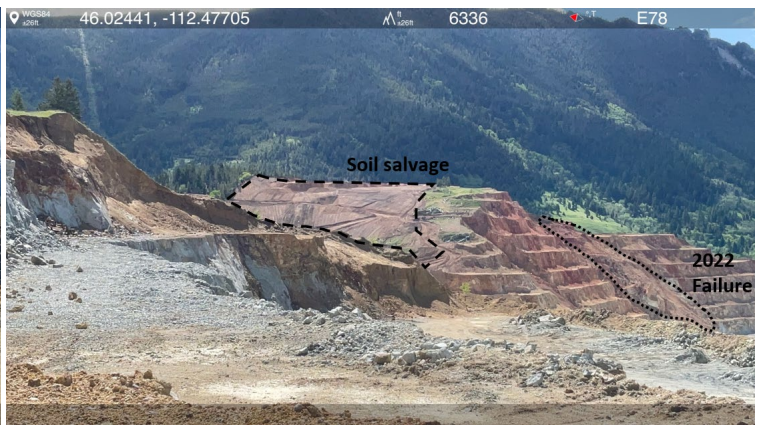
Photo 1- A failure occurred in the central portion of the D East highwall on November 1, 2022, which is a relatively small area in the Continental Pit (left side of photo). Photo 2- Vegetation removal and soil salvage has occurred to the east of the highwall as part of constructing an access ramp.
