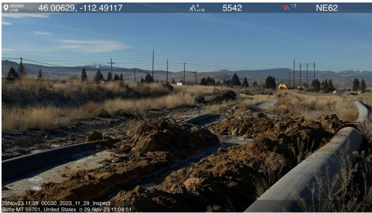
Photos 5 and 6: In addition to the immediate response measures, further earthwork was being performed to expand the trench and channel system and to raise the elevation of the adjacent berm/bank (Photos 5 through 7).
