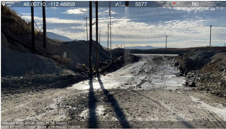
Photo 1: The source location of the process solution release was a truck fill station that is used for water trucks (52,000 gallons) conducting fugitive dust management. Photo 2: The flowing water entered a culvert near the fill station and was diverted beneath the nearby haul road.
