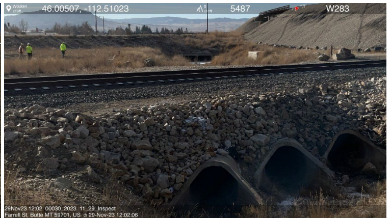
Photo 11: The flow was contained within the open channel of the CRC and segments that consist of culverts or concrete channels. Photo 12: The flowing water ultimately ended with pooling in the sediment pond located at the western end of the CRC.
