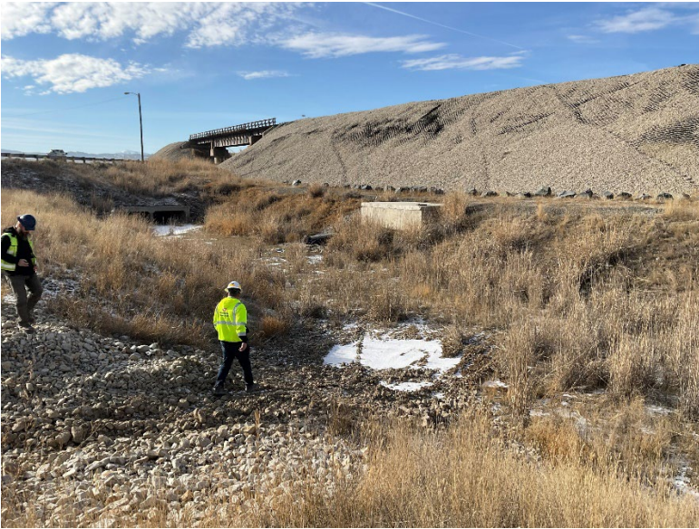
Photo 13: This location is the northern extent of the upper Silver Bow Creek channel, formerly known as Metro Storm Drain. This feature conveys runoff from the area but does not contain perennial flow.
