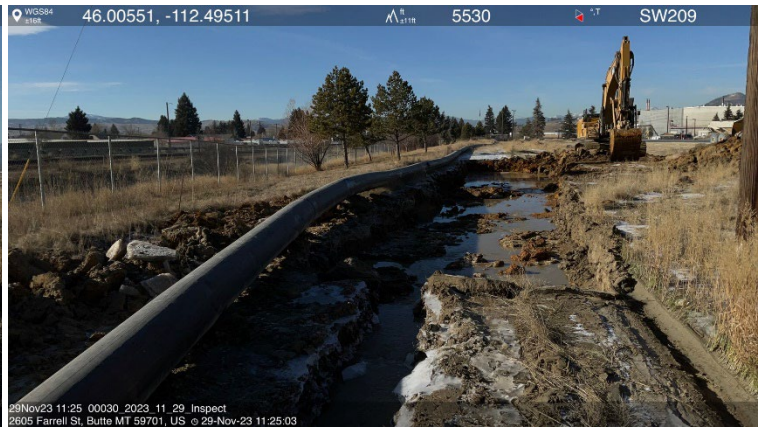
Photos 5 and 6: In addition to the immediate response measures, further earthwork was being performed to expand the trench and channel system and to raise the elevation of the adjacent berm/bank (Photos 5 through 7).
