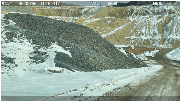
Photo 11- Stockpiles of rock from the Pipestone Quarry have been placed within the HSB area, awaiting placement and drain construction. Photo 12- The foundation drainage layer was being placed during the inspection, prior to the construction of rock drains.
