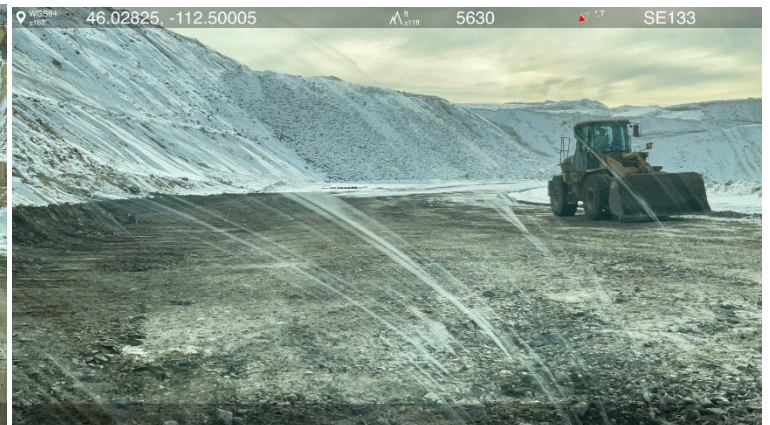
Photo 11- Stockpiles of rock from the Pipestone Quarry have been placed within the HSB area, awaiting placement and drain construction. Photo 12- The foundation drainage layer was being placed during the inspection, prior to the construction of rock drains.
