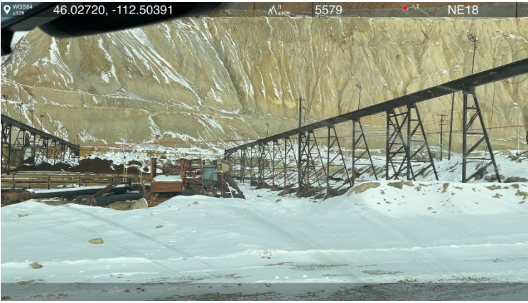
Photo 15- The historical copper precipitation plant has been undergoing demolition in preparation for the RDS construction, though some portions of the plant are still operational at decreased capacity. Copper is being recovered from water pumped out of the Berkeley Pit, when not disrupted by freezing conditions. Photo 16- A new precipitation plant is being constructed to the south of HSB, near the HSB Water Treatment Plant. This facility was approved as revision MR 22-001.
