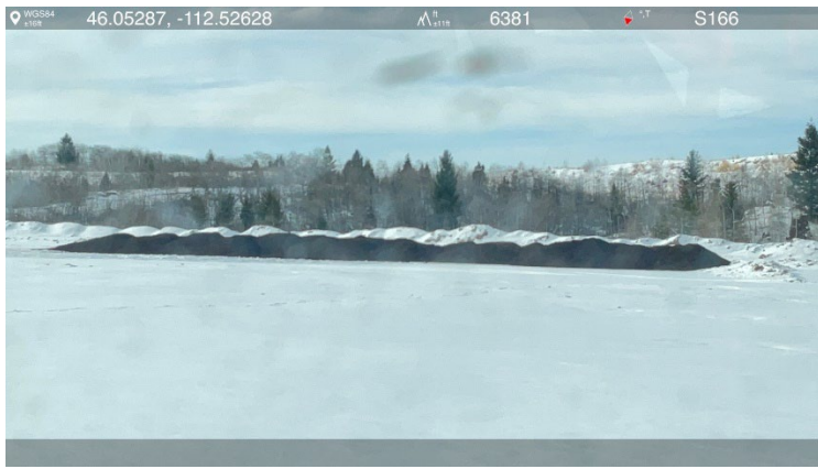
Photo 8- Compost is being stockpiled along a portion of the West Embankment, to be mixed with soil during concurrent reclamation. Photo 9- The interior/upstream face of the West Embankment, with tailings discharge lines across the slope.
