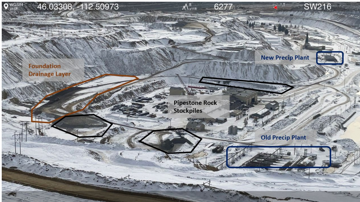
Photo 10- The HSB overlook near Tailings Booster Station #3, major features from the report are outlined and labeled.
