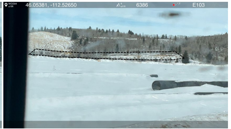
Photo 8- Compost is being stockpiled along a portion of the West Embankment, to be mixed with soil during concurrent reclamation. Photo 9- The interior/upstream face of the West Embankment, with tailings discharge lines across the slope.
