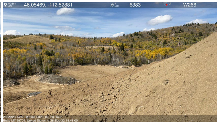
Photo 11- Equipment is placing and pushing soil along the West Embankment. Photo 12- Looking at the outer slope of the West Embankment, drain rock is visible at the bottom. Soil stockpiles in the distance have vegetation established and serve as visual barriers.
