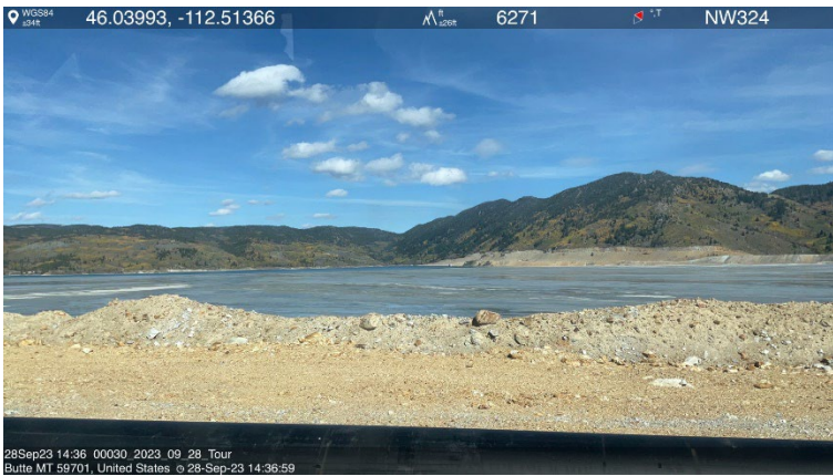
Photos 7 and 8- Additional tailings discharge lines allow greater flexibility for selectively applying tailings slurry in areas that might become dry and prone to blowing dust, and to control the uniform development of the beach and pond areas. The internal face of the embankment has been covered with alluvium and graded. The rocks and vegetation in Photo 8 are the remaining exposure of “Rocky Knob.”
