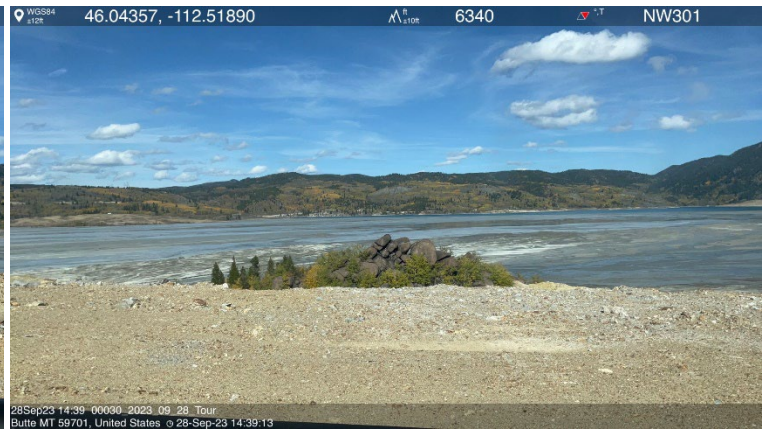
Photos 7 and 8- Additional tailings discharge lines allow greater flexibility for selectively applying tailings slurry in areas that might become dry and prone to blowing dust, and to control the uniform development of the beach and pond areas. The internal face of the embankment has been covered with alluvium and graded. The rocks and vegetation in Photo 8 are the remaining exposure of “Rocky Knob.”
