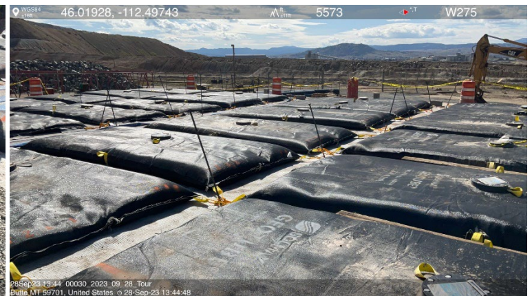
Photos 3 and 4- The piping and valve system used to discharge precipitated sludge into the geotubes, which are made of woven synthetic materials.
