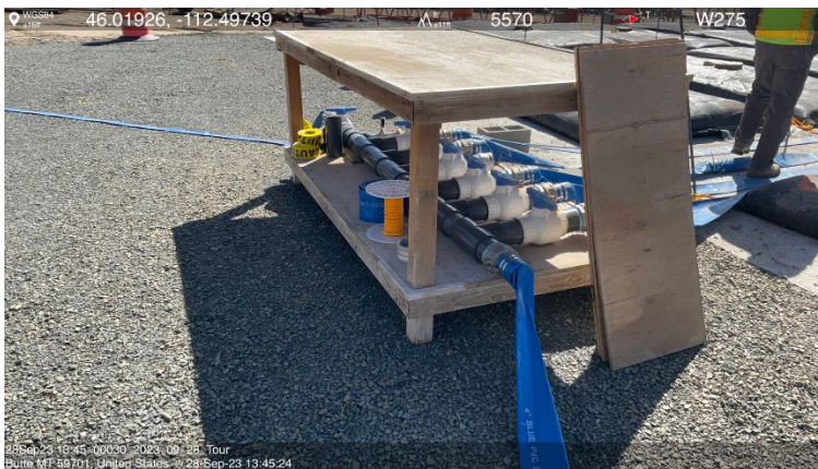
Photos 3 and 4- The piping and valve system used to discharge precipitated sludge into the geotubes, which are made of woven synthetic materials.
