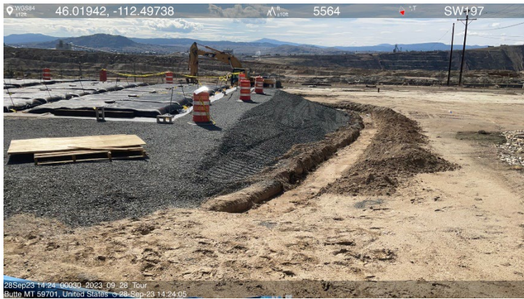
Photo 5- A drainage ditch was constructed around the gravel pad to contain water seeping out the geotubes. Photo 6- Sludge samples will be taken out of the geotubes and transported to West Virginia for further analysis.
