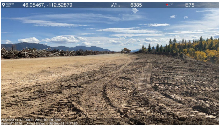
Photo 11- Equipment is placing and pushing soil along the West Embankment. Photo 12- Looking at the outer slope of the West Embankment, drain rock is visible at the bottom. Soil stockpiles in the distance have vegetation established and serve as visual barriers.
