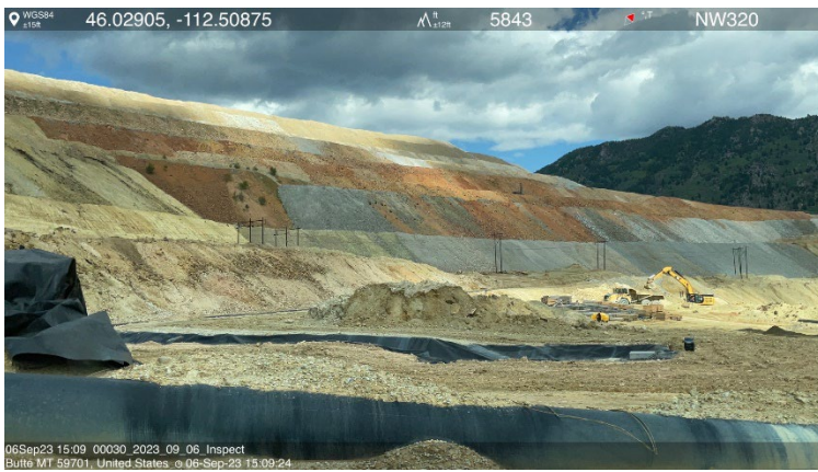
Photo 12- A lined channel and pipeline system is being constructed to divert Seep 10 flows around the future HSB RDS area. Photo 13- Pilot scale testing for REE/CM recovery will begin later in September 2023, which would involve the placement of “geotubes” on a gravel pad area that is adjacent to the current plant facility.
