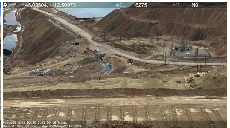
Photo 10- A new precipitation plant is being constructed to the south of HSB, near the HSB Water Treatment Plant. This facility was approved as revision MR 22-001. Photo 11- A lined channel and pipeline system is being constructed to divert Seep 10 flows around the future HSB RDS area.
