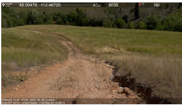
Photo 5- The primary access road on the East RDS has been eroded by recent storm events, preventing light vehicle traffic. When practicable, this feature should be repaired to restore access. Photo 6- A failure occurred in the central portion of the D East highwall in 2022, vegetation removal and soil salvage has occurred to the east (right) of the highwall as part of constructing an access ramp for the layback.
