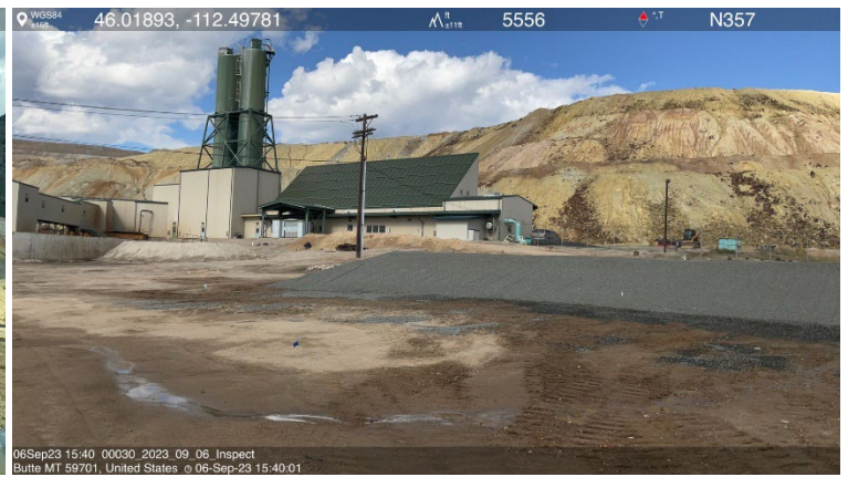
Photo 12- A lined channel and pipeline system is being constructed to divert Seep 10 flows around the future HSB RDS area. Photo 13- Pilot scale testing for REE/CM recovery will begin later in September 2023, which would involve the placement of “geotubes” on a gravel pad area that is adjacent to the current plant facility.
