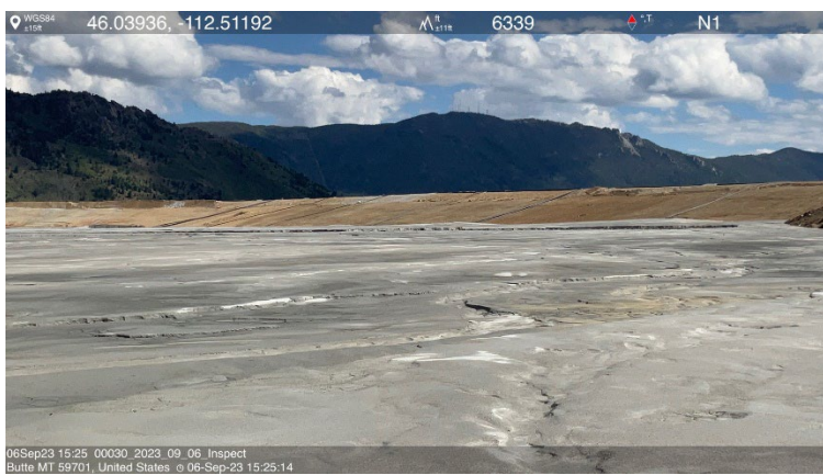
Photo 7- Additional tailings discharge lines allow greater flexibility for selectively applying tailings slurry in areas that might become dry and prone to blowing dust, and to control the uniform development of the beach and pond areas. The internal face of the embankment has been covered with alluvium and graded. Photo 8- As seen across the extent of the tailings beach, soil salvage is occurring along the north end of the West Embankment.
