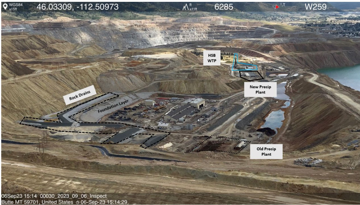
Photo 9- The HSB overlook near Tailings Booster Station #3, major features from the report are outlined and labeled.
