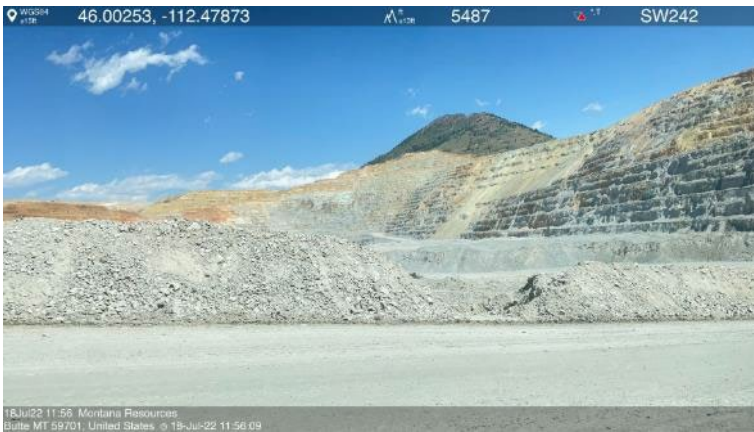
Photo 16- Mining continues within the D East, D North, and C Block portions of the Continental Pit. Photo 17- The west highwall of Continental Pit, which reveals the Central Zone alluvium (brown) above an iron-rich oxidized cap (red), which occurs above an enriched ore zone.
