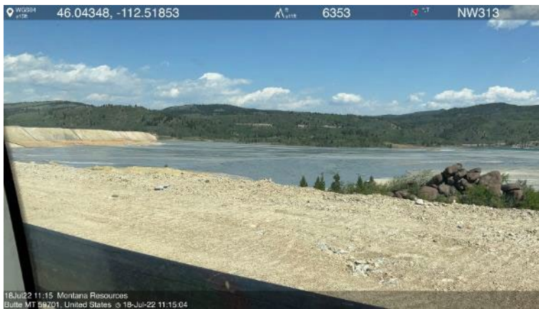
Photo 10- The interior/upstream face of the West Embankment, with tailings discharge lines across the slope. Photo 11- The extraction pond at the south end of the WED, where a pump barge is used to circulate water back into the YDTI.
