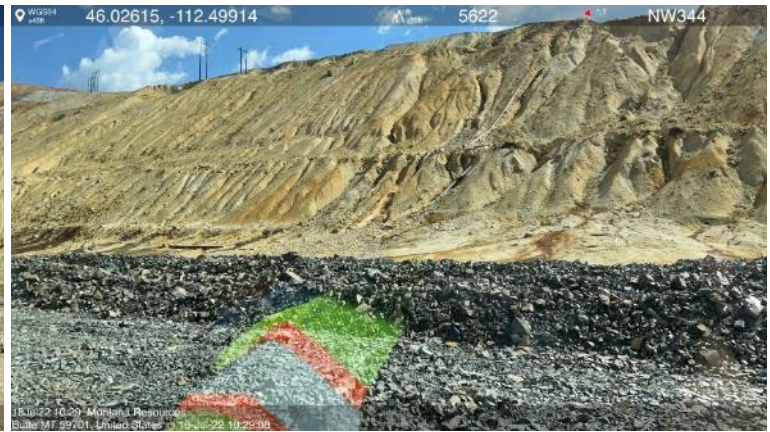
Photo 2- Stockpiles of drain rock from the Pipestone Quarry have been staged around the HSB area for future construction of a foundation drainage layer and engineered rock drains. Photo 3- Some fill material and drain rock have also been placed around the east side of HSB, to assist with compaction and drainage of the collection ponds at the toe of adjacent leach pads.
