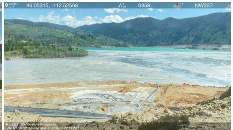
Photo 10- The interior/upstream face of the West Embankment, with tailings discharge lines across the slope. Photo 11- The extraction pond at the south end of the WED, where a pump barge is used to circulate water back into the YDTI.
