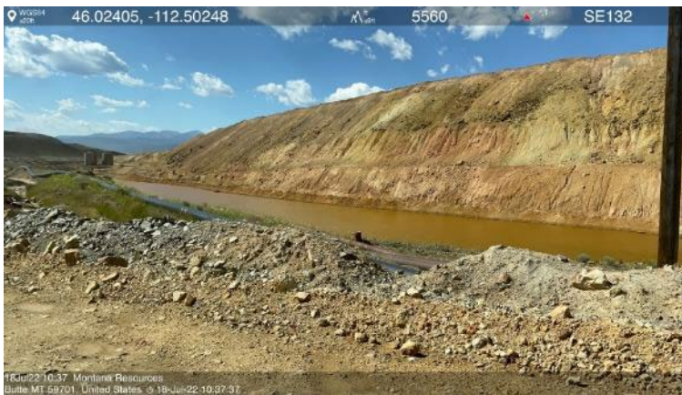
Photo 6- The primary HSB Pond, which contains the multiple sources of seepage that emanate from HSB. From this holding pond, water may be diverted to the HSB Water Treatment Plant or pumped into the YDTI. Photo 7- The old Precipitation Plant is in the process of being demolished, a few components still remain.
