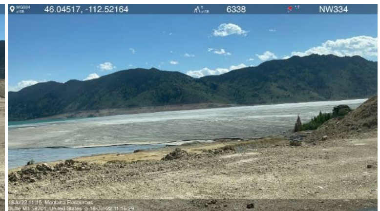
Photo 12- MR has installed storage bladders for magnesium chloride around the YDTI, to speed up the process to deploy and refill tracked vehicles onto the beach. Photo 13- Tracks across the tailings beach and darkened surfaces indicate the proactive efforts to apply magnesium chloride and limit the potential for fugitive dust.
