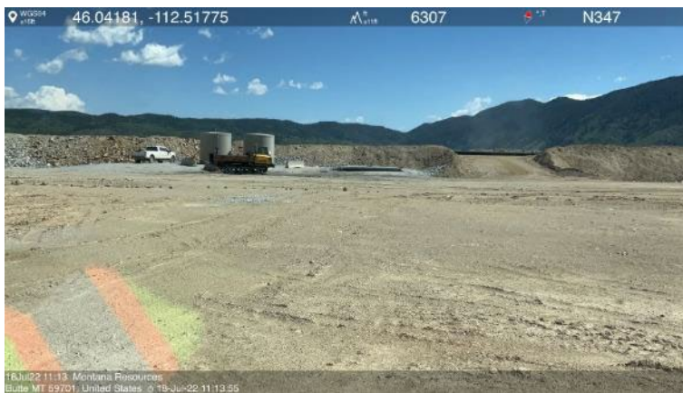
Photo 12- MR has installed storage bladders for magnesium chloride around the YDTI, to speed up the process to deploy and refill tracked vehicles onto the beach. Photo 13- Tracks across the tailings beach and darkened surfaces indicate the proactive efforts to apply magnesium chloride and limit the potential for fugitive dust.
