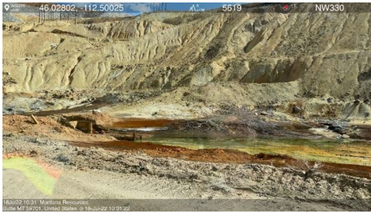
Photos 4 and 5- The former collection ponds have been drained and residual seepage flows are being collected and conveyed to the primary HSB Pond through diversion ditches
