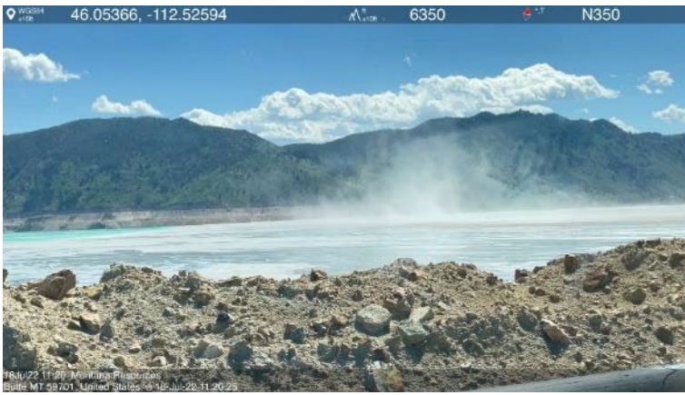
Photo 14: Wind gusts began around 10:00 AM and exceeded 40 mph through midday. The severity of blowing dust would likely have been worse in the absence of the application of magnesium chloride. Photo 15: At the south end of the West Embankment, the lined extraction pond continues to receive the outflow from the WED installed within the embankment's foundation.
