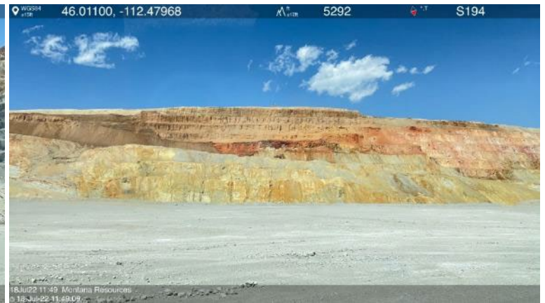
Photo 16- Mining continues within the D East, D North, and C Block portions of the Continental Pit. Photo 17- The west highwall of Continental Pit, which reveals the Central Zone alluvium (brown) above an iron-rich oxidized cap (red), which occurs above an enriched ore zone.
