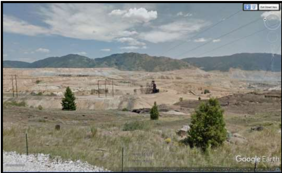
Figure 3.13-4 Views of North-South Embankment and Great Northern RDS from Granite Mountain Memorial via Google Street View.
