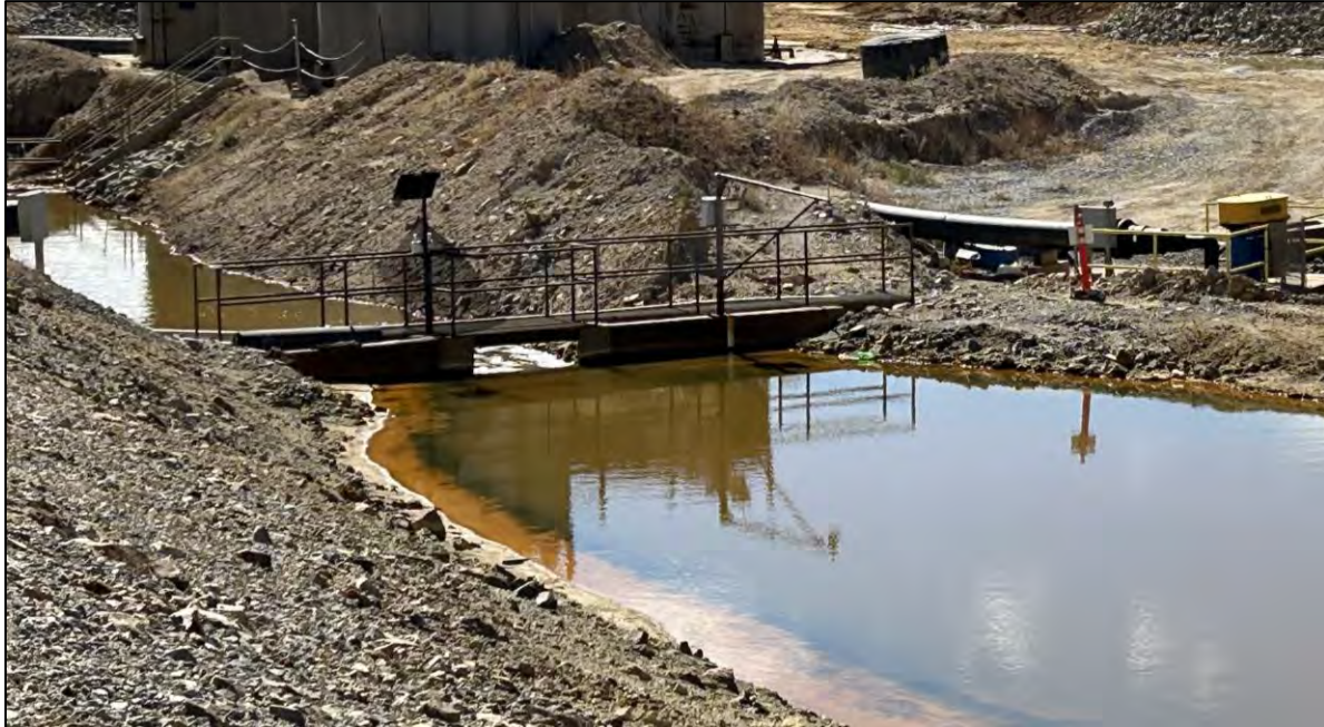
PHOTO 69 – Horseshoe Bend Weir, facing south.
