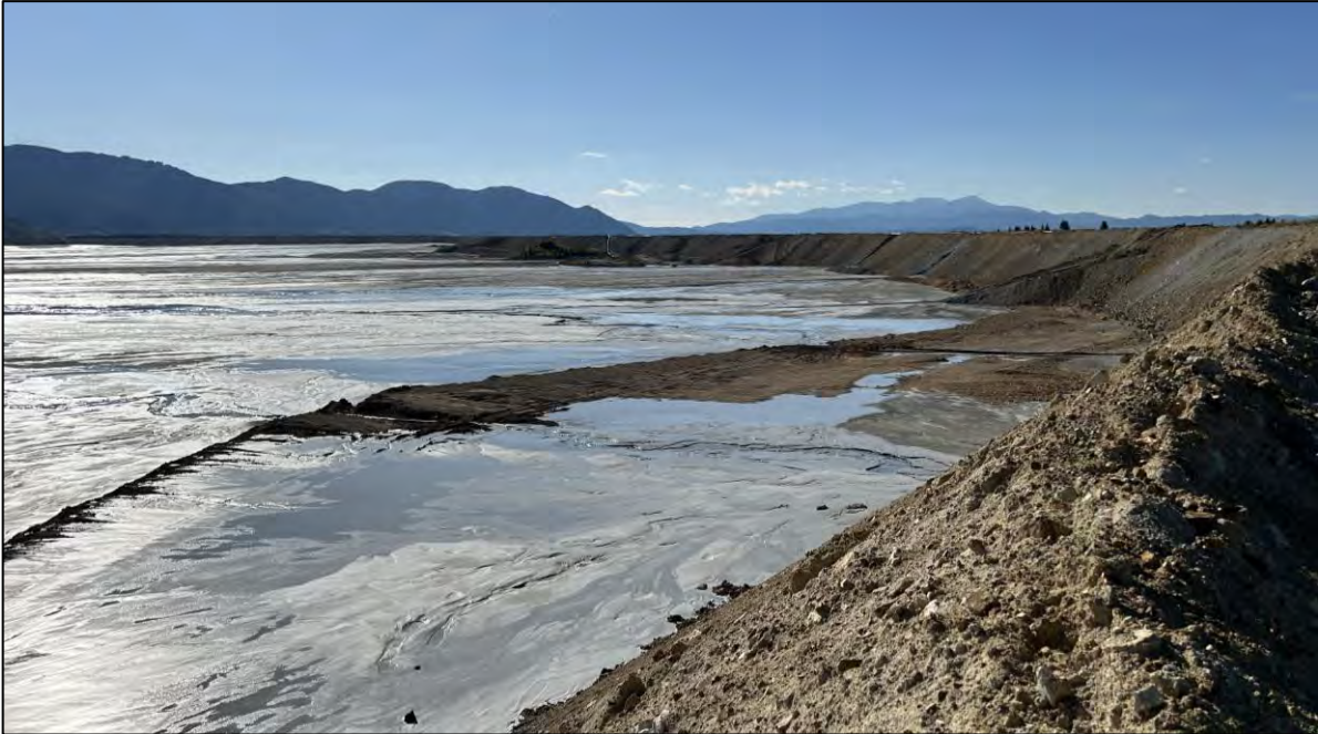
PHOTO 51 – West Embankment upstream shell (right) and tailings beach (left) north of Rocky Knob, facing southeast from EL. 6,450 ft.
