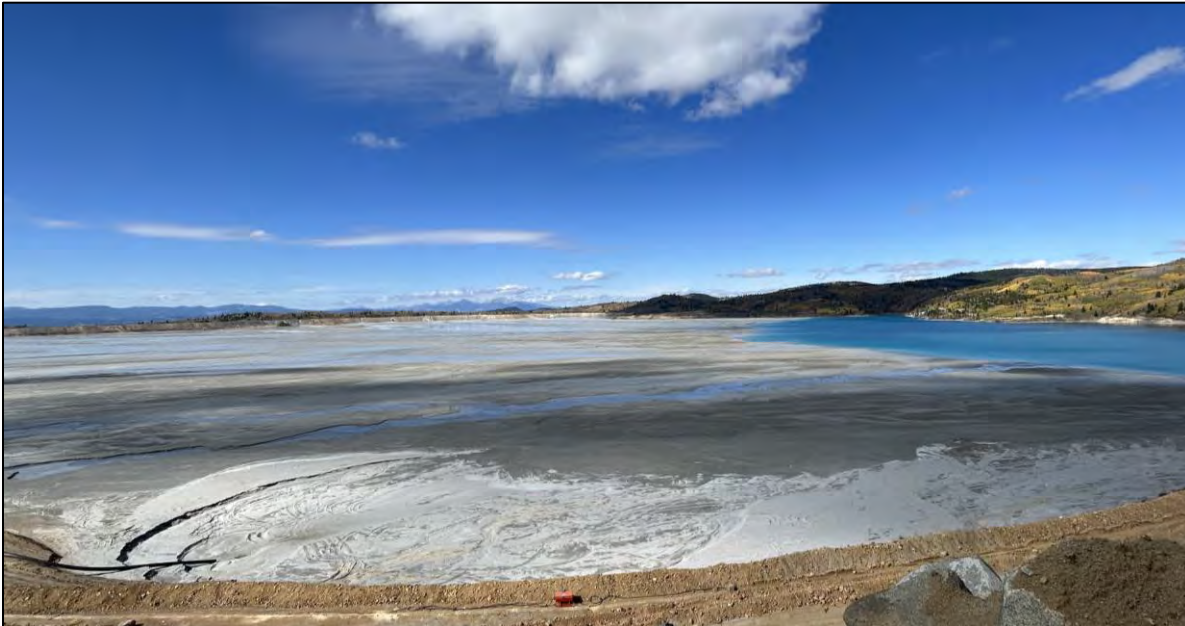
PHOTO 32 – YDTI tailings beach and supernatant pond interface, facing west from the new reclaim pipeline road.
