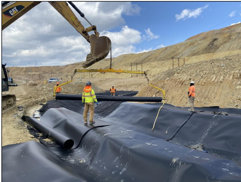
Photo 2.6 Seep 10 SWD #10 Geomembrane Install – Looking West
