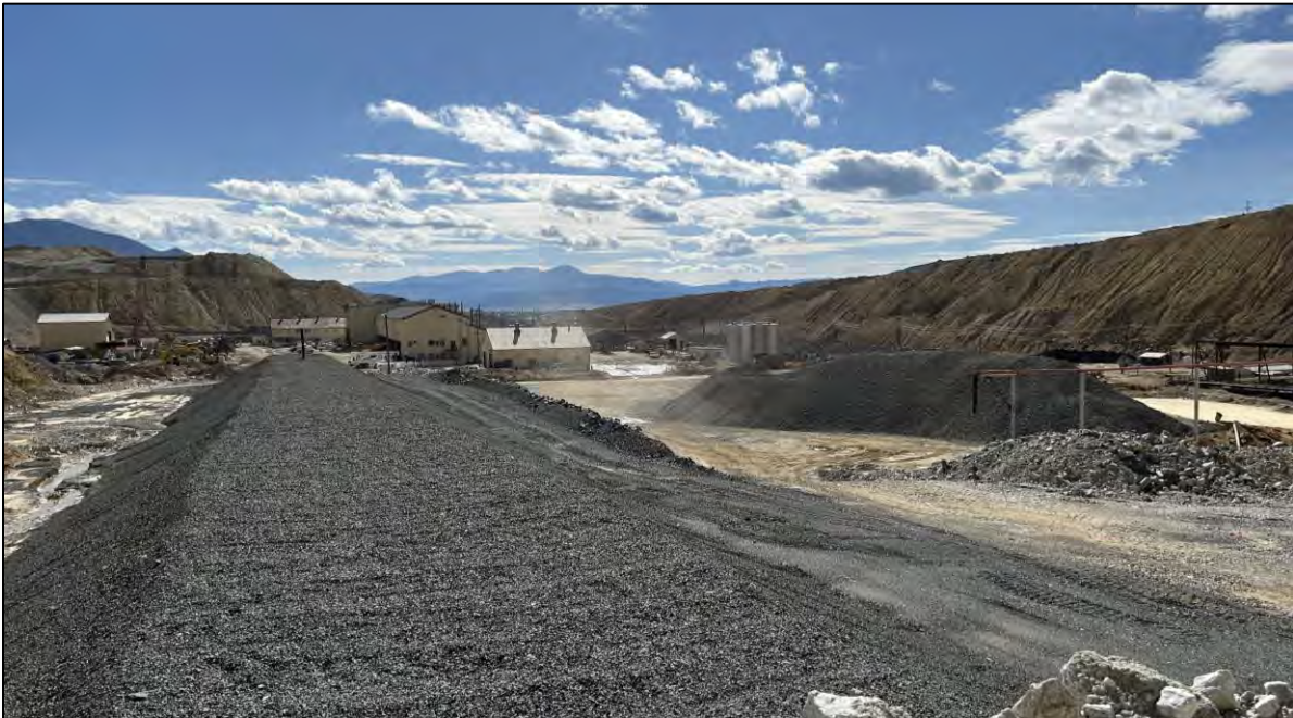
PHOTO 60 – Rock drain D4 construction progress in the HsB Area, facing south.
