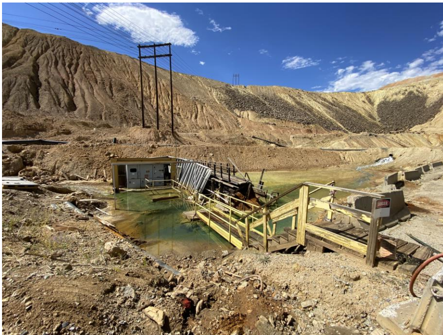
PHOTO 22 – Stage 1 HsB RDS – Old Precip Plant Cell 10 Pump Area
