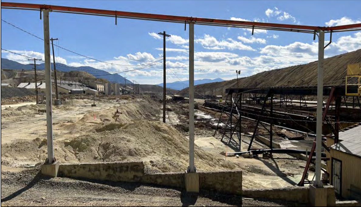
PHOTO 63 – Decommissioned Precipitation Plant awaiting demolition, facing south
