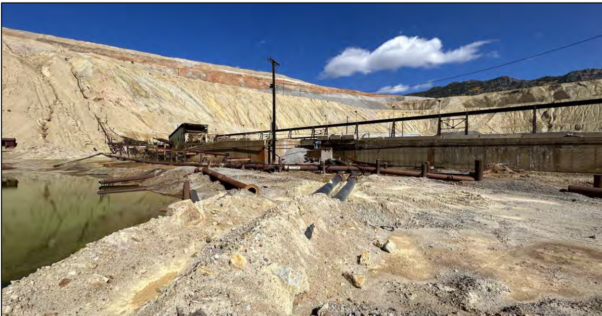
PHOTO 68 – Precipitation plant prior to demolition and salvage, facing northeast.
