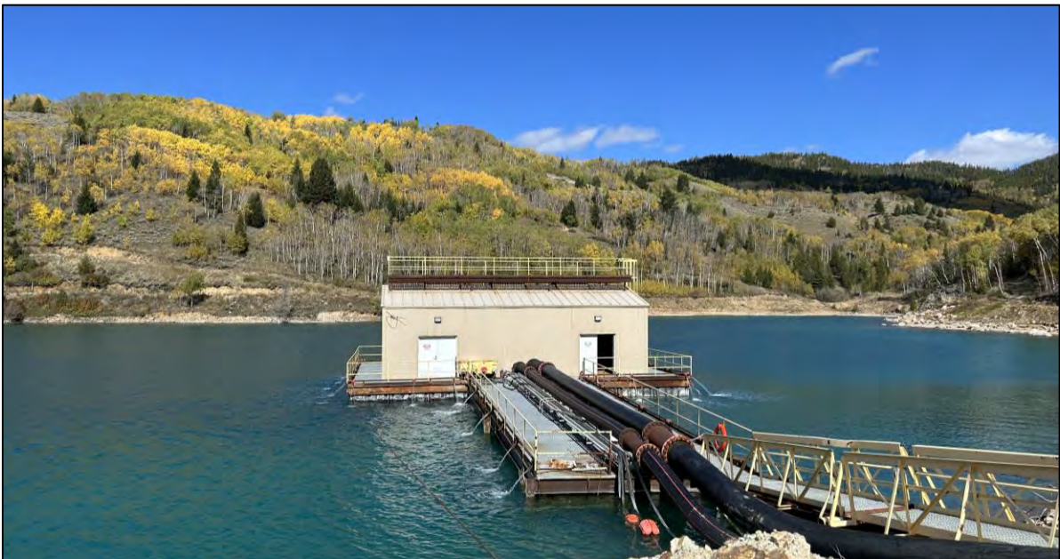
PHOTO 30 – Newer (northern) Reclaim Barge, facing north
