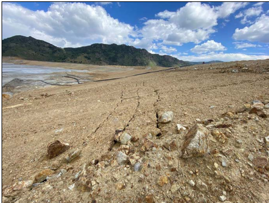
Photo 2.3 EL. 6,450 ft East-West Embankment Upstream Alluvium Facing Slope Cracking
