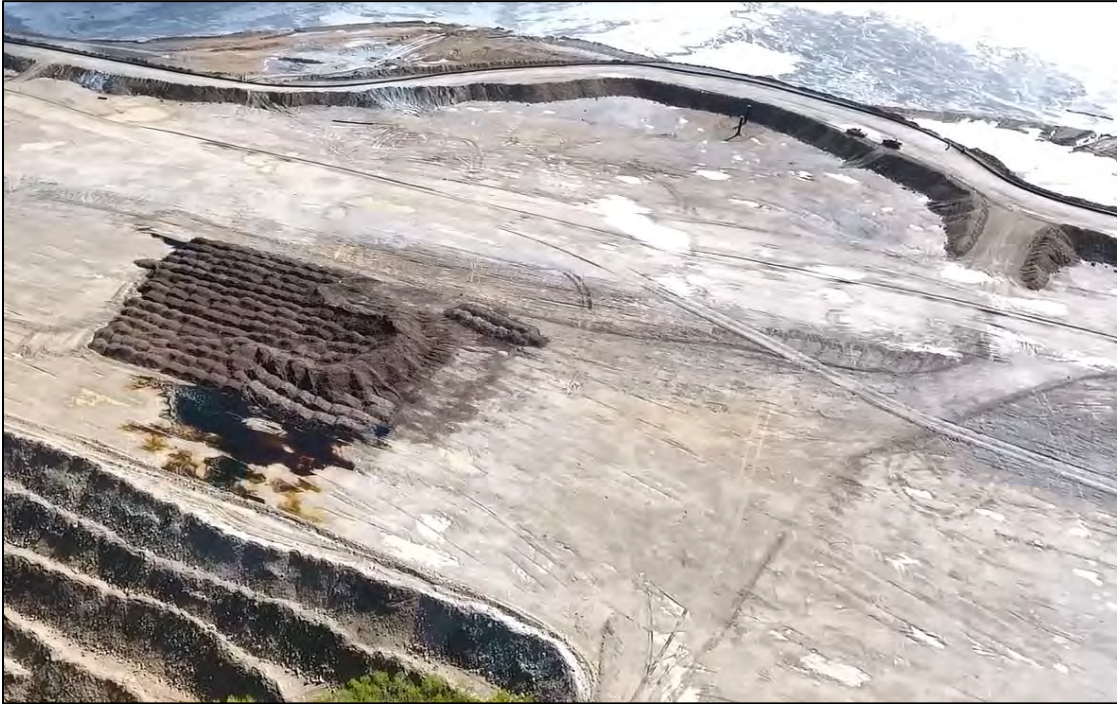
PHOTO 27 – West Embankment – organics stockpile on EL. 6,450 ft crest for use in downstream slope progressive reclamation.
