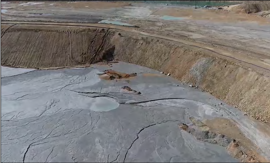
PHOTO 17 – East-West Embankment upstream face at discharge location EW-1, facing south.
