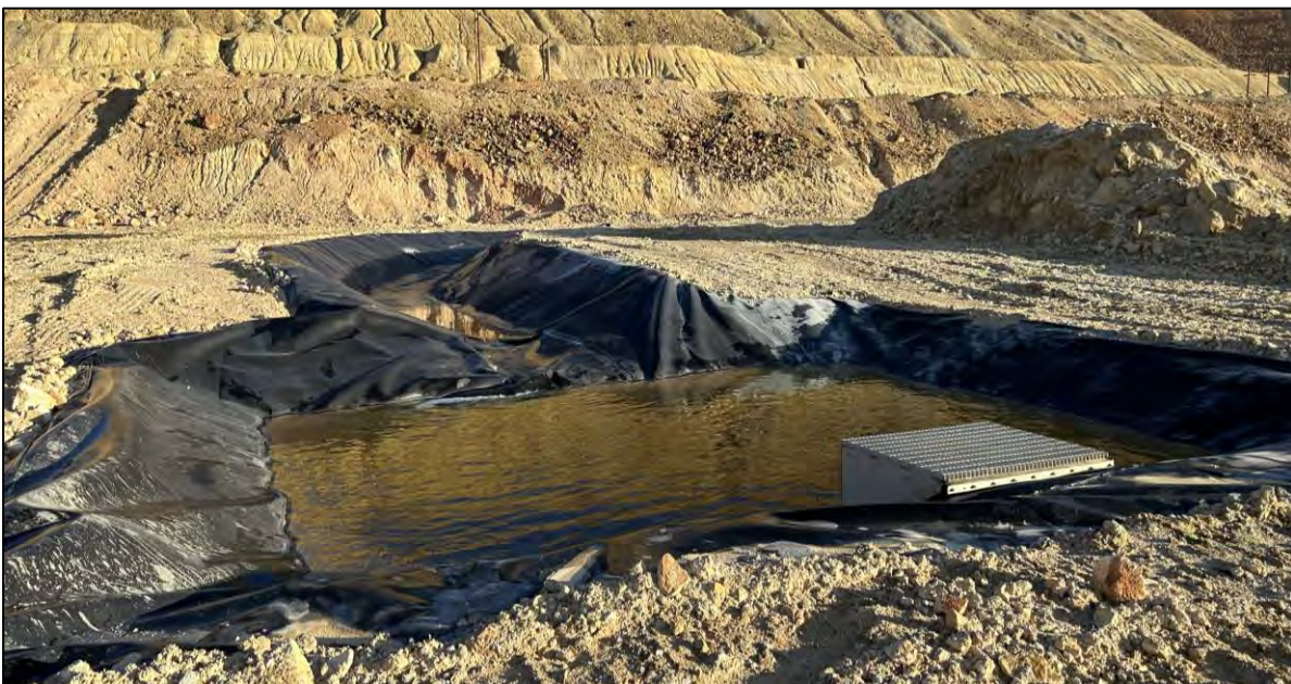
PHOTO 74 – Transition Pond on Seep 10 bench at end of SWD #10, facing north.
