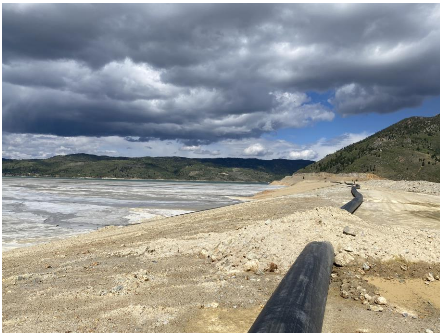
PHOTO 14 – North-South Embankment – Pipeline corridor – Tailings Pipeline 3
