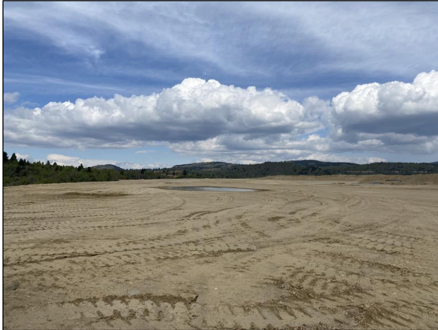
PHOTO 1 – West Embankment – Crest of Dam well graded with minimal depressions
