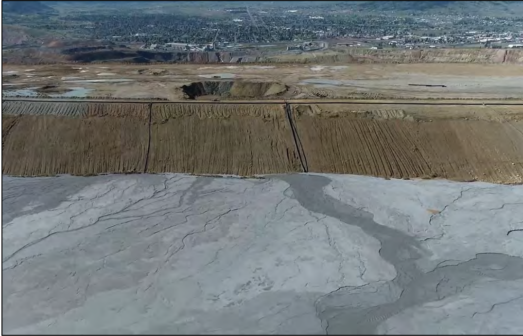
PHOTO 9 – East-West Embankment upstream regrading and alluvium facing completed in Central Pedestal Area, facing south.
