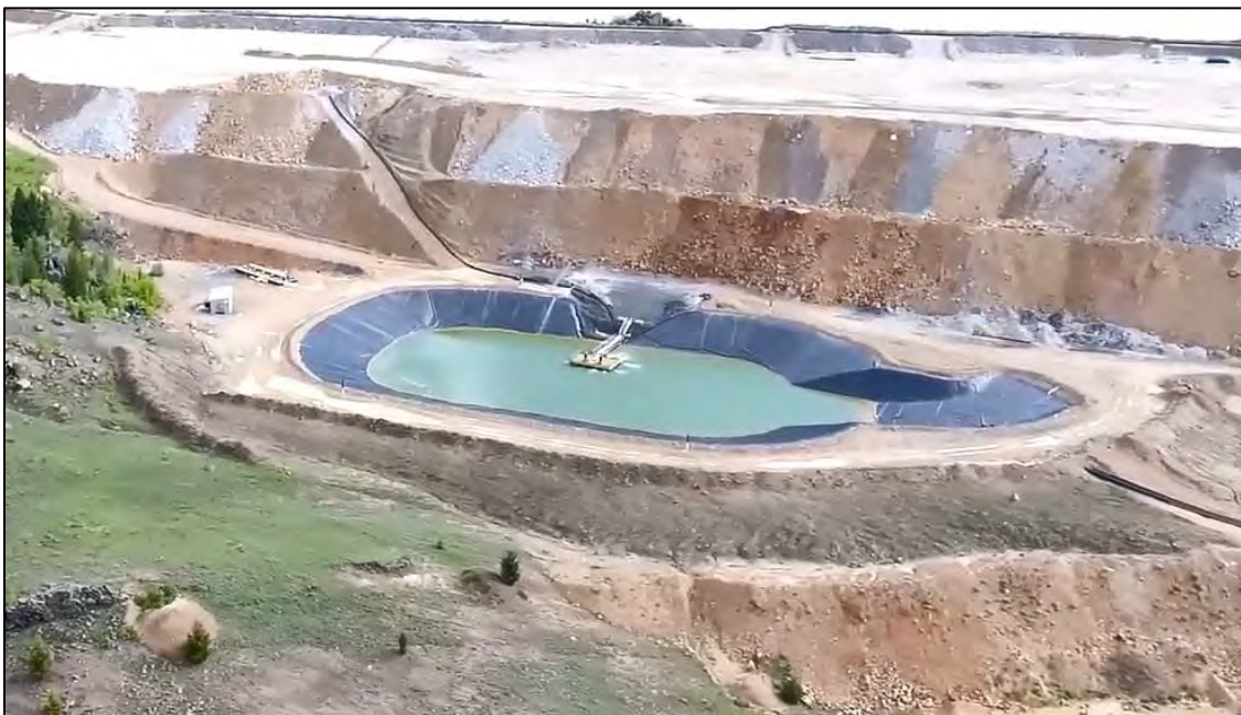
PHOTO 28 – Overview of WED Extraction Pond.
