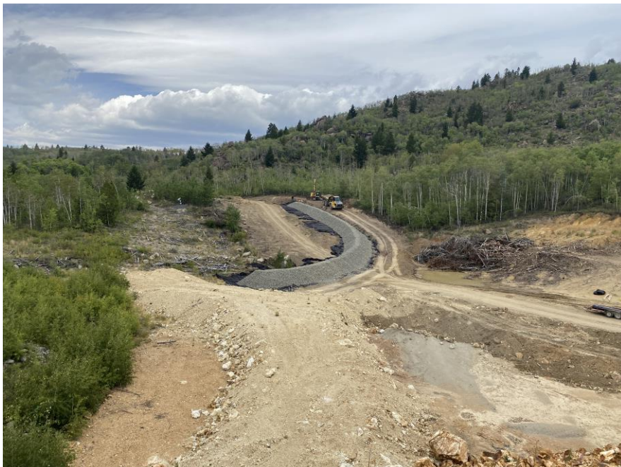
PHOTO 4 – West Embankment – Drain located at the north abutment
