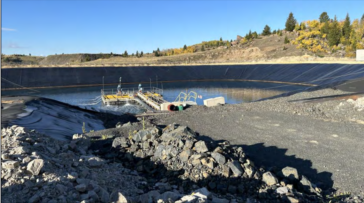
PHOTO 45 – WED Extraction Pond, facing west.
