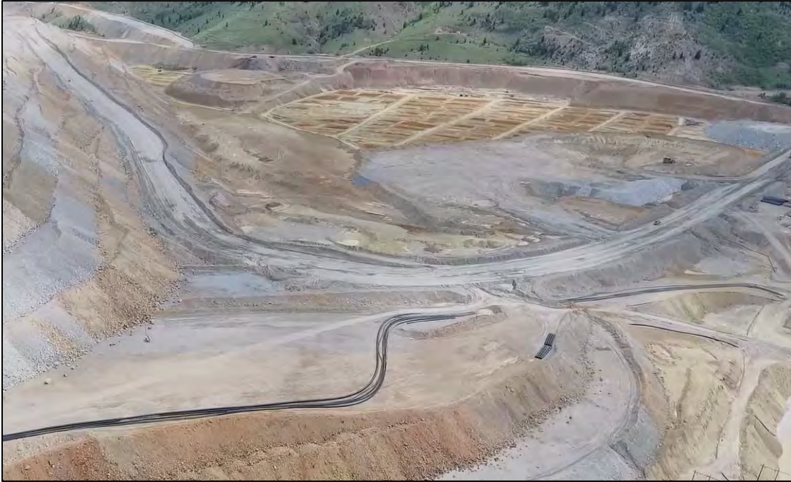
PHOTO 3 – North RDS construction with initial haul ramp lifts, facing northeast
