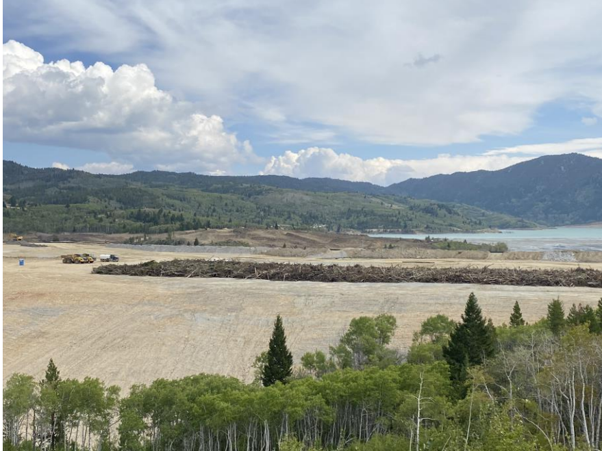
PHOTO 3 – West Embankment – EL. 6,450 ft lift crest – Organics stockpile
