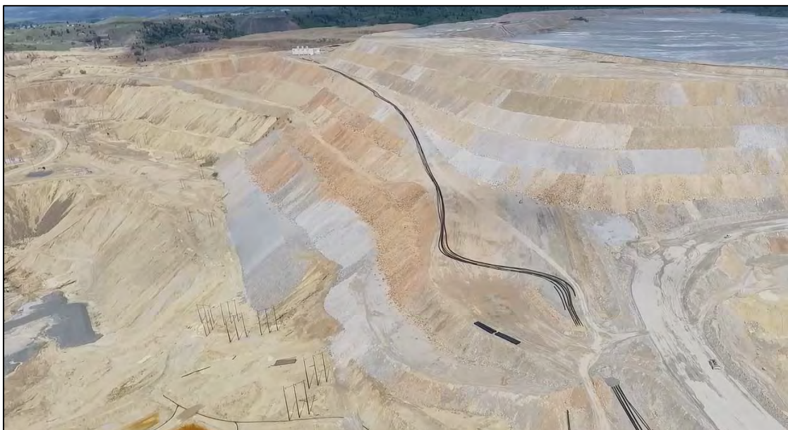
PHOTO 2 – Central Pedestal Area downstream shell, facing west.
