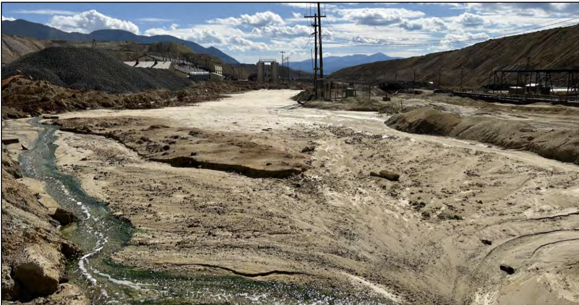
PHOTO 62 – Zone 2B stockpile (left) and dewatered Houligan Pond (center), facing south
