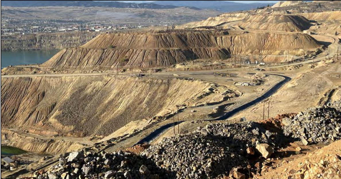
PHOTO 73 – Overview of Seep 10 bench surface water ditch (SWD #10), facing southwest.
