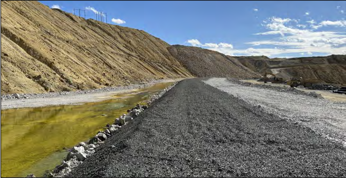
PHOTO 57 – Rock drain D6 construction progress in the HsB Area, facing south.
