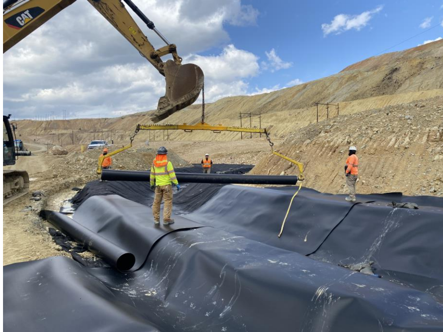
PHOTO 29 – Seep 10 – SWD#10 geomembrane install by Northwest Linings
