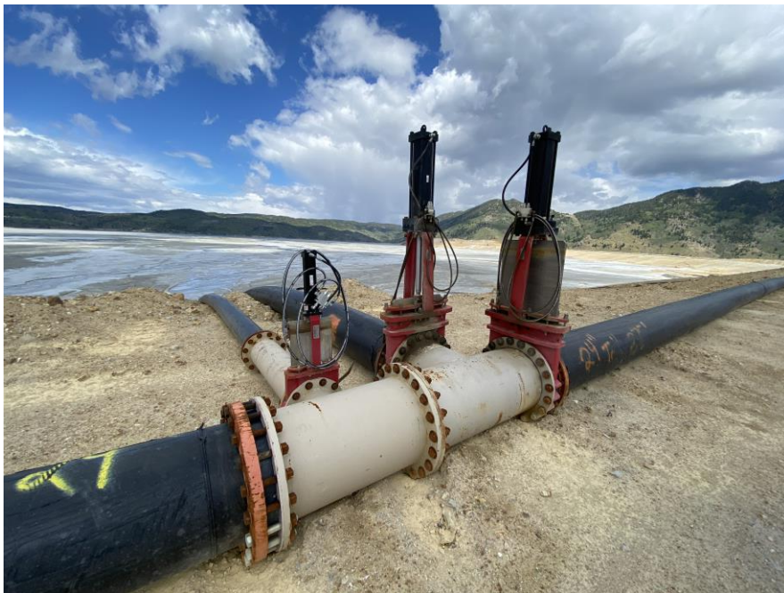
PHOTO 10 – East-West Embankment – Spigot 3-2 and 3-2A
