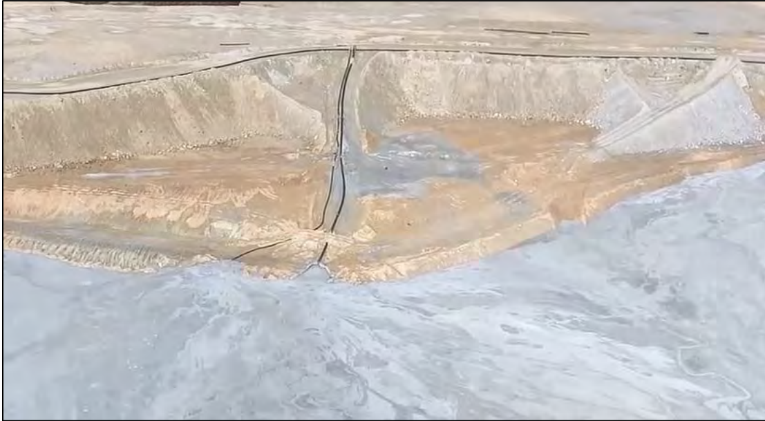
PHOTO 23 – West Embankment upstream interface and discharge location RK-3, facing west.
