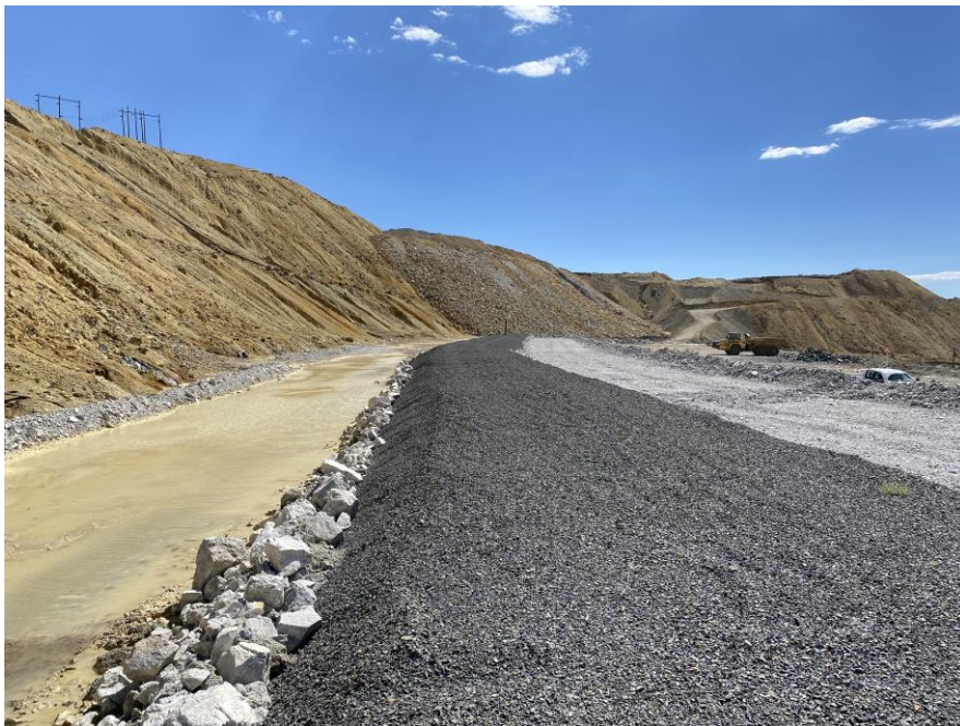
PHOTO 26 – Stage 1 HsB RDS – D6 STA 0+600 ft looking south
