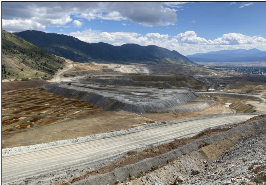
Photo 2.4 EL. 6,150 ft North RDS and Future Haul Ramp Construction
