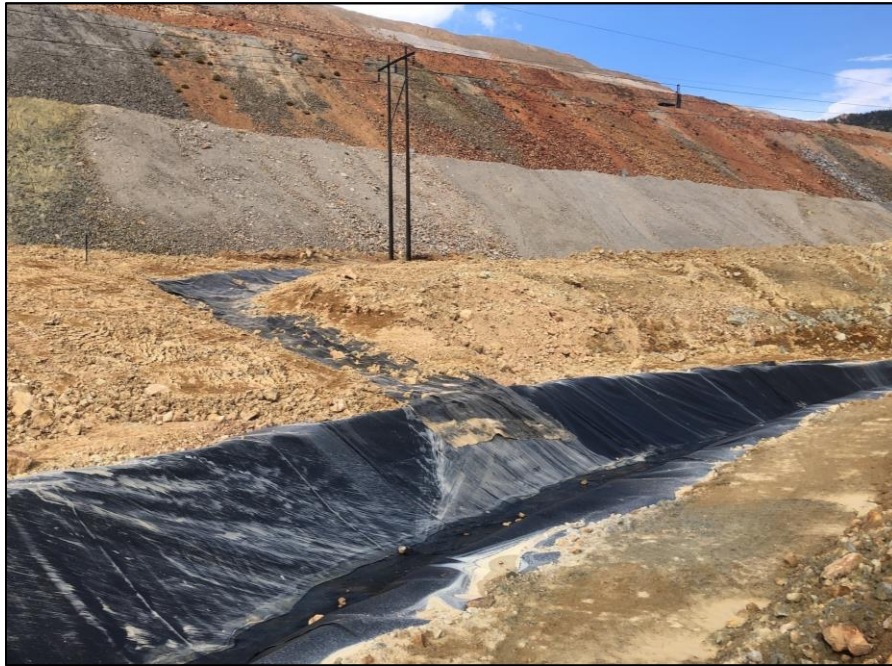
Photo 2.8 Geotextile Added North of SWD#10 to Prevent Sediment Erosion into Ditch
