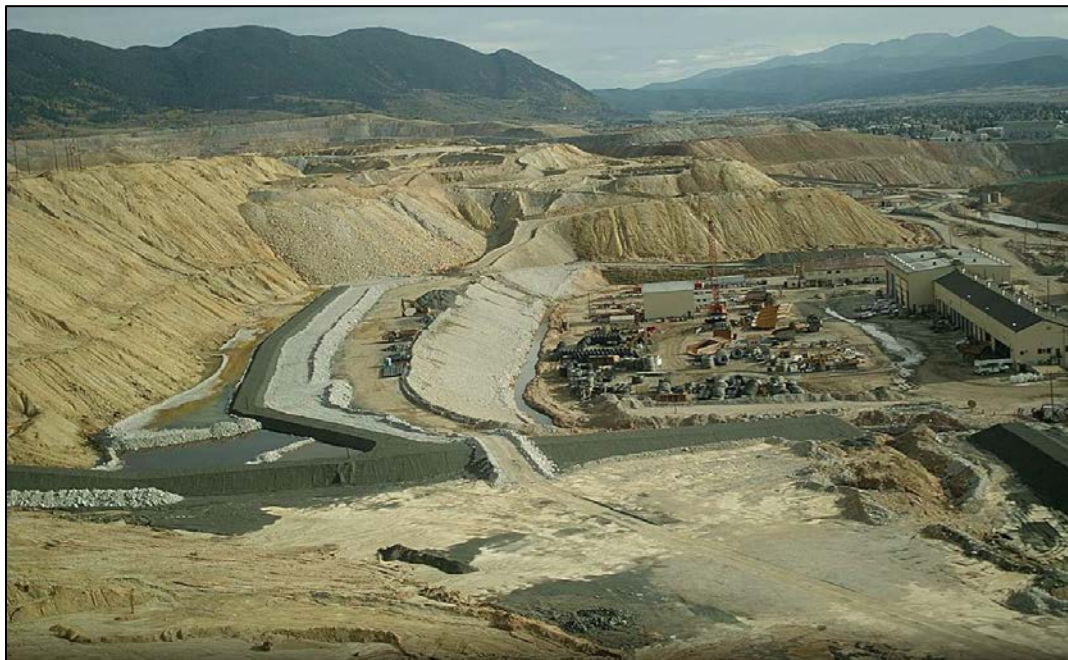
Photo 2.5 Zone UF Placement along Drain D6
