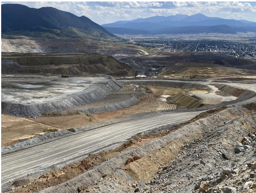
PHOTO 16 – North RDS – Ripping of existing ground for future expansion of RDS
