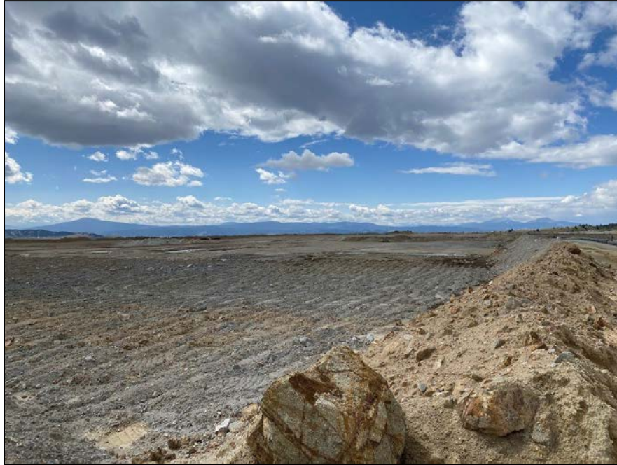
Photo 2.2 EL. 6,450 ft East-West Embankment Ripping for Fill Placement and Regrading
