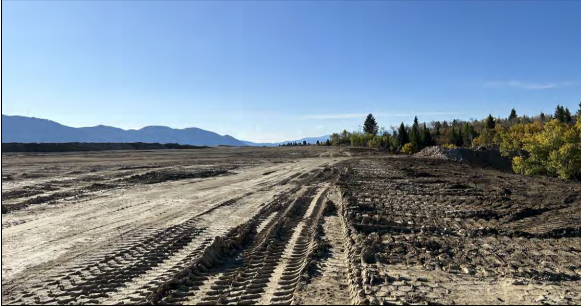
PHOTO 49 –West Embankment EL. 6,450 ft lift crest near Section 95+00W, facing south.
