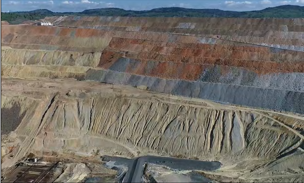
PHOTO 11 – East-West Embankment downstream slope and Number 10 Seep bench area, facing north.
