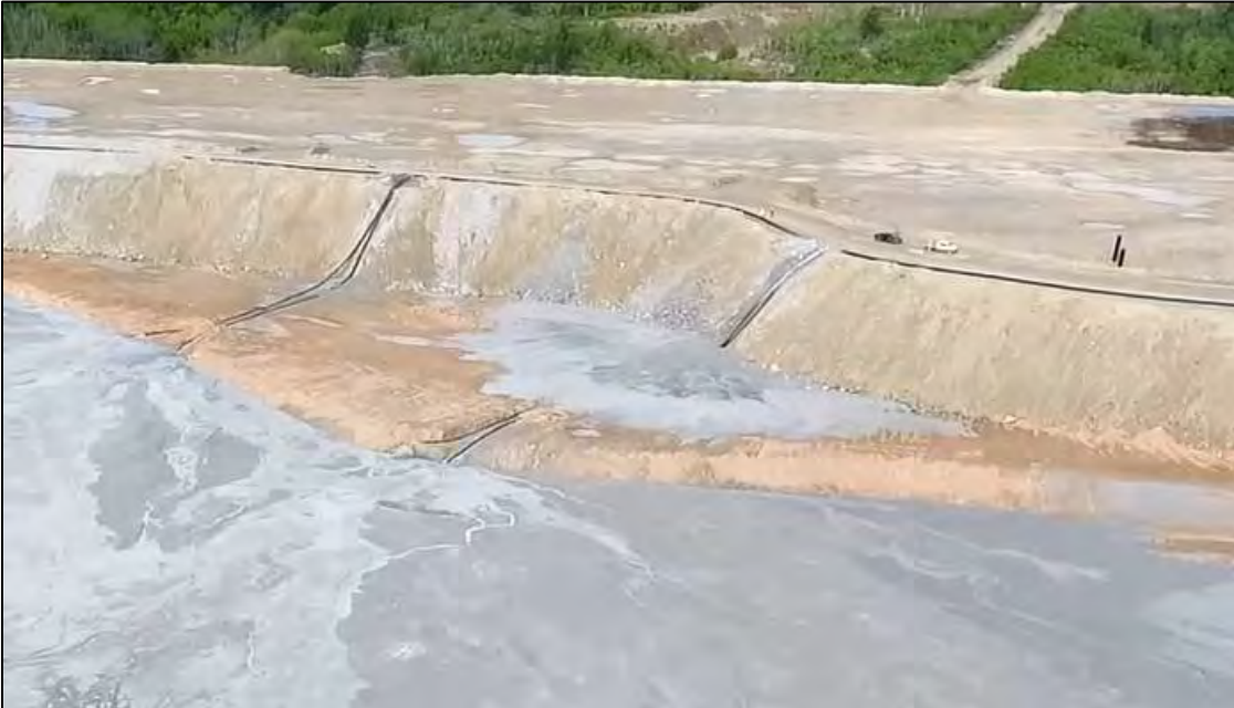
PHOTO 22 – West Embankment upstream interface with view of 12-inch discharges between discharge locations RK-2 and RK-3, facing west.
