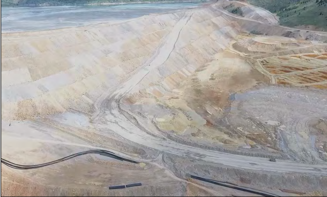
PHOTO 1 – North-South Embankment downstream shell, facing north from southeast end of YDTI.
