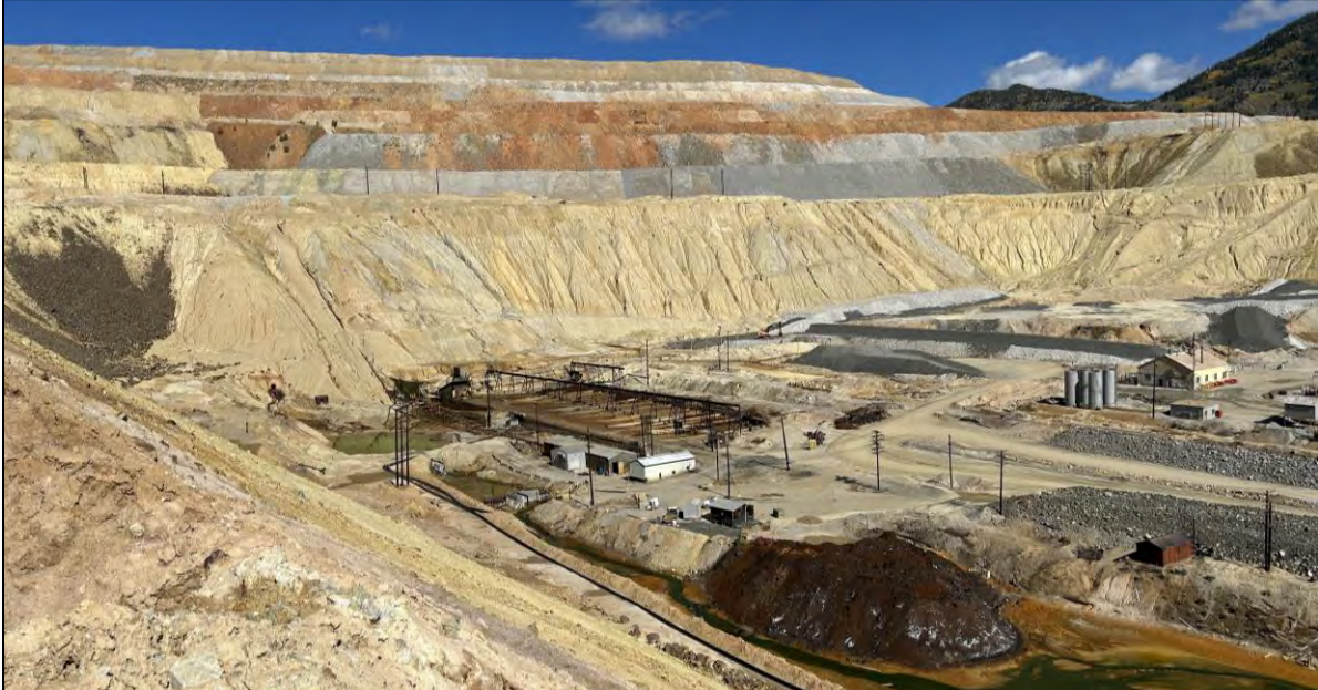
PHOTO 65 – HsB area drainage system construction progress, facing northeast from 7% ramp.
