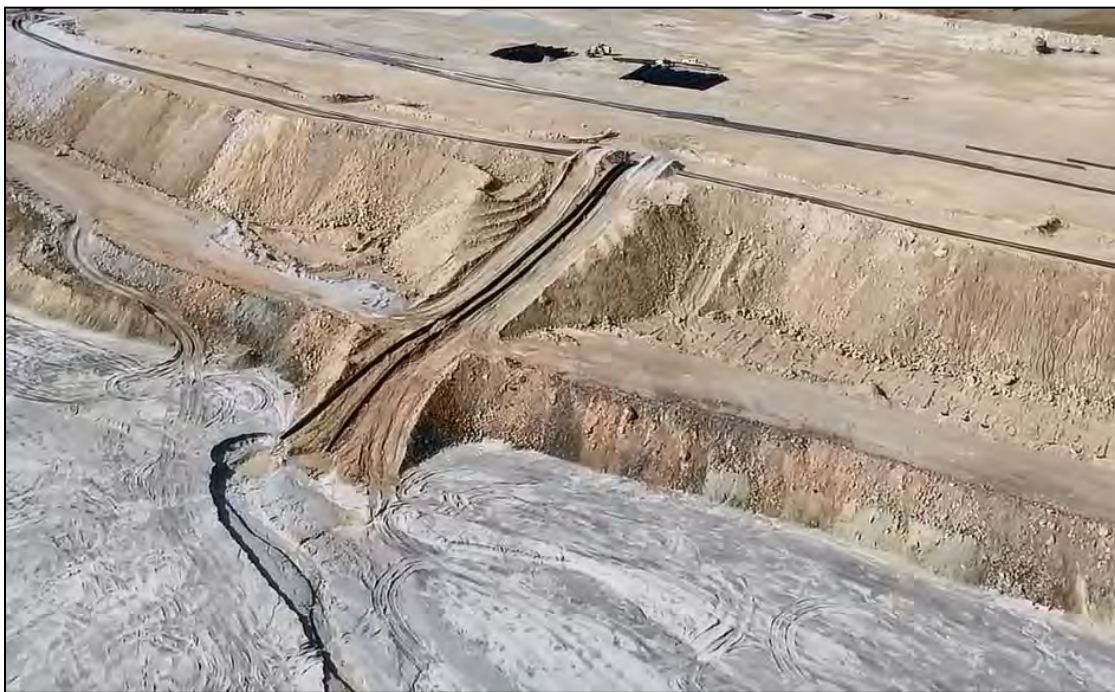
PHOTO 20 – East-West Embankment upstream side at discharge location EW-2, facing southwest.
