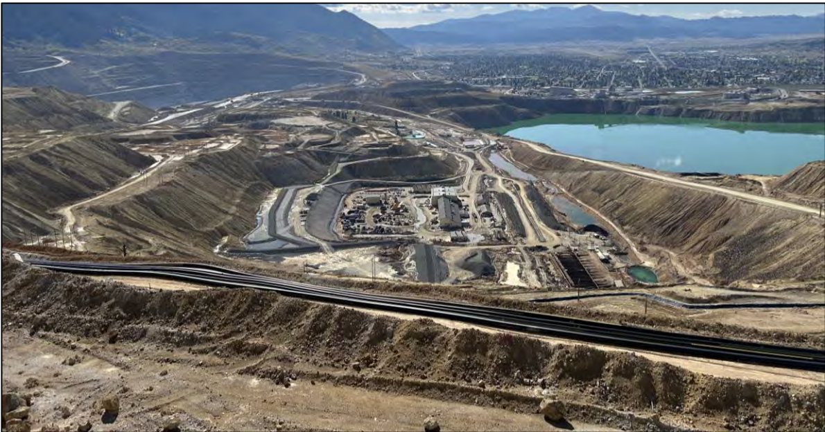
PHOTO 54 – Horseshoe Bend overview from East-West Embankment EL. 6,450 ft crest, facing south.
