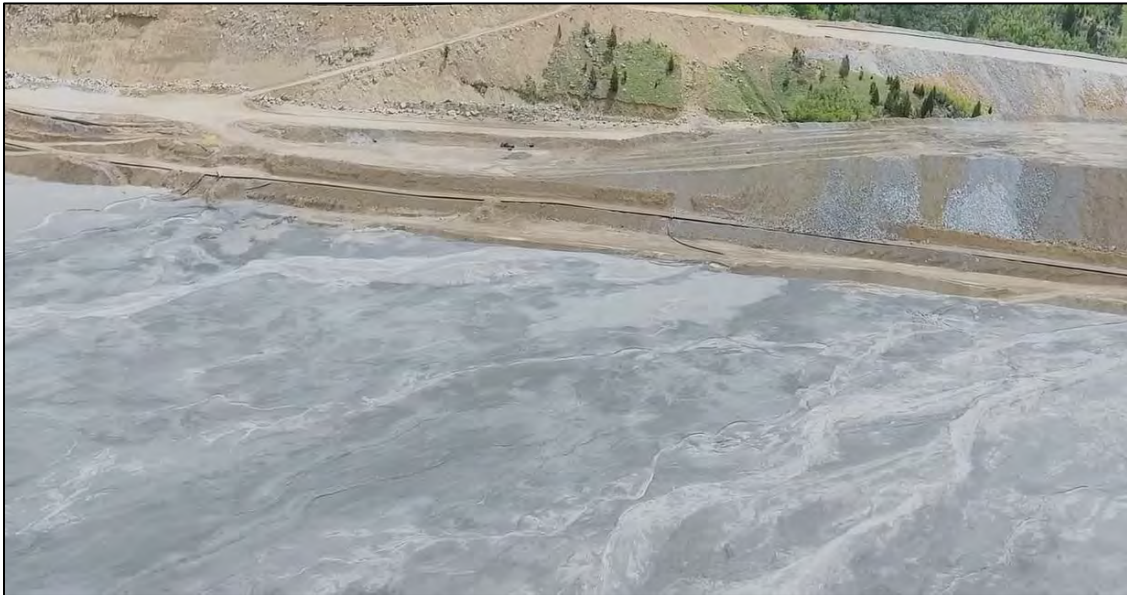
PHOTO 6 – North-South Embankment deferred fill placement area beyond approximately Section 50+00N, facing east.
