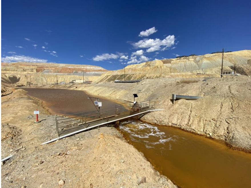
PHOTO 23 – HsB Weir – Looking North
