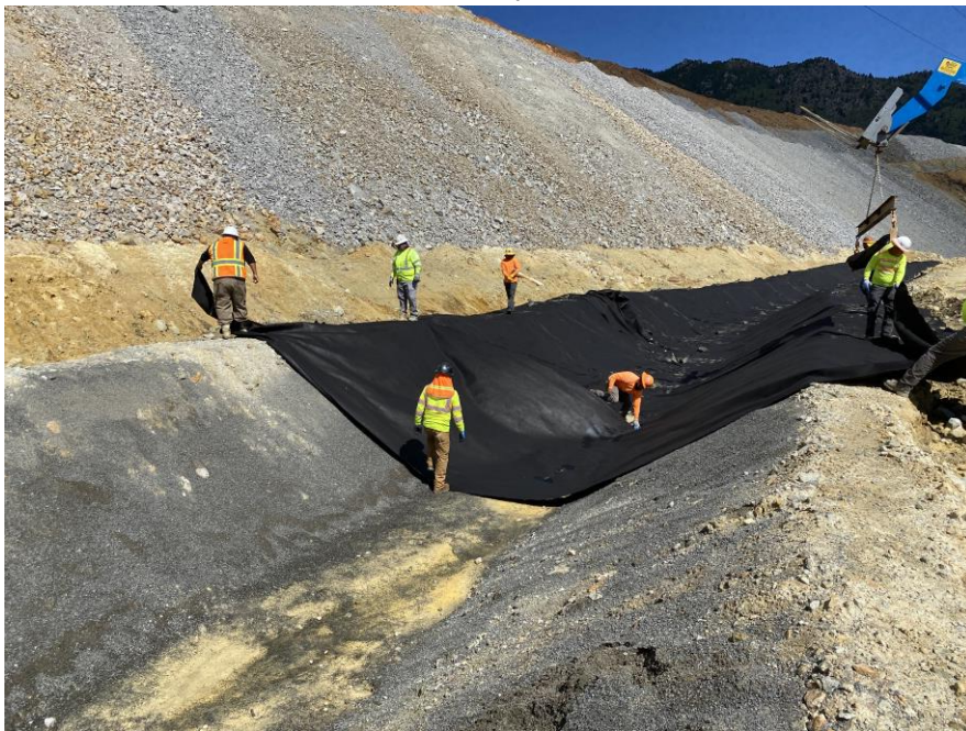
PHOTO 28 – Seep 10 – SWD#10 geotextile install by Northwest Linings
