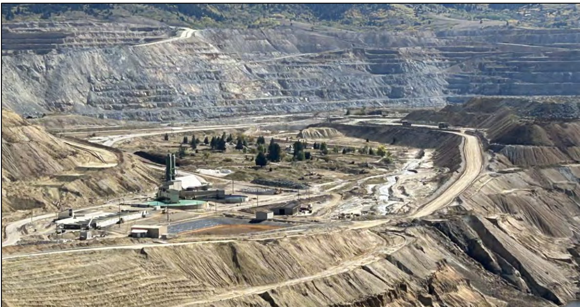
PHOTO 80 – Scalper Road On-site Containment Project visible with Continental Pit in background, facing southeast.
