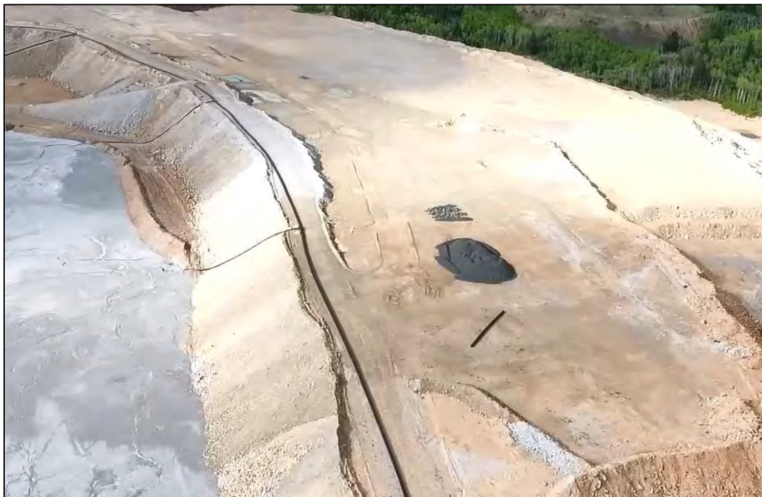
PHOTO 24 – West Embankment with view of upstream interface and EL. 6,450 ft crest, facing south near discharge location RK-4.
