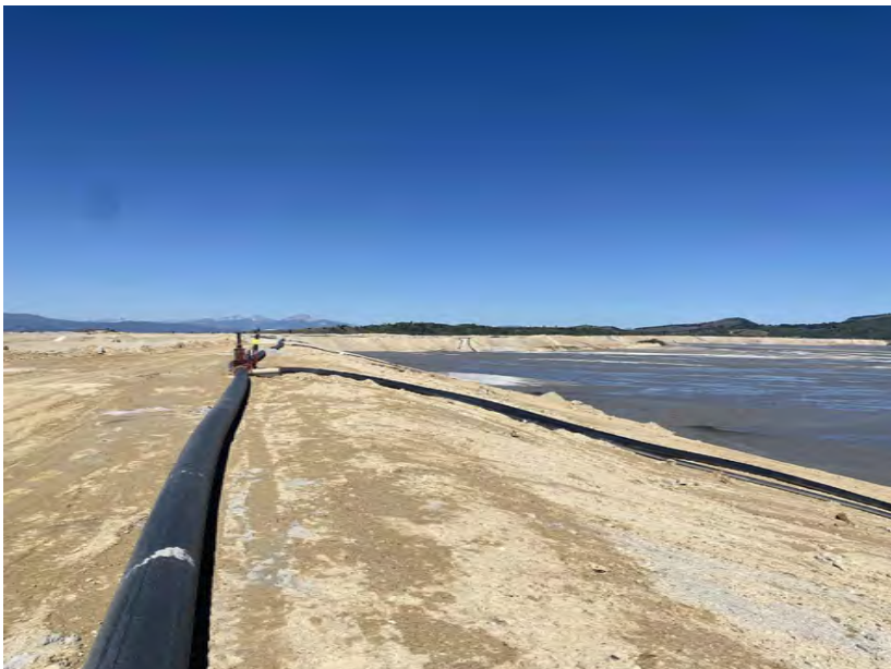
EAST-WEST EMBANKMENT (JULY 2023)
