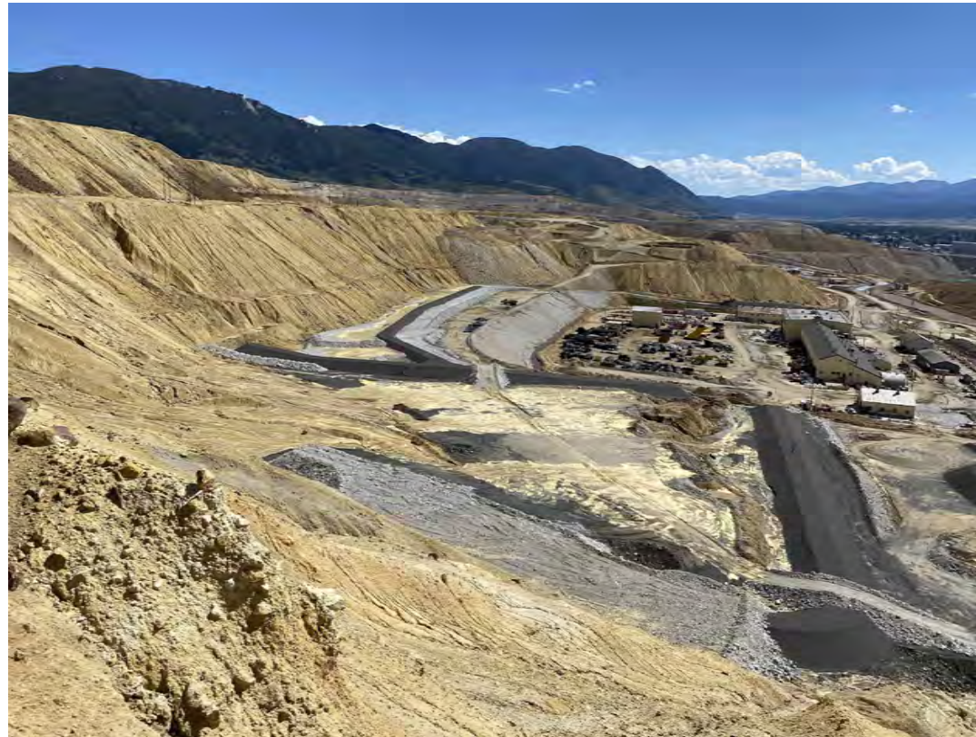
STAGE 1 HsB RDS DRAINAGE SYSTEM - EAST SIDE (UNDER CONSTRUCTION)
