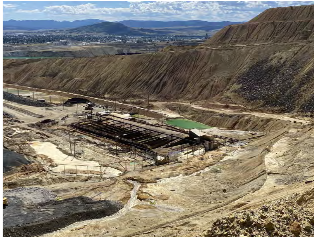
STAGE 1 HsB RDS DRAINAGE SYSTEM - WEST SIDE (UNDER CONSTRUCTION)
