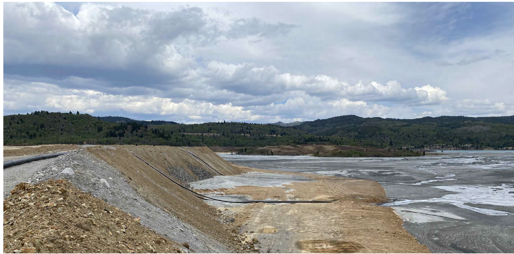
TAILINGS DISCHARGE WEST EMBANKMENT
