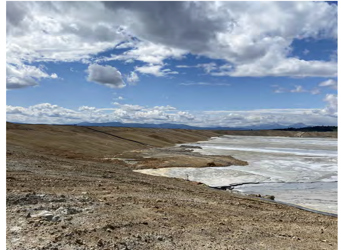
TAILINGS DISCHARGE EAST-WEST EMBANKMENT
