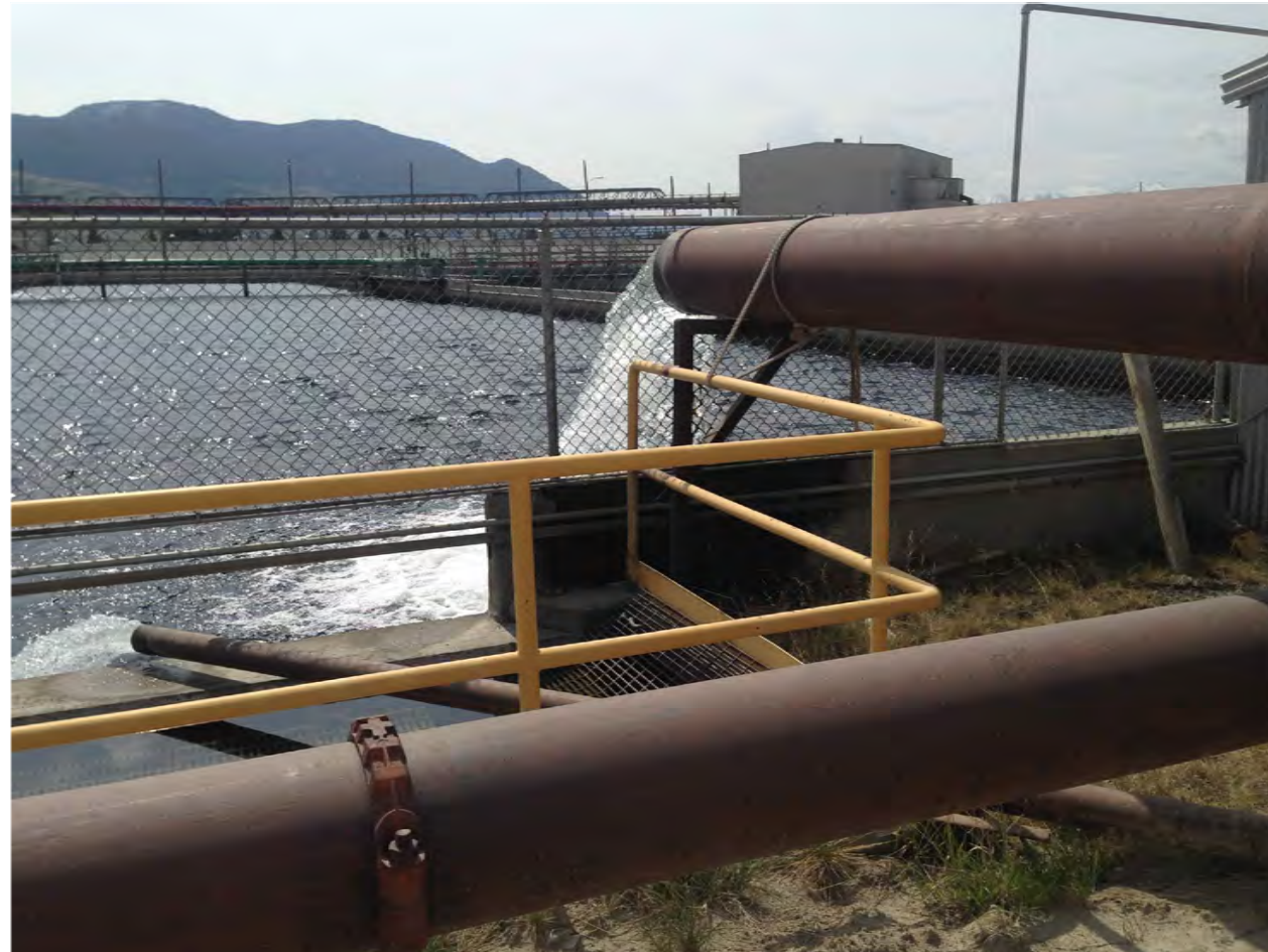
RECLAIM DISCHARGE INTO MILL RESERVOIRS
