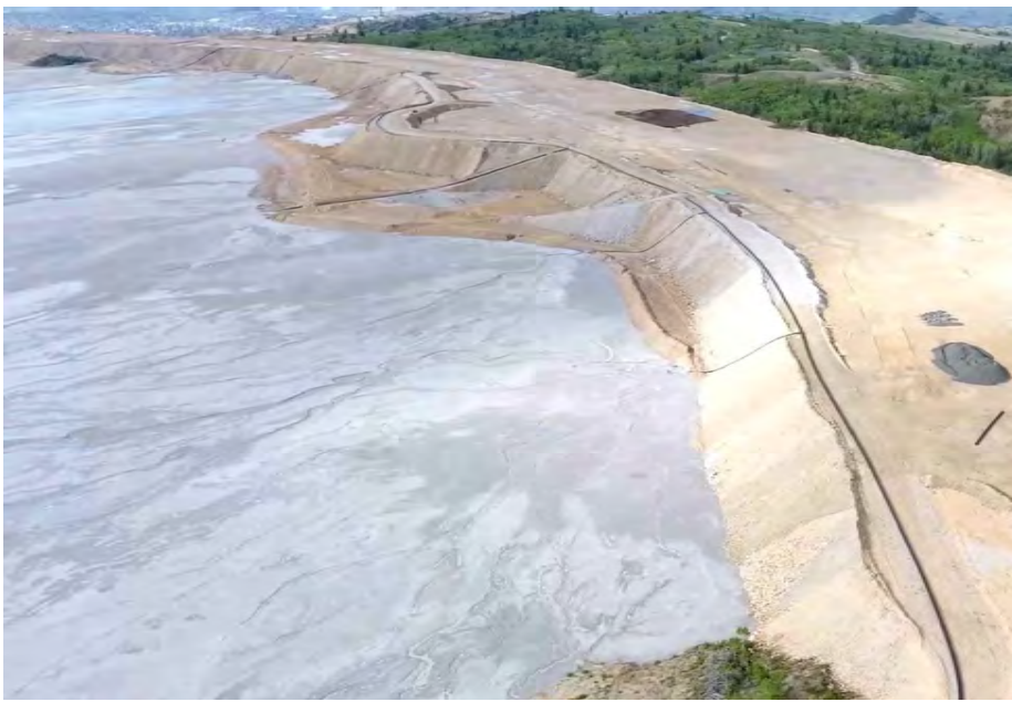
WEST EMBANKMENT (JULY 2023)
