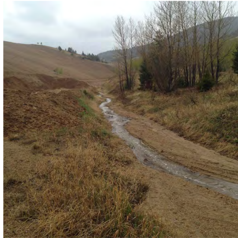
CLEAR WATER DITCH
