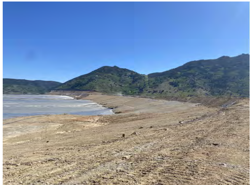
NORTH-SOUTH EMBANKMENT (JULY 2023)
