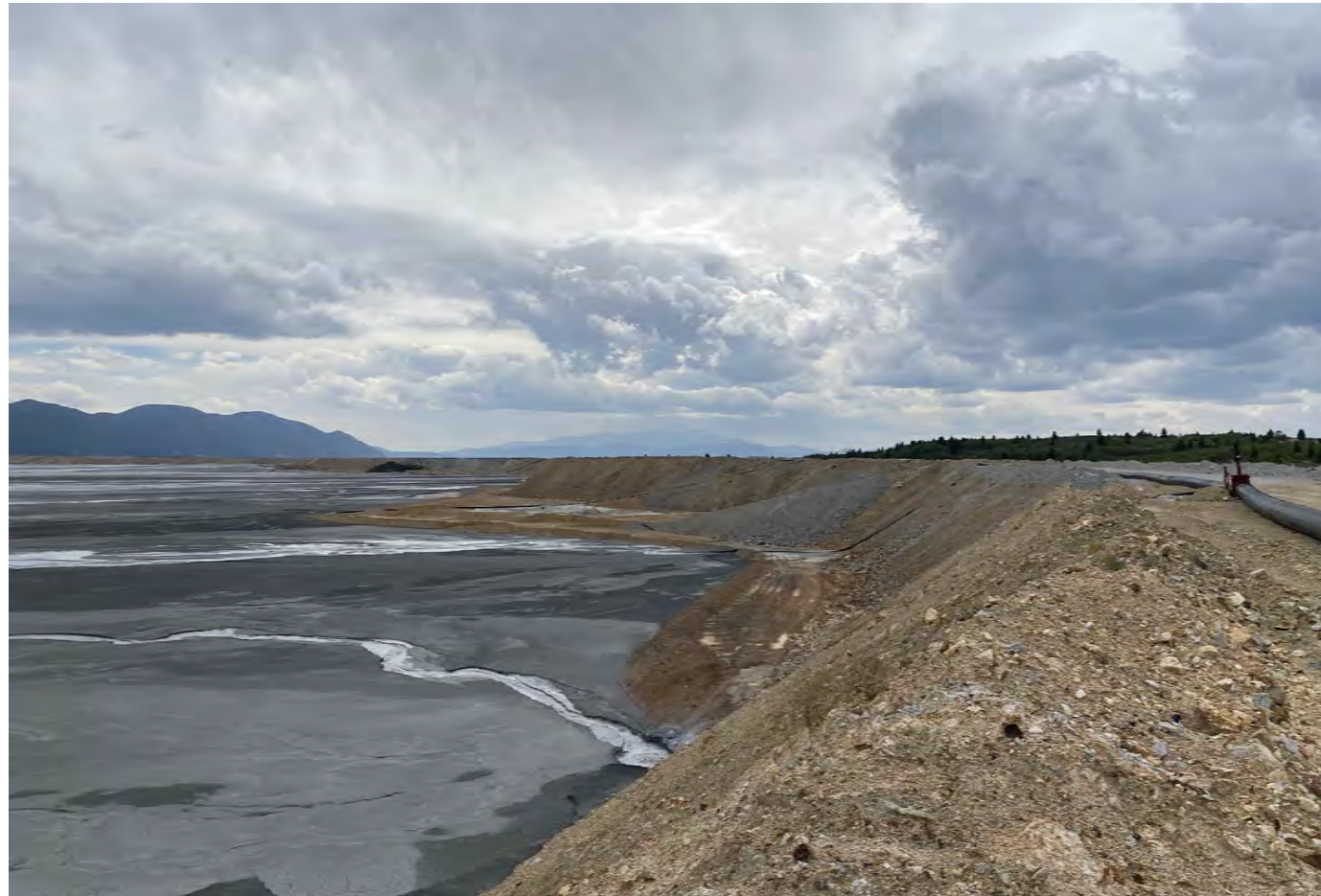
UPSTREAM EMBANKMENT SLOPE WEST EMBANKMENT
