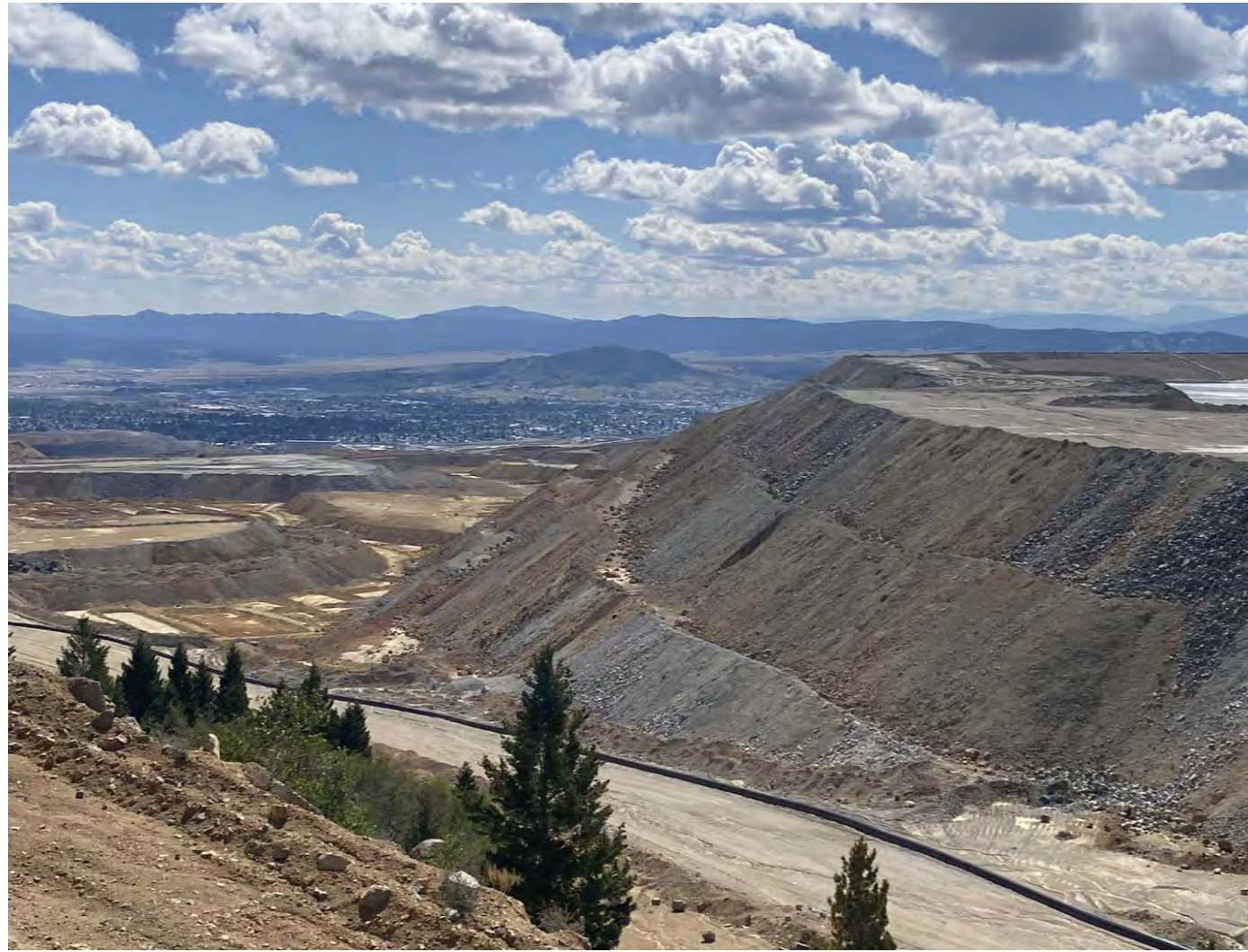
DOWNSTREAM EMBANKMENT SLOPE NORTH-SOUTH EMBANKMENT
