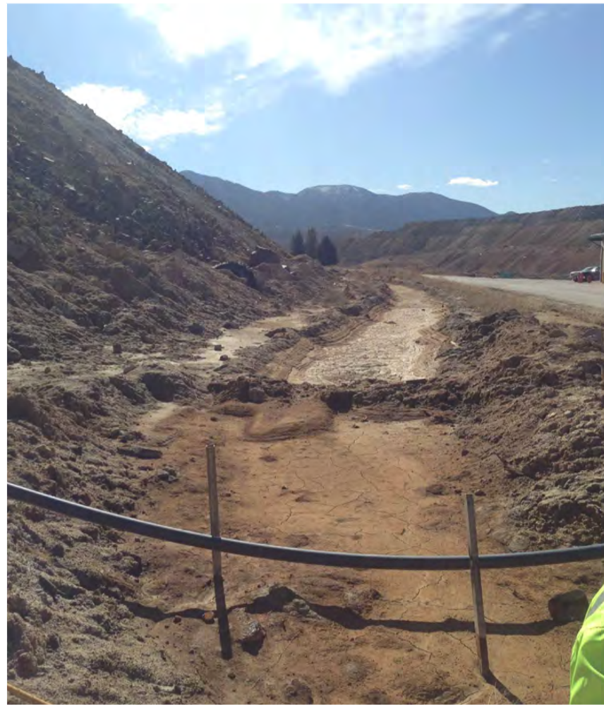
TYPICAL DRAINAGE DITCH
