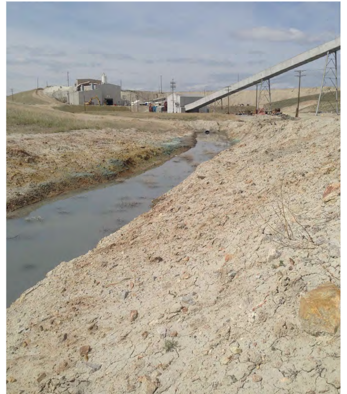
SITE DRAINAGE DITCH
