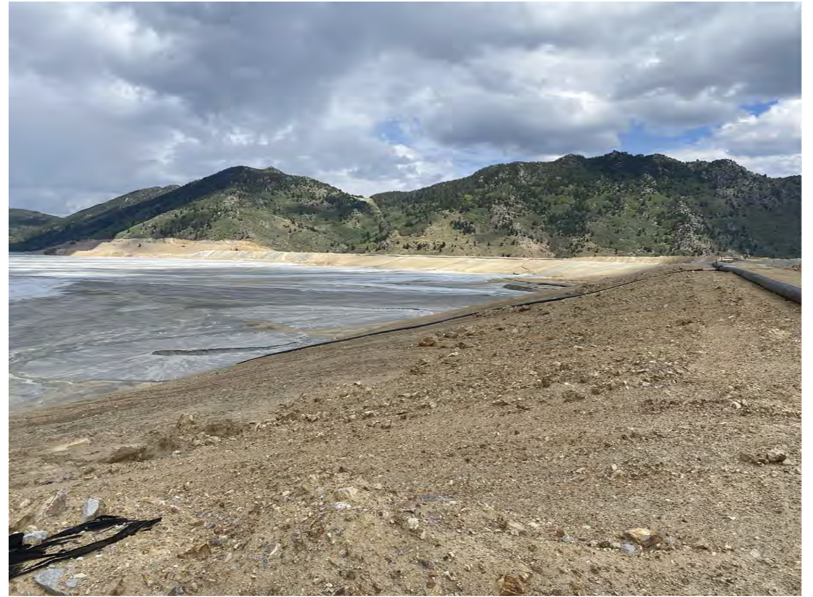
UPSTREAM EMBANKMENT SLOPE EAST-WEST AND NORTH SOUTH EMBANKMENT
