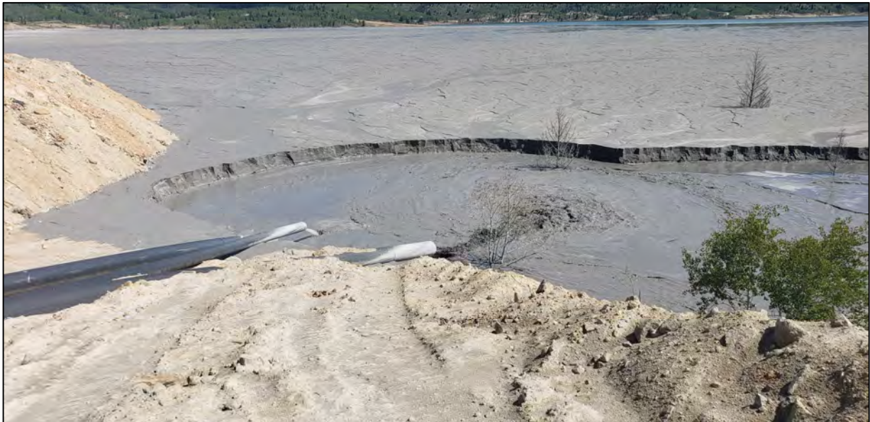
PHOTO 12 – West Embankment – RK-1 tailings discharge location. (June 26, 2020)
