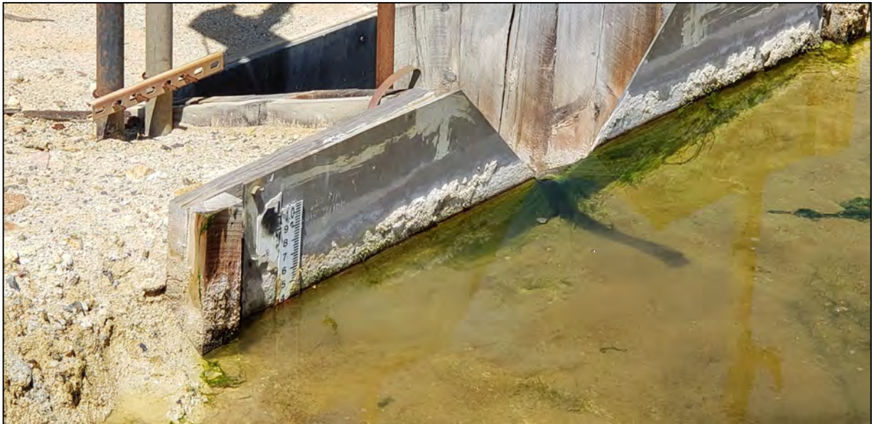
PHOTO 16 – Seep 10 Weir Staff Gauge reading approximately 0.4. (June 26, 2020)
