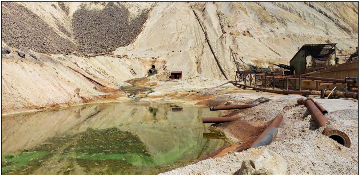
PHOTO 20 – HsB Area – Upper Pond and HsB seeps. (June 26, 2020)
