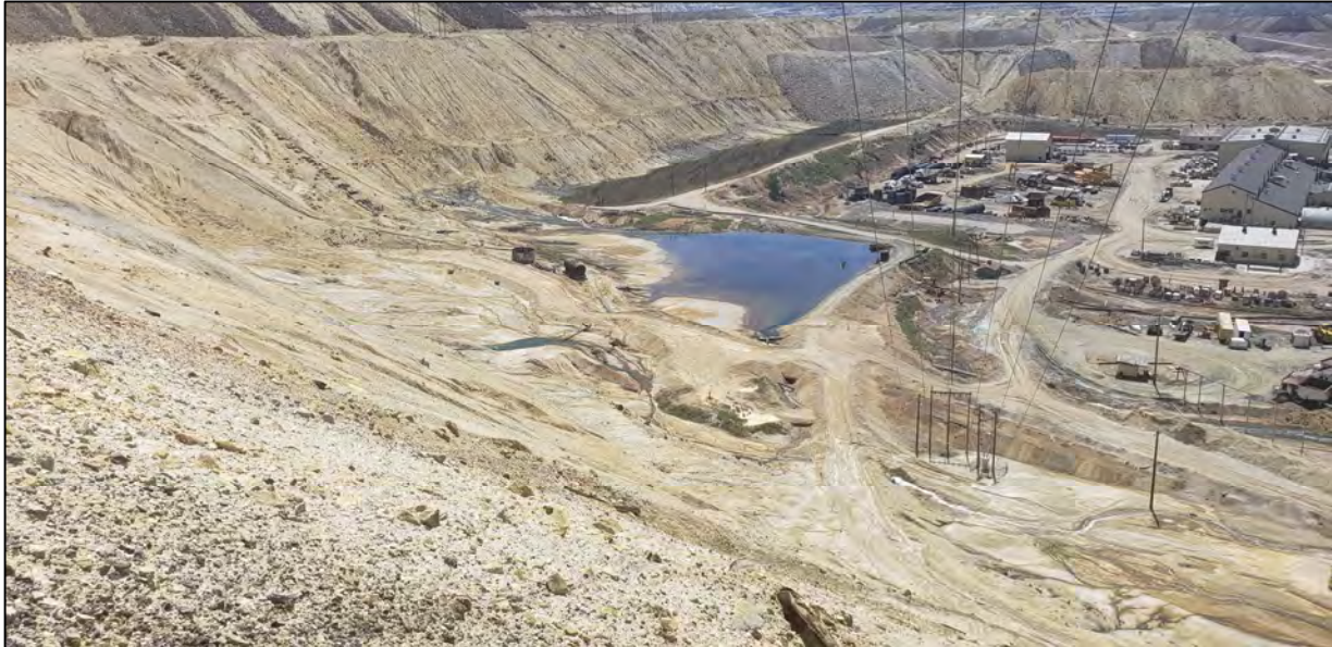
PHOTO 17 – Horseshoe Bend (HsB) Area – Leach seeps along toe of East-West Embankment viewed from Seep 10 bench. (June 26, 2020)
