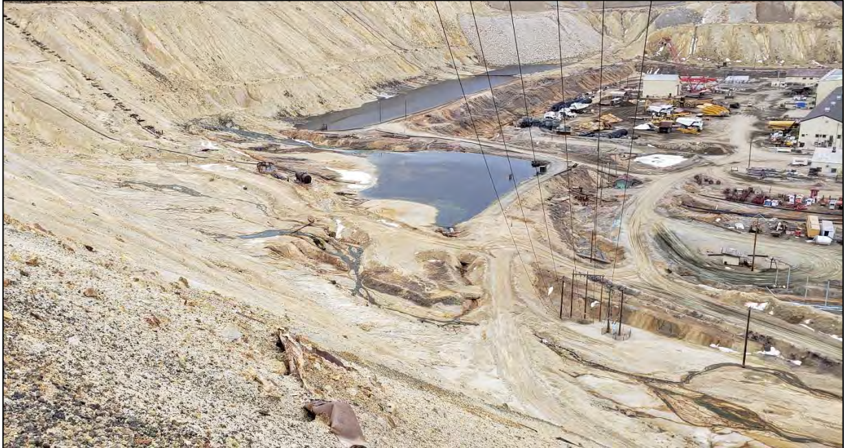
PHOTO 17 – Horseshoe Bend (HsB) Area – Leach seeps along toe of East-West Embankment viewed from Seep 10 bench. (March 31, 2020)
