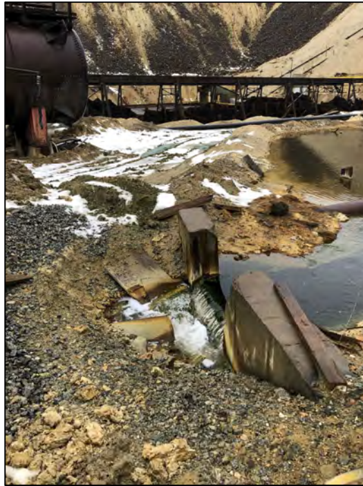
Photo 7.1 Bypass Flow at Hooligan Pond Weir
