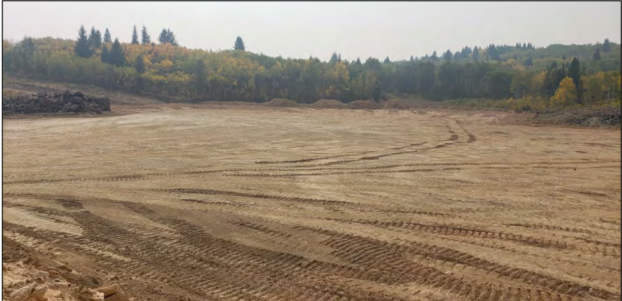
PHOTO 11 – West Embankment – EL 6,400 ft Zone D1 Material near Temporary Extraction Pond location
