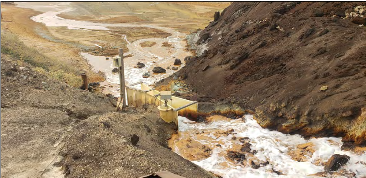
PHOTO 26 – HsB Area – Cell 10 Return Water Flume
