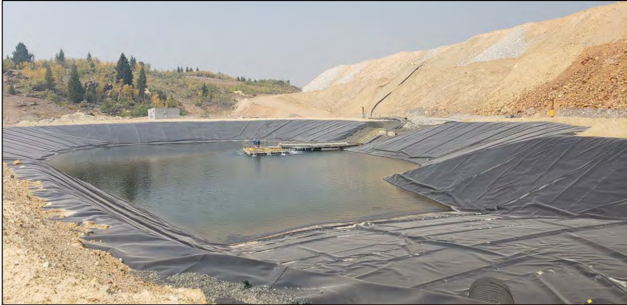
PHOTO 13 – Sep 16, 2020 – WED Extraction Pond and Dewatering System.
