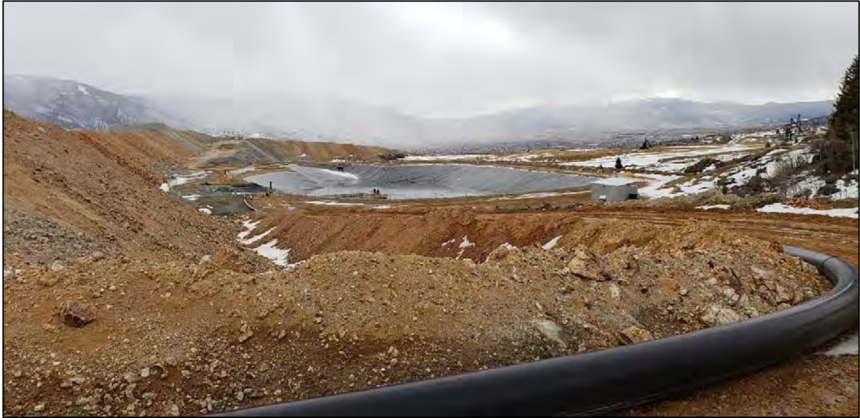
PHOTO 11 – West Embankment – WED Extraction Pond and Pump Station. (March 30, 2020)
