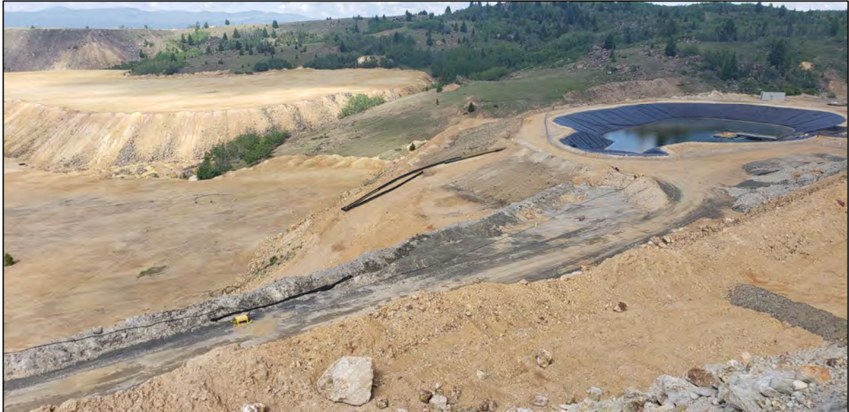
PHOTO 11 – West Embankment – WED Extraction Pond and emergency overflow pipelines. (June 26, 2020)
