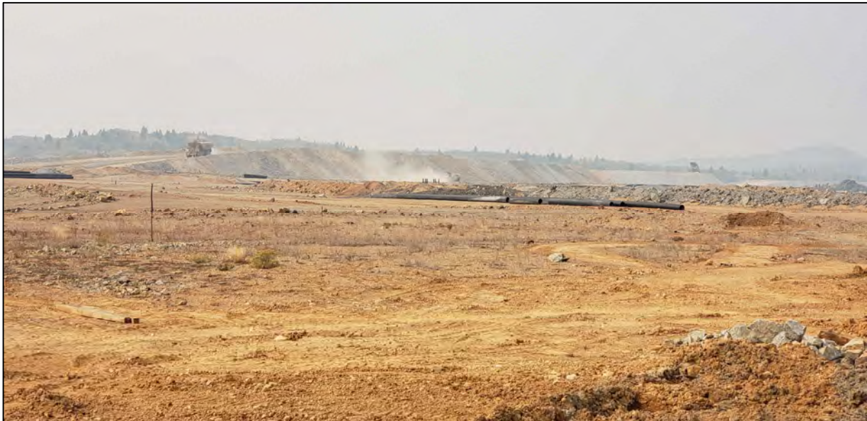
PHOTO 6 – East-West Embankment – EL 6,450 ft construction progress
