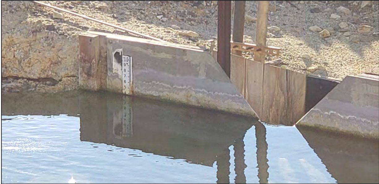
PHOTO 3 – Dec 10, 2020 – Seep 10 Weir and Staff Gauge. Staff Gauge reading slightly below 0.4.
