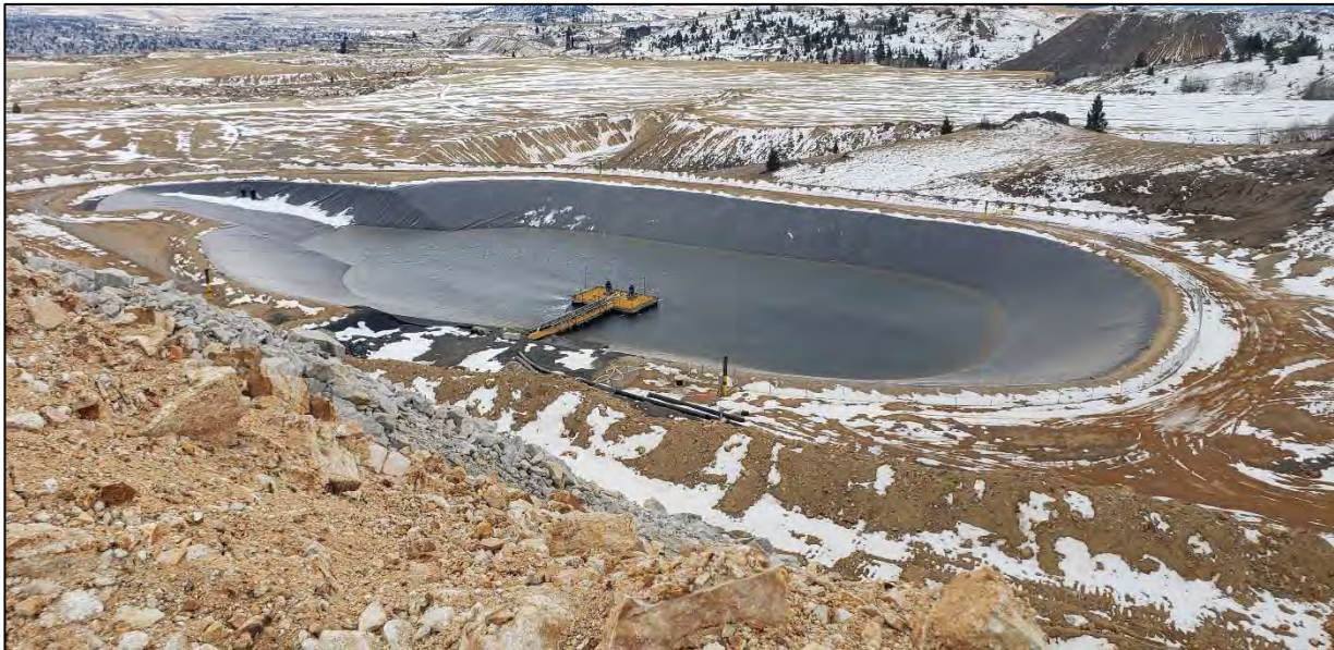
PHOTO 10 – West Embankment – Extraction Pond
