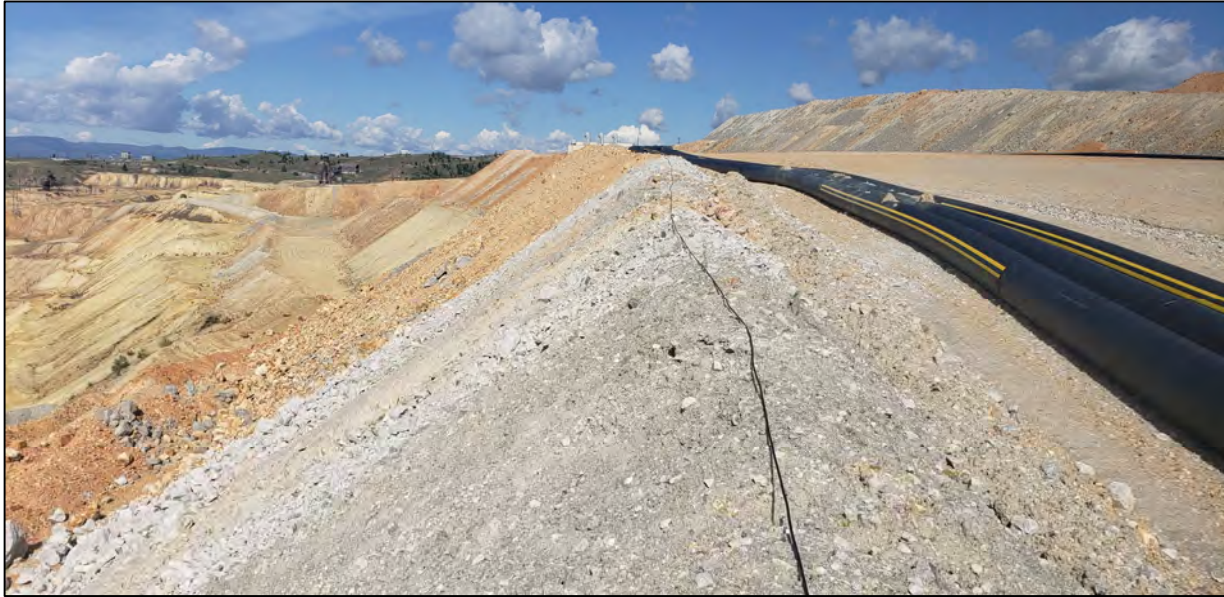
PHOTO 5 – East-West Embankment – Downstream edge of the pipe ramp. (June 26, 2020)
