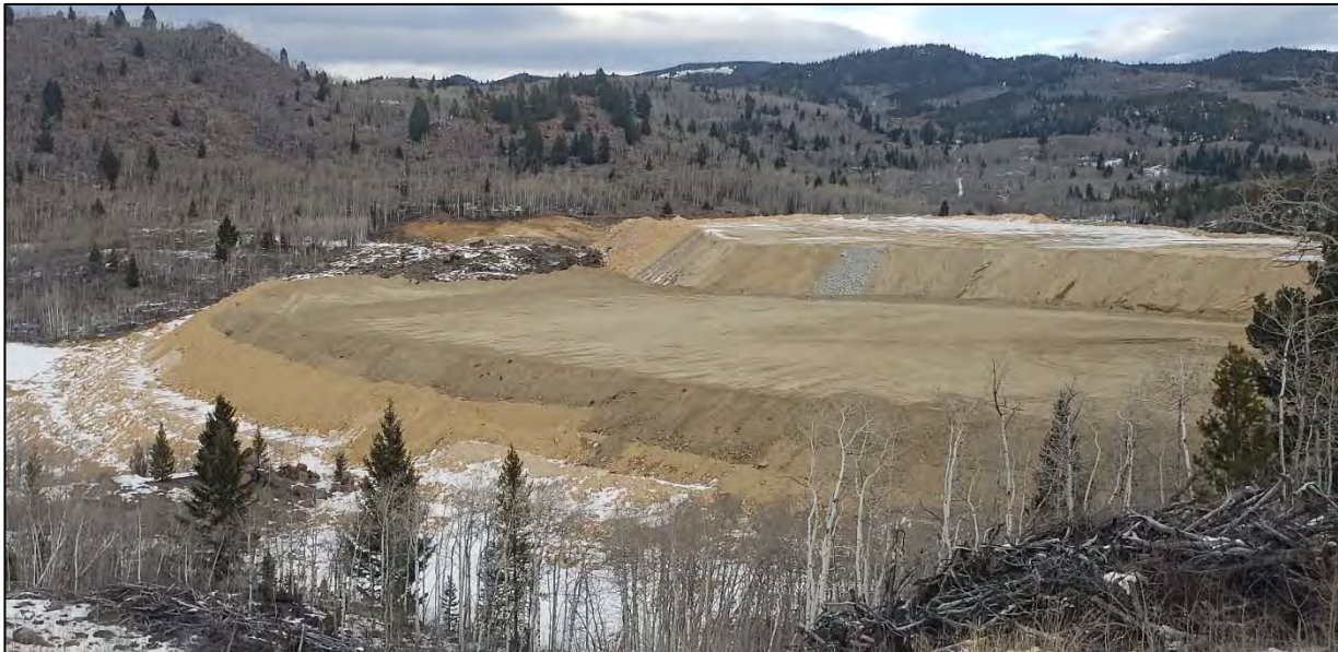
PHOTO 8 – West Embankment – Zone D1 construction at Drain Pod 1 location
