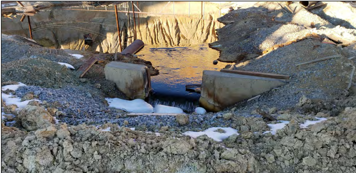
PHOTO 6 – Dec 10, 2020 – Hooligan Pond and bypassing flow through weir.
