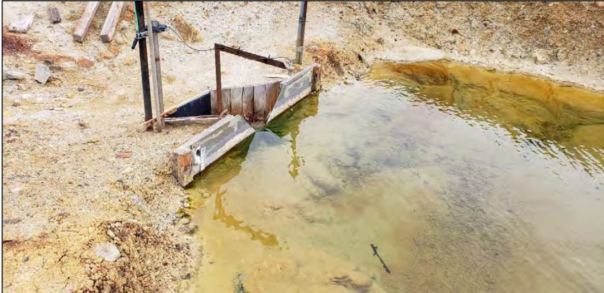
PHOTO 15 – Seep 10 Weir. (March 30, 2020)
