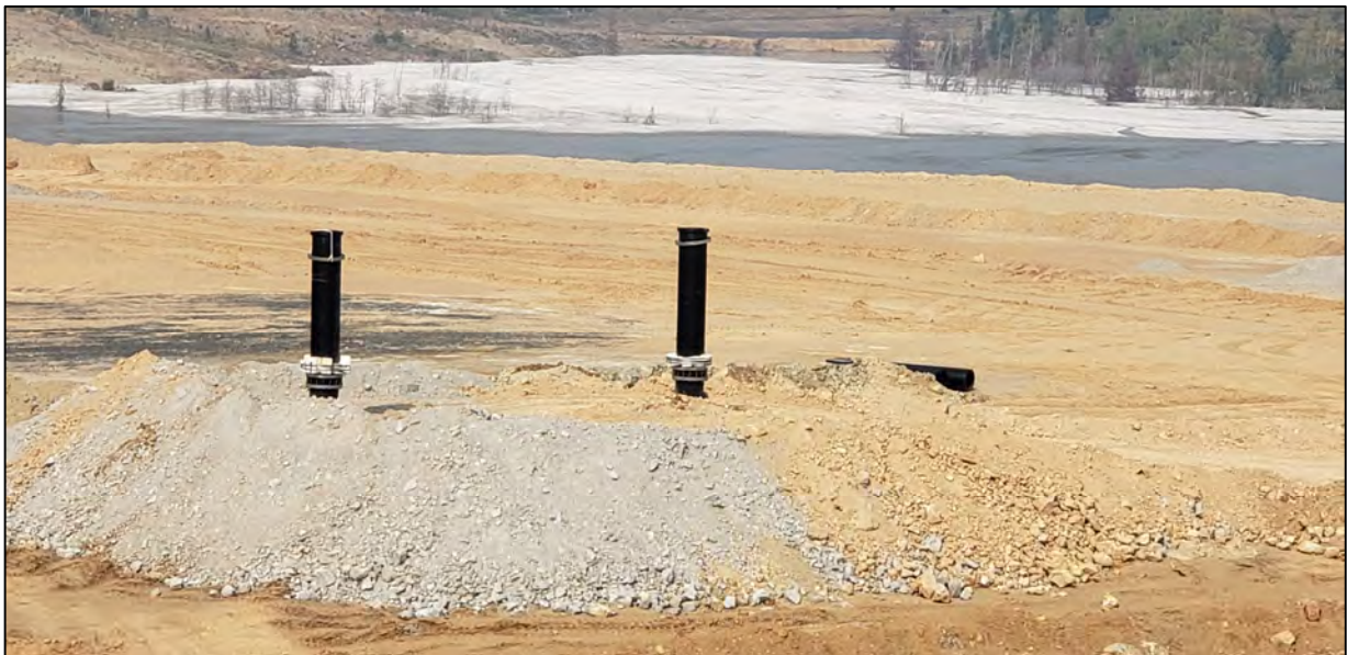
PHOTO 12 – West Embankment – Extraction Basin well risers
