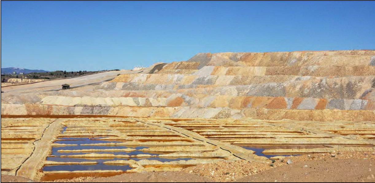
PHOTO 1 – North-South Embankment – Downstream step-out construction. (June 26, 2020)
