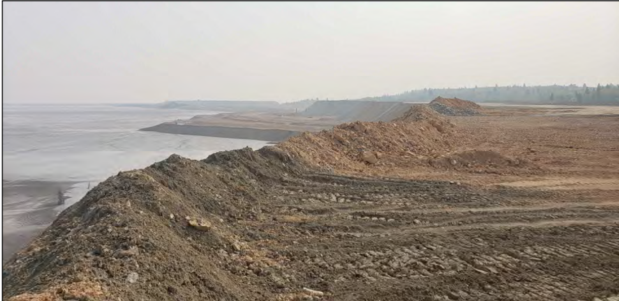
PHOTO 13 – West Embankment – EL 6,450 ft construction progress
