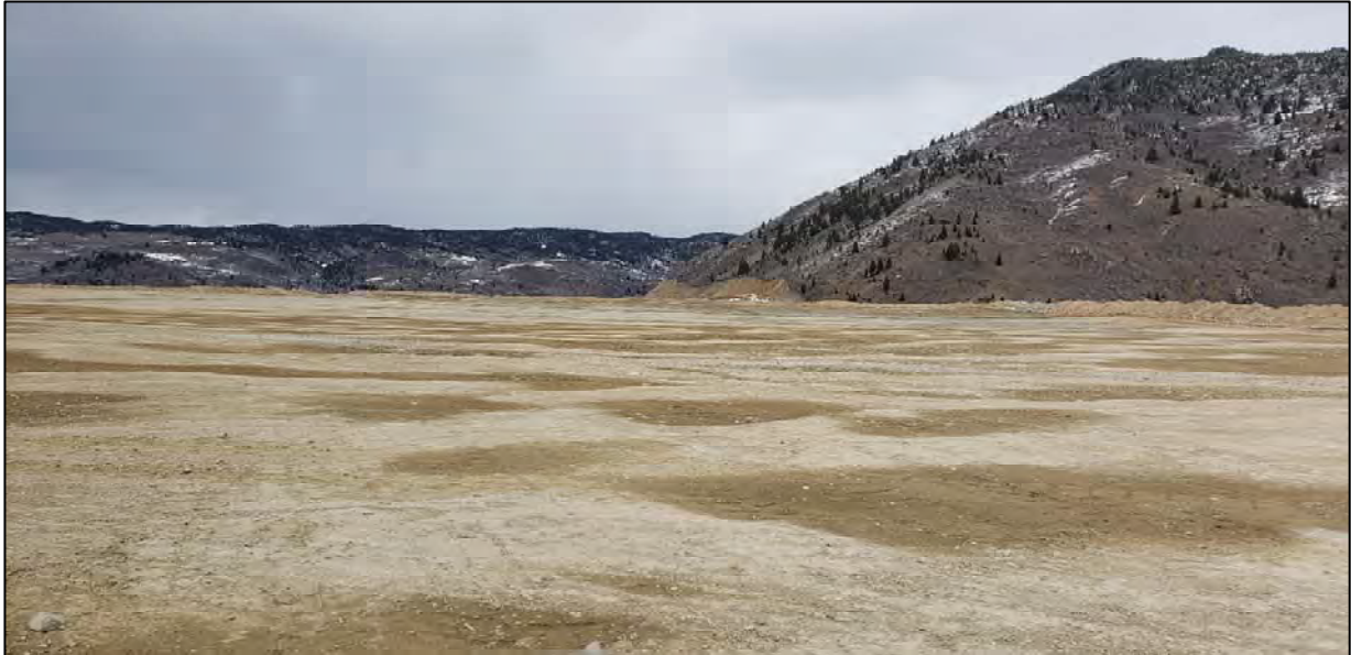
PHOTO 1 – North-South Embankment – Construction of the 6,400 ft lift. (March 30, 2020)
