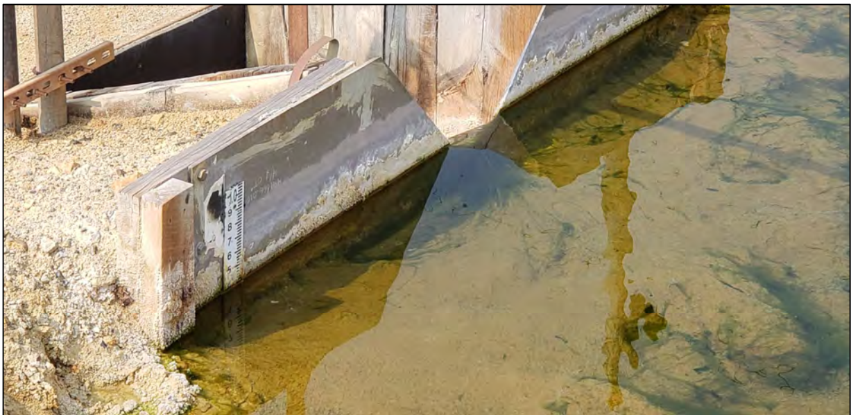
PHOTO 22 – Seep 10 Weir Staff Gauge reading approximately 0.4
