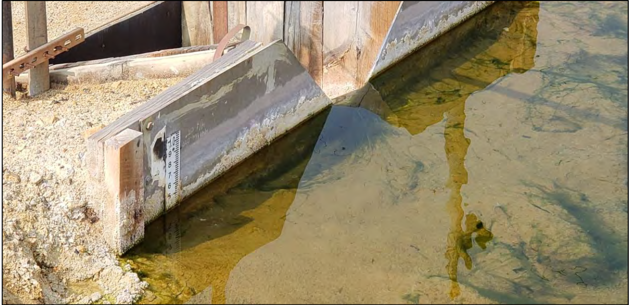
PHOTO 3 – Sep 16, 2020 – Seep 10 Weir and Staff Gauge.
