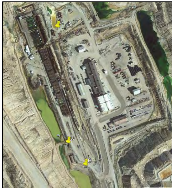
PHOTO 8 – Relevant locations regarding Hooligan Pond bypassing flows. A) Hooligan Pond; B) first discharge location; C) second discharge location.
