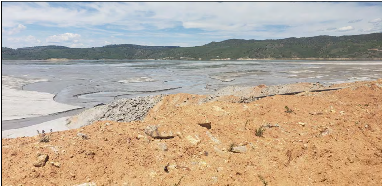
PHOTO 4 – North-South Embankment – Tailings beach and supernatant pond as viewed from the NS-2 discharge location. (June 26, 2020)
