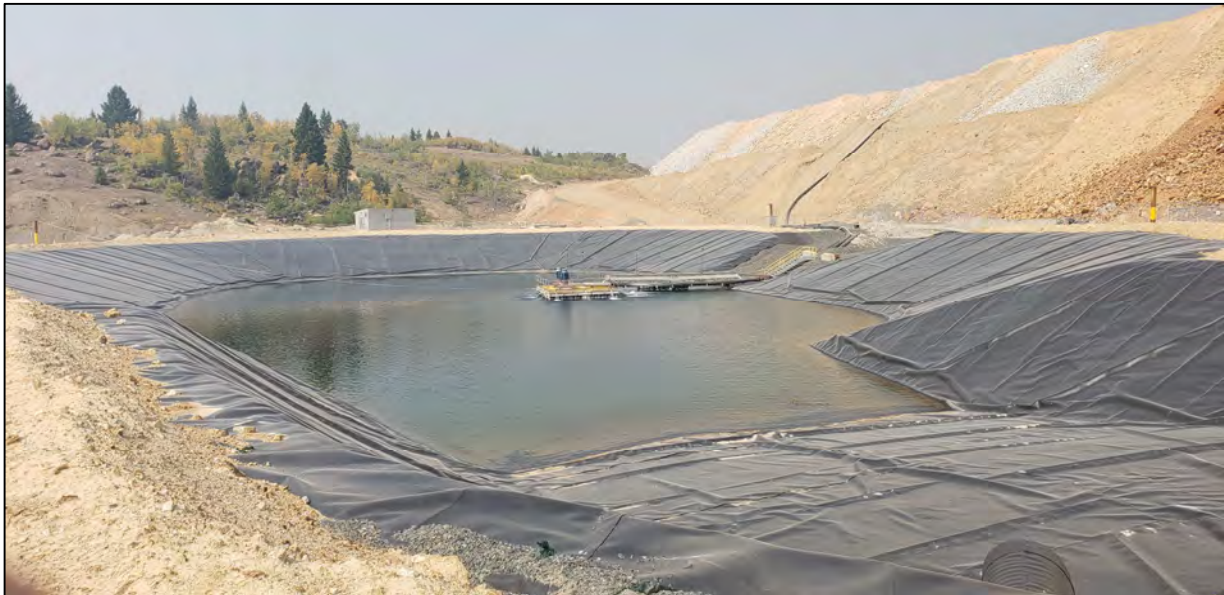
PHOTO 14 – West Embankment – Extraction Pond
