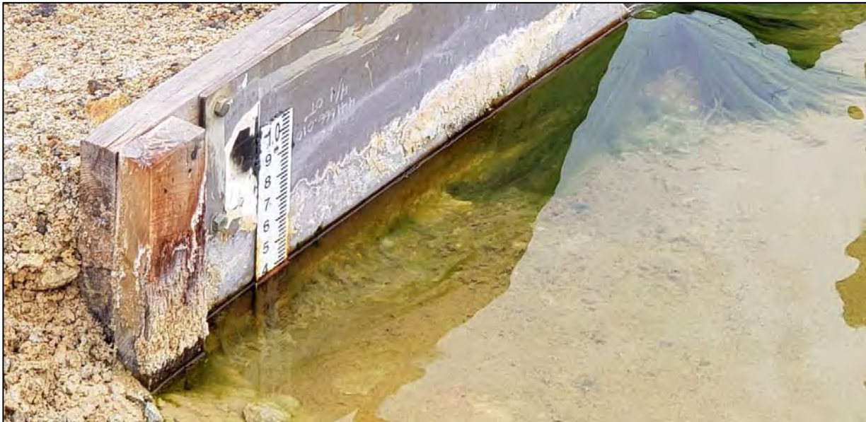
PHOTO 16 – Seep 10 Weir Staff Gauge reading approximately 0.38. (March 30, 2020)
