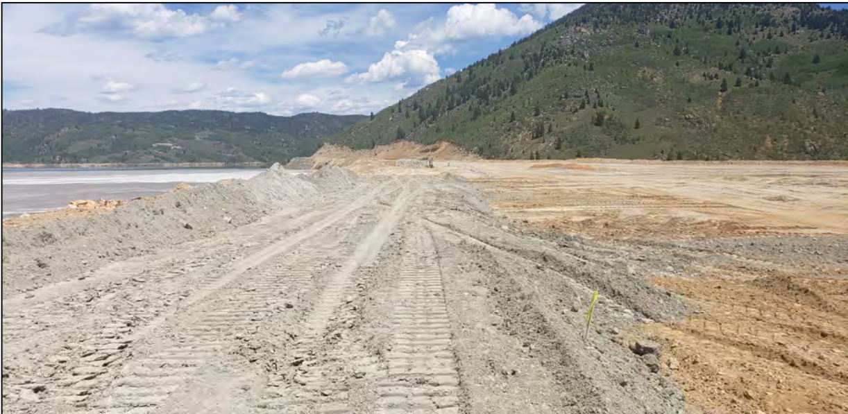
PHOTO 2 – North-South Embankment – Tailings discharge corridor construction, looking towards NS-3. (June 26, 2020)
