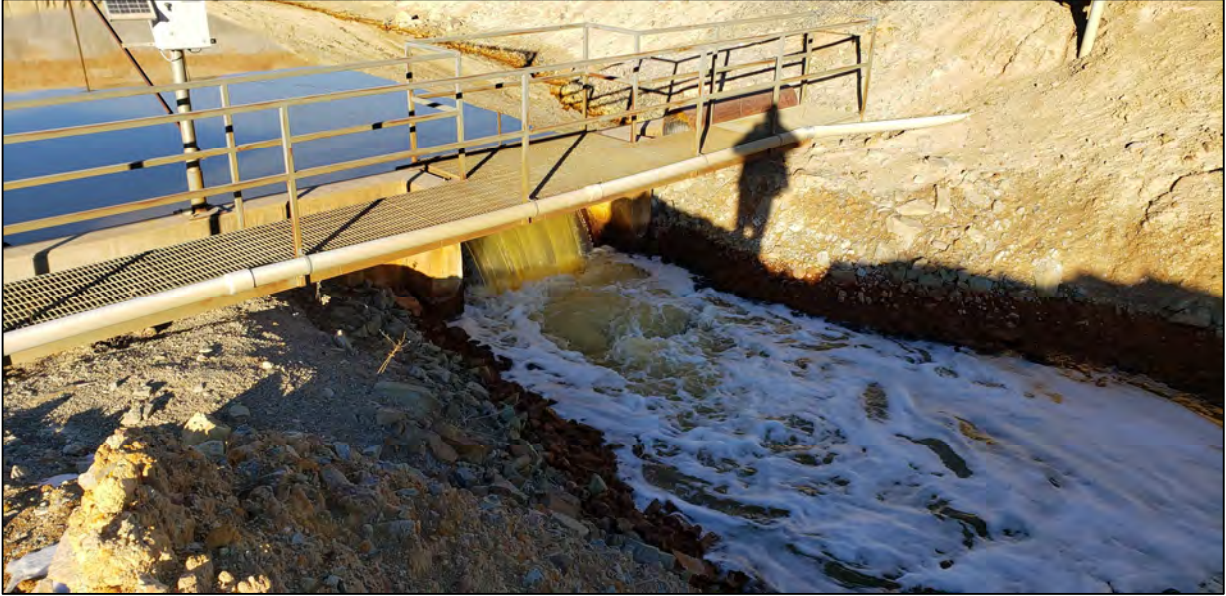
PHOTO 1 – Dec 10, 2020 – Flow through HsB Weir.
