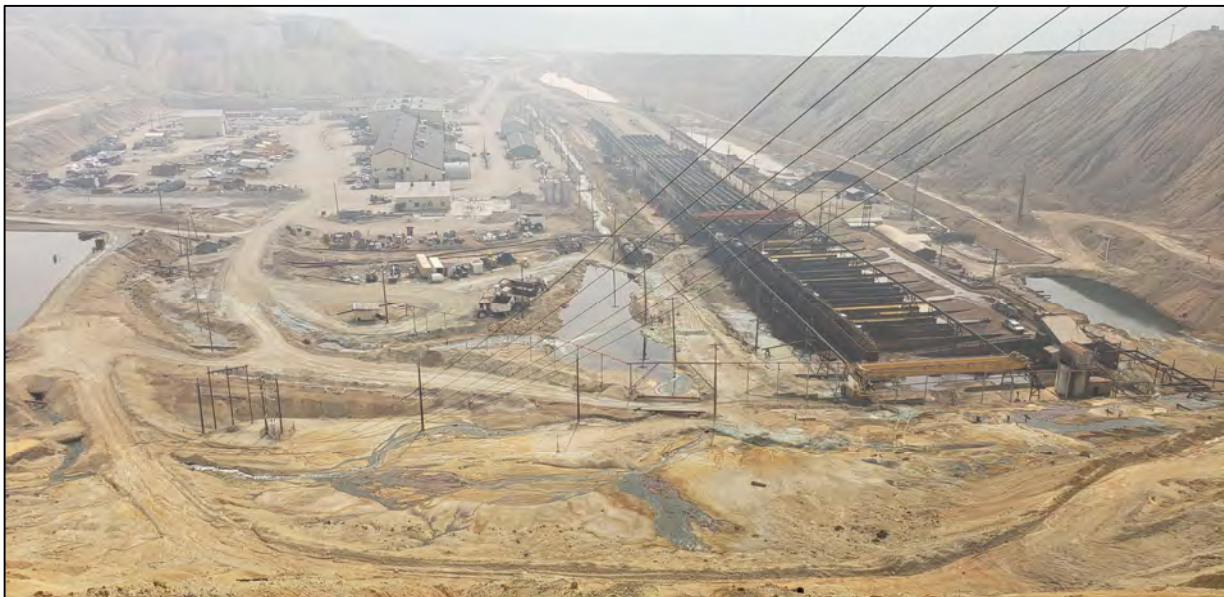
PHOTO 16 – Horseshoe Bend (HsB) Area – Leach seeps along toe of East-West Embankment viewed from Seep 10 bench.
