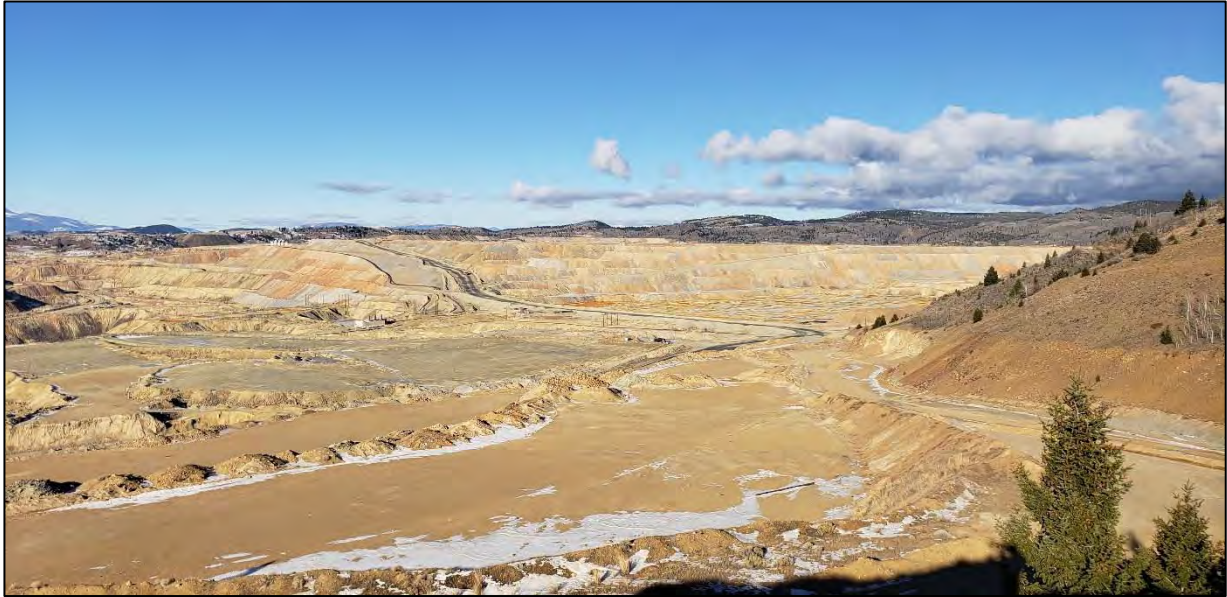
PHOTO 1 – North-South Embankment – Viewed from the Great Northern Dump
