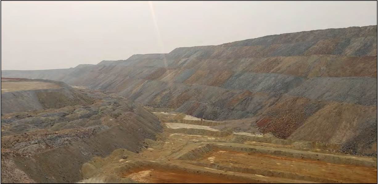
PHOTO 1 – North-South Embankment – Downstream step-out overview
