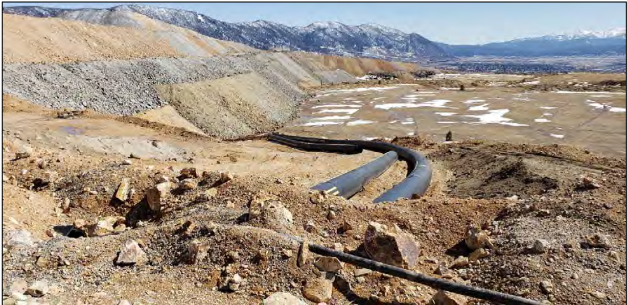
PHOTO 12 – West Embankment – Extraction Pond Emergency Pipelines, still under construction. (March 30, 2020)
