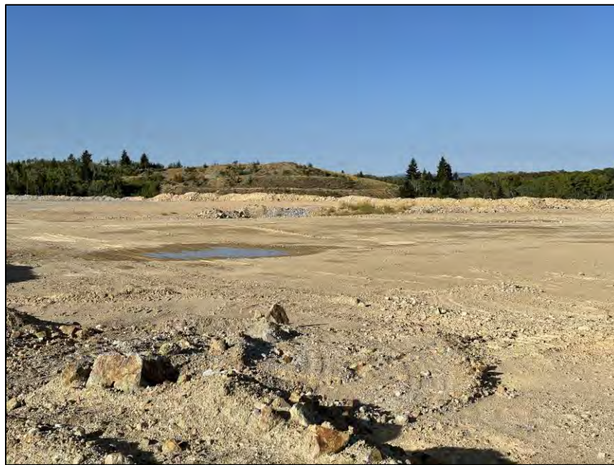
Photo 3.1 EL. 6,450 ft West Embankment Crest and Ponding
