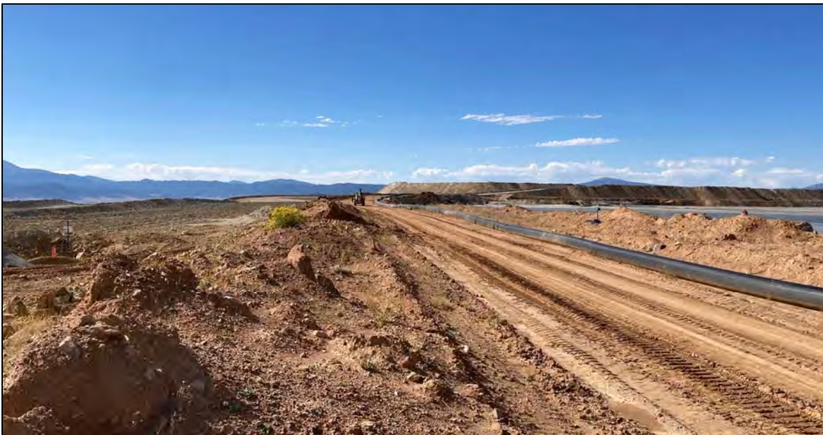
PHOTO 38 – North-South Embankment crest (left) and tailings discharge corridor (right), facing south.
