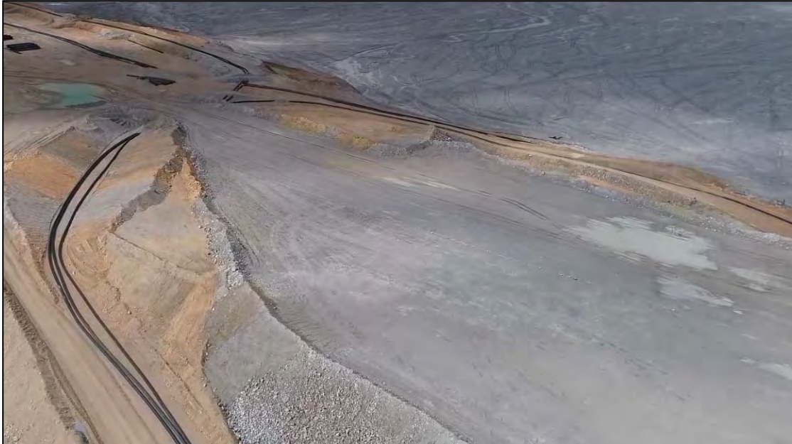
PHOTO 19 – East-West Embankment EL. 6,450 ft lift and surcharge zone, with view of adjacent tailings beach and Line 3, recently routed over the EL. 6,450 ft lift.
