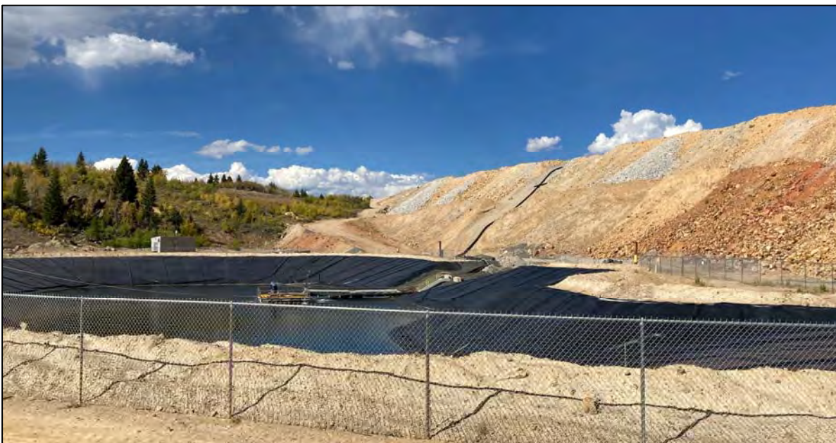
PHOTO 46 – WED Extraction Pond facing north along West Embankment.
