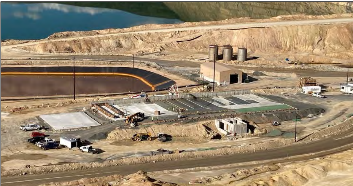
PHOTO 76 – New Precipitation Plant construction, facing west.
