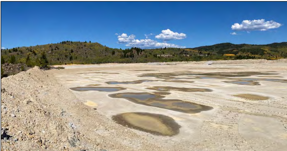
PHOTO 50 – Minor depressions and ponded water on downstream side of West Embankment crest, facing north at EL. 6,450 ft.
