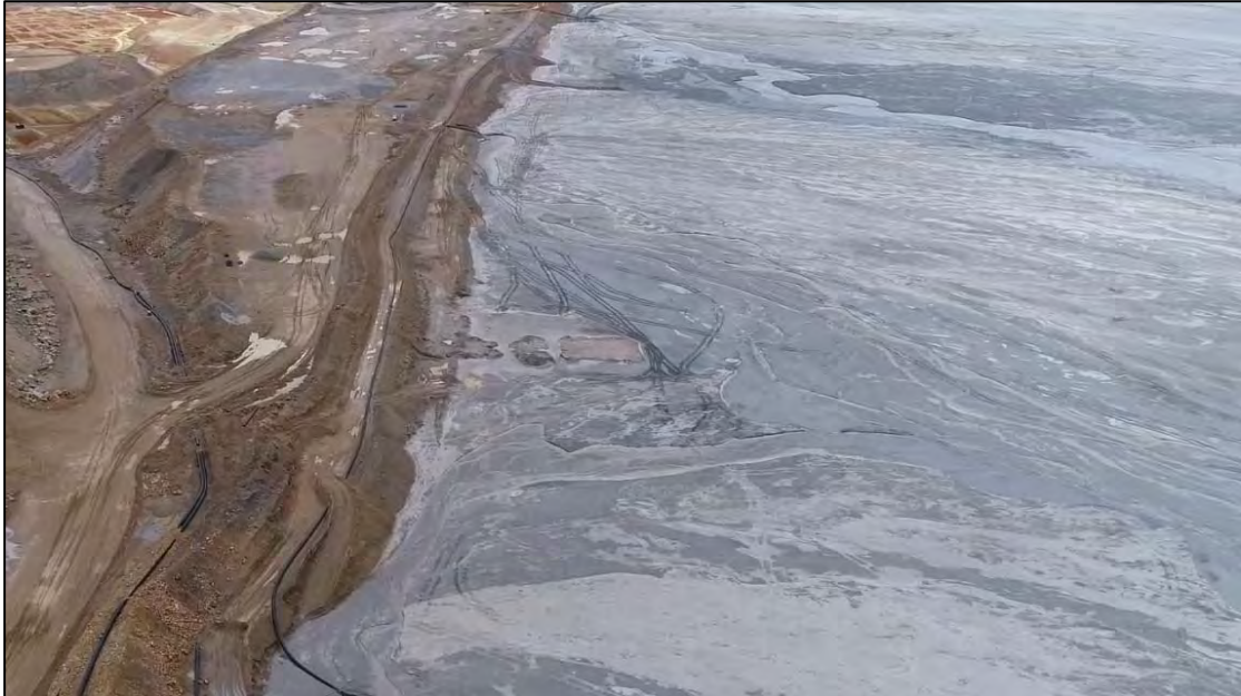
PHOTO 7 – North-South Embankment crest (left), tailings discharge corridor, and tailings beach (right) near tailings discharge NS-4.
