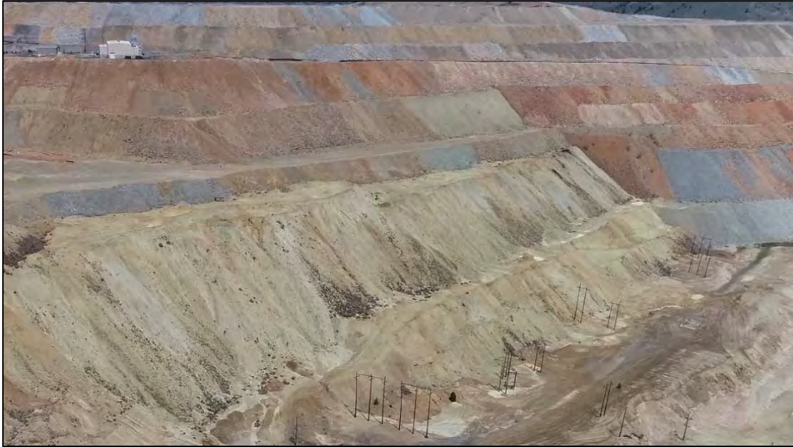
PHOTO 13 – Central pedestal area of the East-West Embankment, looking northeast.
