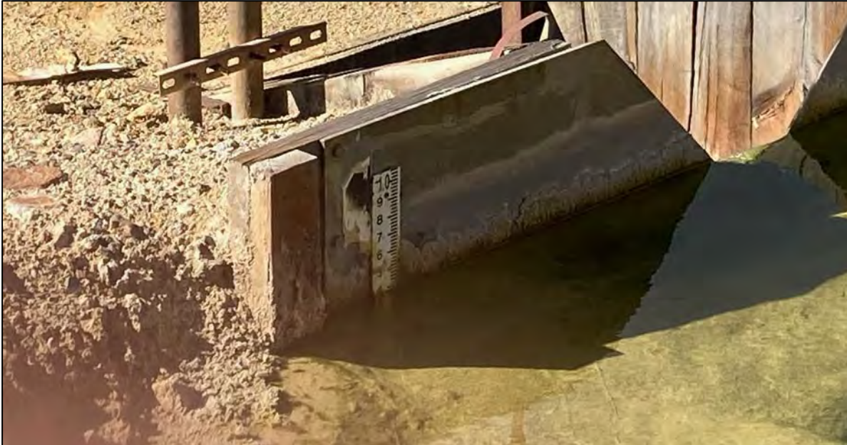
PHOTO 73 – Number 10 Seep V-notch weir staff gauge reading 0.38.
