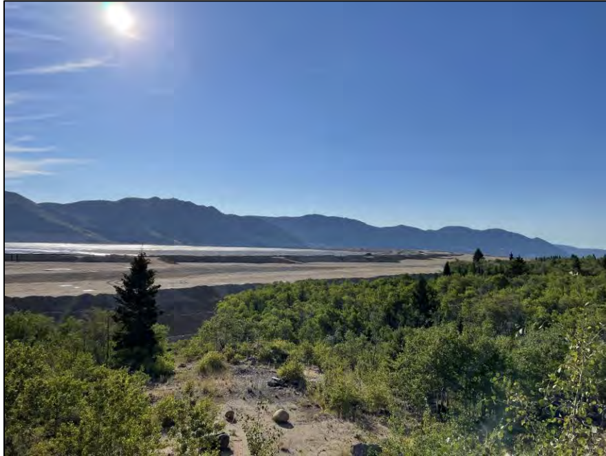
PHOTO 1 – West Embankment – Viewed from the topsoil stockpiles along the West Ridge
