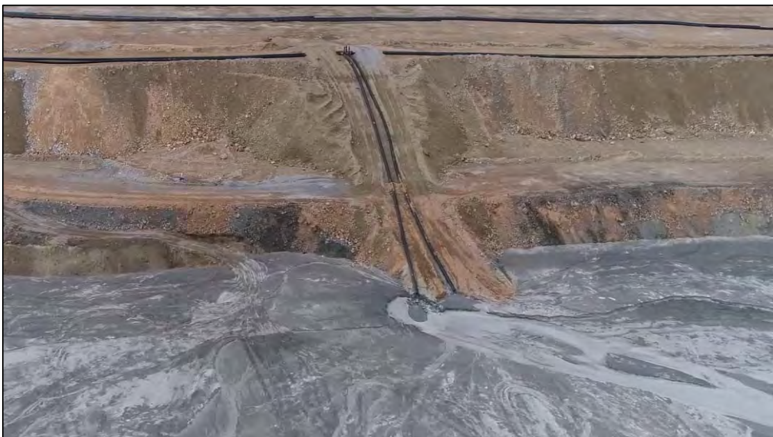
PHOTO 20 – East-West Embankment upstream side at discharge location EW-2, facing southwest.
