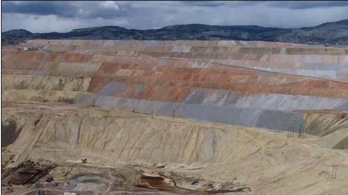
PHOTO 11 – East-West Embankment downstream slope and Number 10 Seep bench area, facing north.
