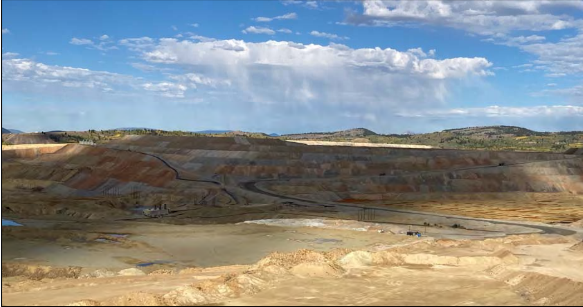
PHOTO 39 – East-West Embankment and North-South Embankment tie-in area downstream shell, facing northwest from Sunflower Hill.
