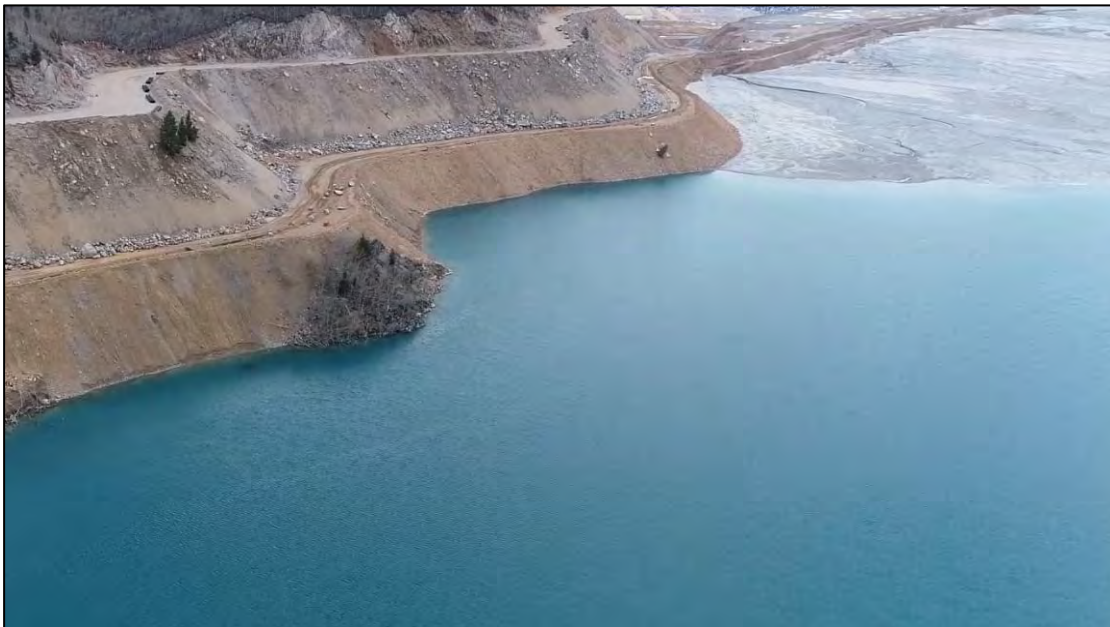
PHOTO 4 – New Reclaim Water Pipeline road, supernatant pond, and tailings beach, facing southeast.
