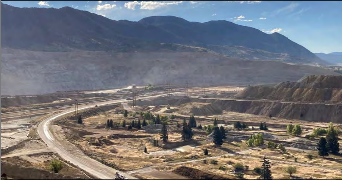
PHOTO 77 – Scalper Road On-site Containment Project construction progress, facing southeast.
