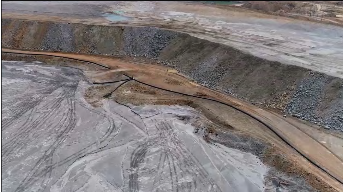
PHOTO 17 – East-West Embankment upstream face at discharge location EW-1, facing south.
