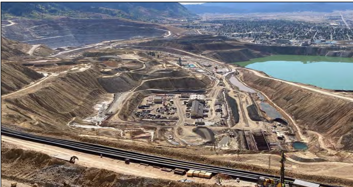
PHOTO 54 – Horseshoe Bend overview from East-West Embankment EL. 6,450 ft, facing south.
