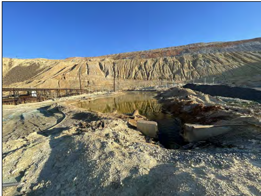
PHOTO 16 – Horseshoe Bend – Houligan Pond and overflow, looking north
