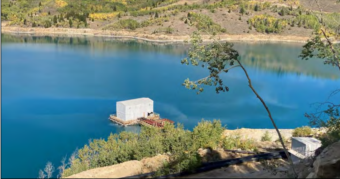
PHOTO 29 – Reclaim Barge and YDTI supernatant pond, facing west from the New Reclaim Water Pipeline road.
