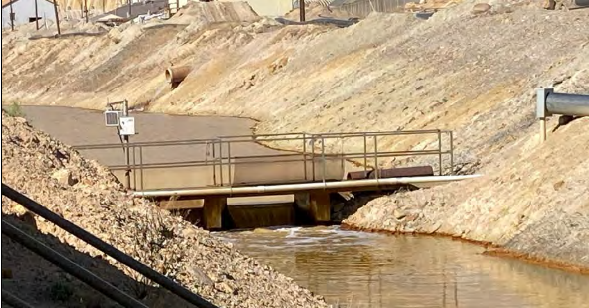
PHOTO 69 – Horseshoe Bend Weir, facing north.
