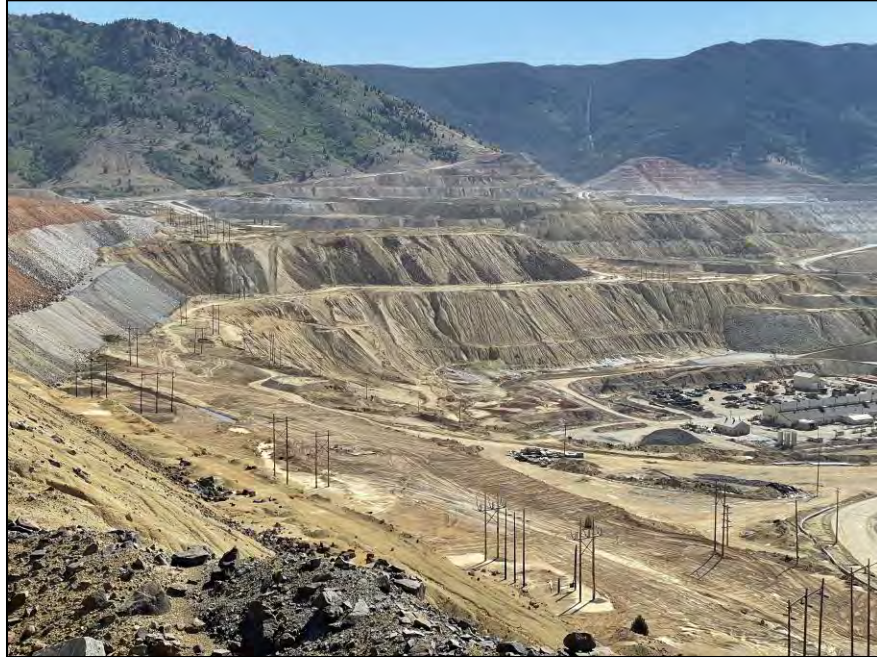
PHOTO 11 – Overview of the Seep 10 bench and Horseshoe Bend Area, looking east
