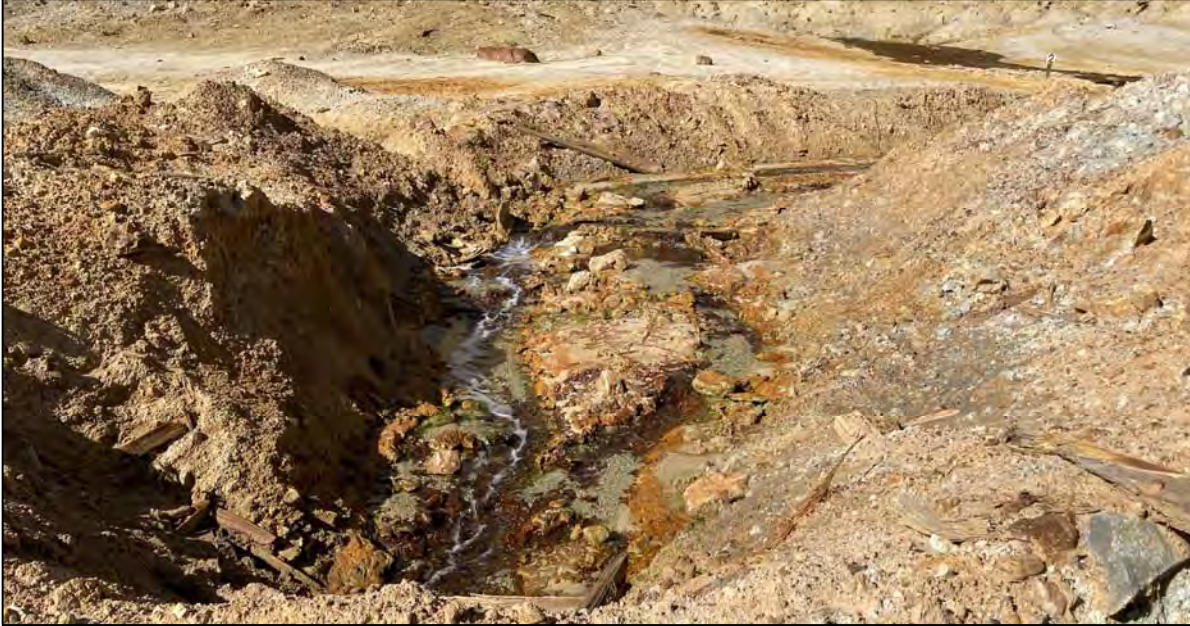
PHOTO 61 – Houligan Pond inflow in ditch collecting embankment toe seepage and conveying surface water flow from the Holding Pond to the Houligan Pond, facing north from the Houligan Pond.
