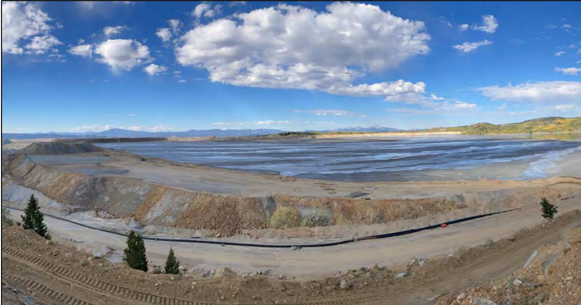
PHOTO 33 – North-South Embankment and beach, looking west from the New Reclaim Water Pipeline ramp.
