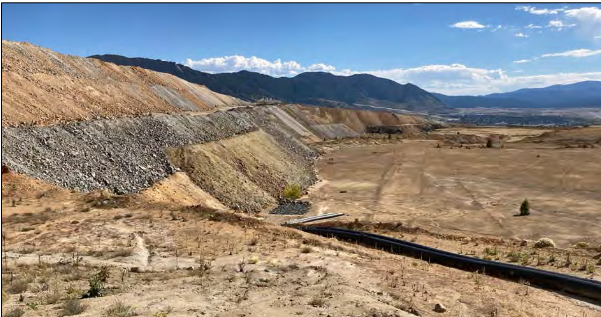
PHOTO 44 – East-West Embankment downstream slopes and WED Extraction Pond emergency overflow pipelines, west of Booster Station #3, facing southeast near Extraction Pond. Boulders for energy dissipation and final alignment of pipeline discharge remains to be completed.
