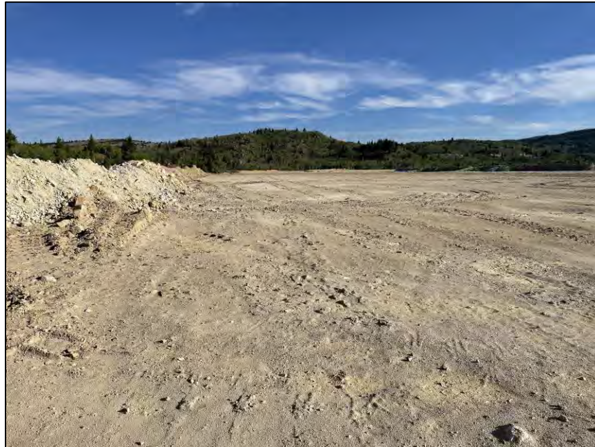
Photo 3.2 Completed Zone D1 – North of the Ridge Road at EL. 6,450 ft
