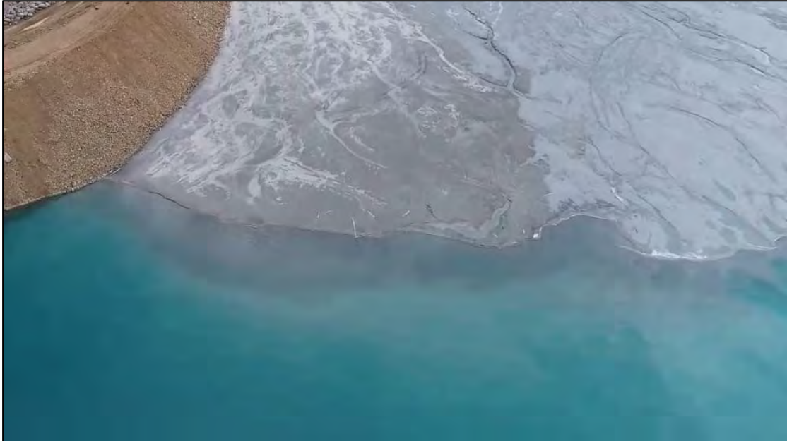
PHOTO 5 – Tailings beach and supernatant pond interface, looking south from the supernatant pond.
