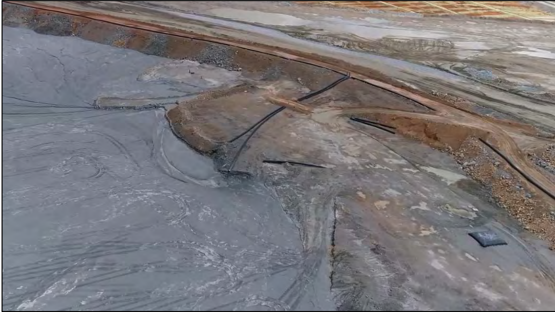
PHOTO 9 – Discharge location NS-1 along the North-South Embankment, facing east.
