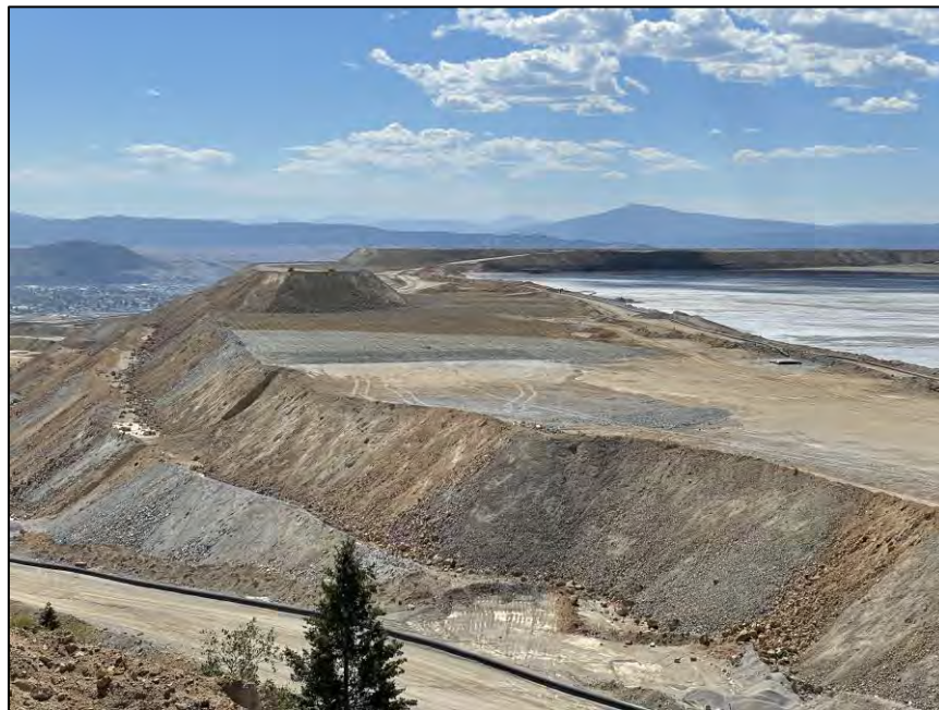
Photo 3.5 EL. 6,450 ft North-South Embankment Construction
