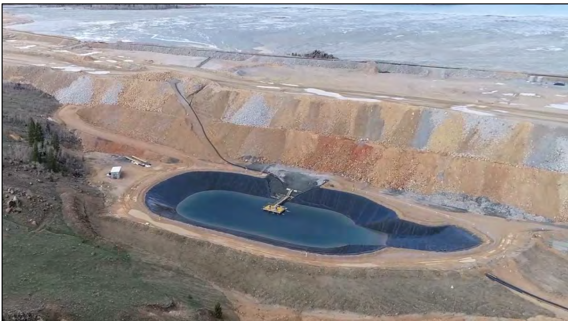
PHOTO 28 – Overview of WED Extraction Pond.
