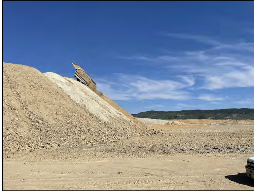
Photo 3.3 EL. 6,450 ft East-West Embankment Construction Near Section 0+00
