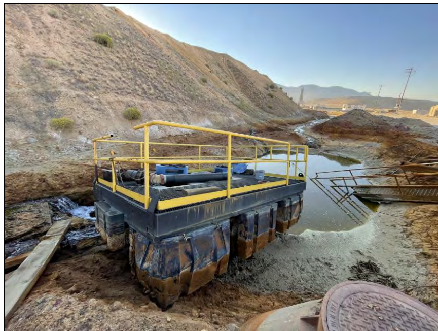
Photo 3.10 Decommissioned Muddler Pump Area
