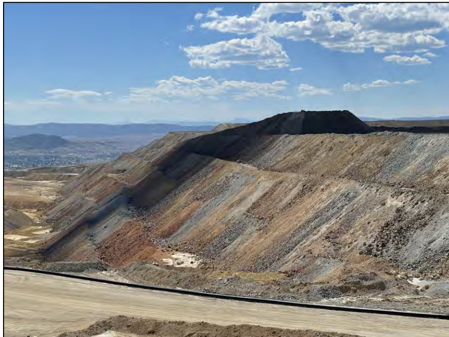
PHOTO 10 – North-South Embankment – Overview of embankment downstream slope
