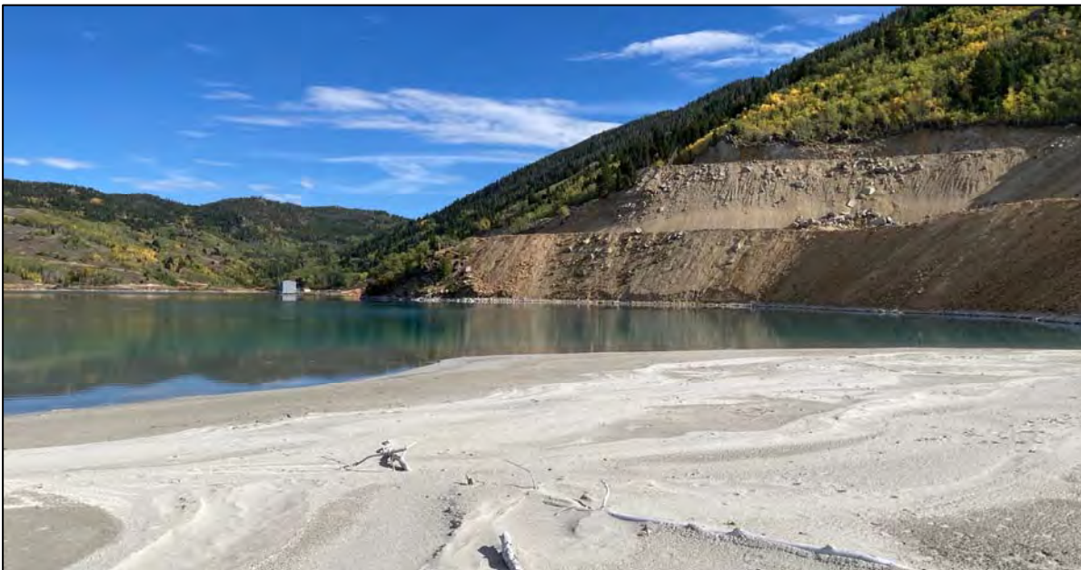
PHOTO 32 – YDTI tailings beach and supernatant pond interface, facing north.
