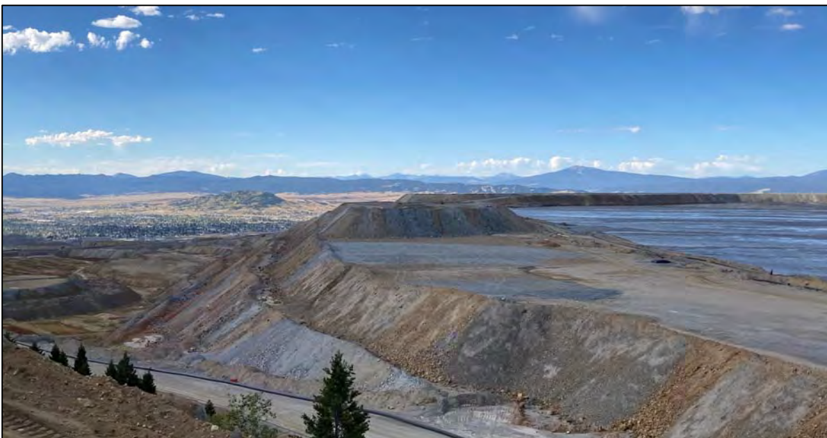
PHOTO 34 – North-South Embankment downstream side, looking southwest from New Reclaim Water Pipeline ramp.
