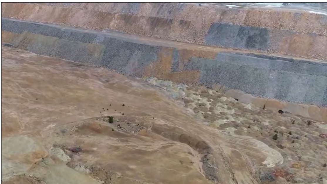
PHOTO 18 – East-West Embankment downstream slope along the northwest dumps area, facing northeast.
