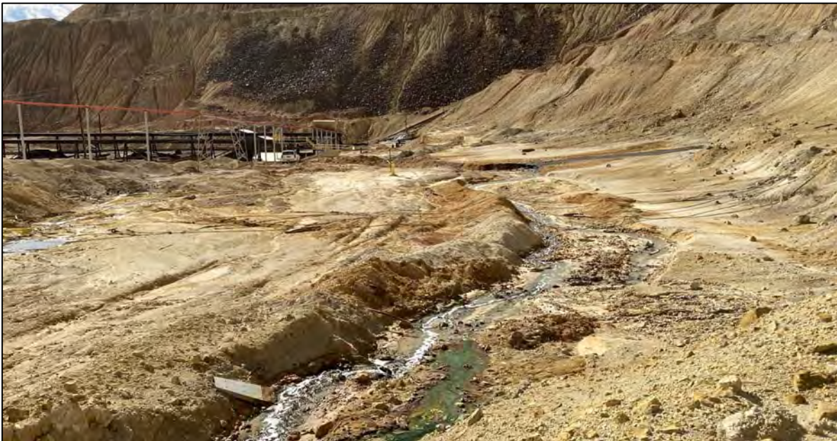
PHOTO 62 – Ditch conveying surface water flows from the Holding Pond, around the perimeter of the historical Surge Pond, to the Houligan pond, facing west.
