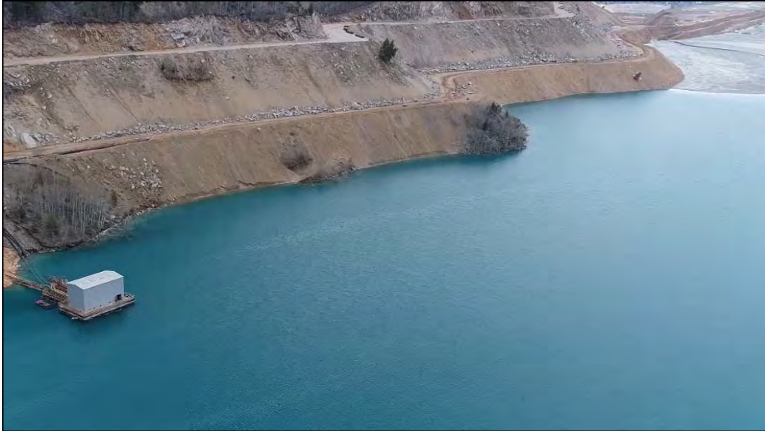
PHOTO 3 – Old Reclaim Barge and New Reclaim Water Pipeline Ramp road.
