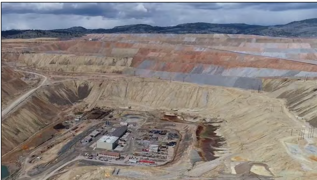
PHOTO 12 – Overview of Central Pedestal Area of the East-West Embankment, Seep 10 Bench, and HsB Area, facing north.
