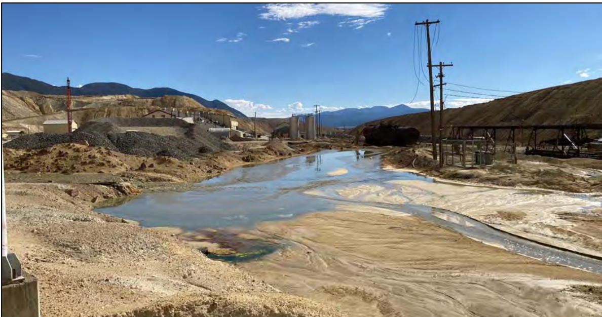
PHOTO 60 – Zone 2B stockpile (left) and Houligan Pond (center), facing south.
