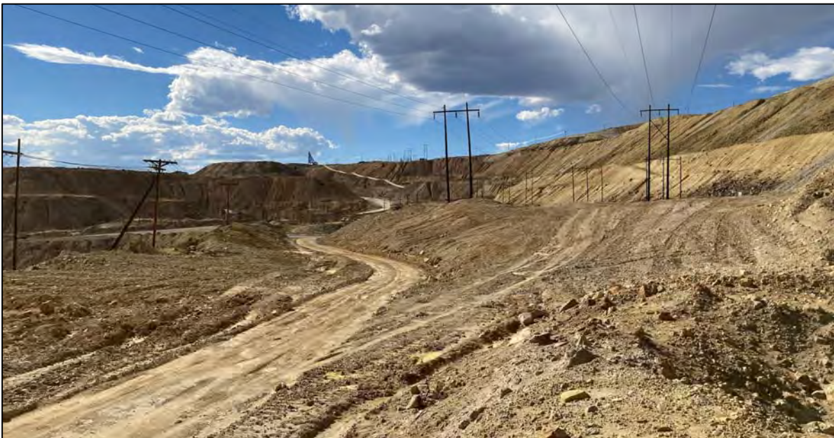
PHOTO 72 – Regrading progress of the Number 10 Seep bench area, looking west.
