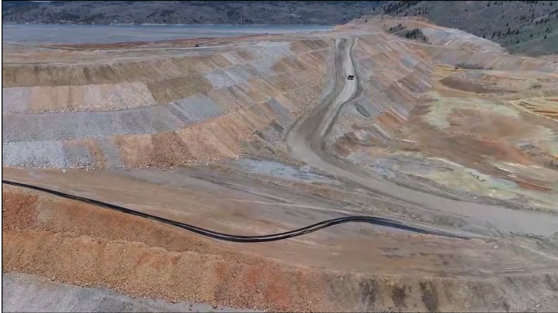
PHOTO 1 – North-South Embankment downstream shell, facing north from southeast end of YDTI.
