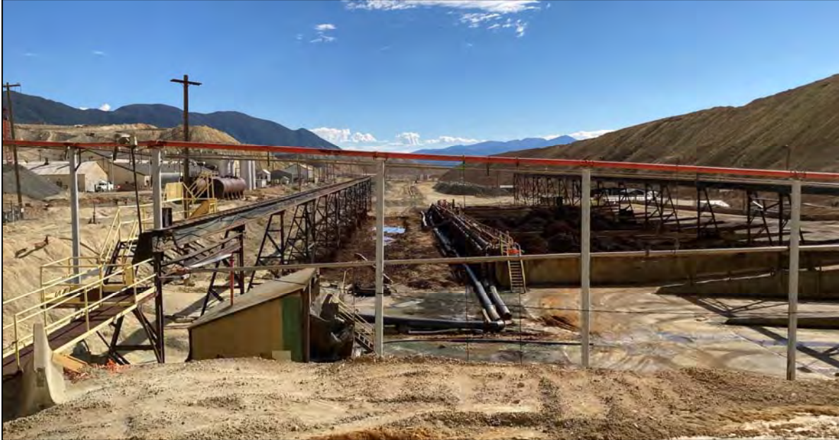
PHOTO 63 – Decommissioned Precipitation Plant, facing south
