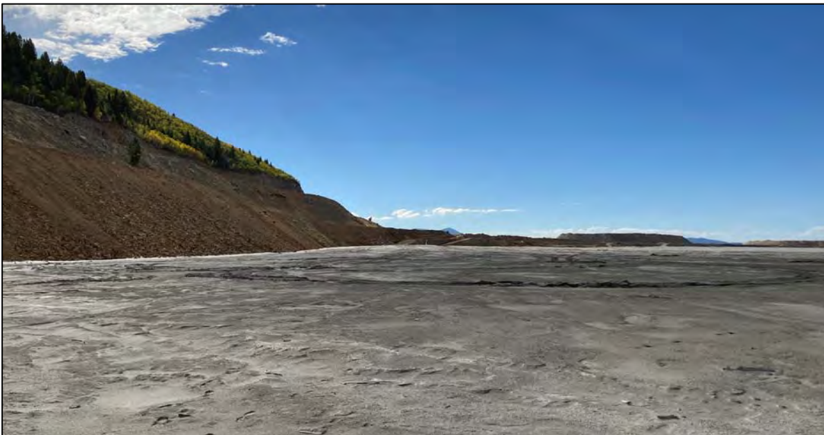
PHOTO 36 – Tailings beach north of tailings discharge location NS-4 and by New Reclaim Water Pipeline Ramp hillside cut, facing south.
