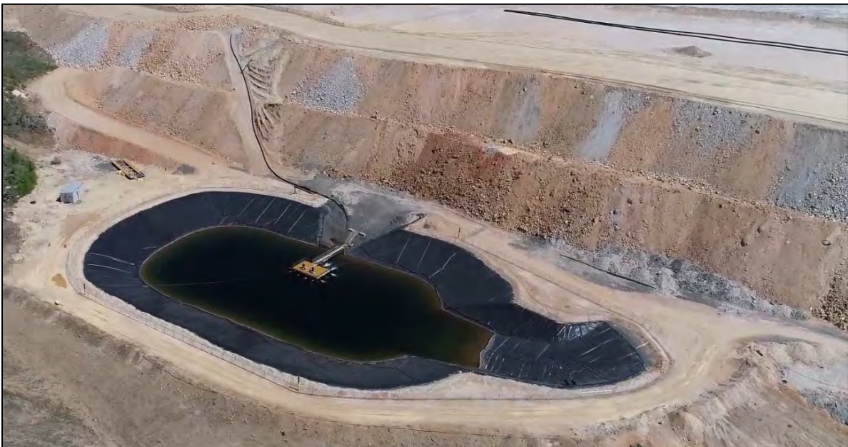
PHOTO 26 – Overview of WED Extraction Pond.
