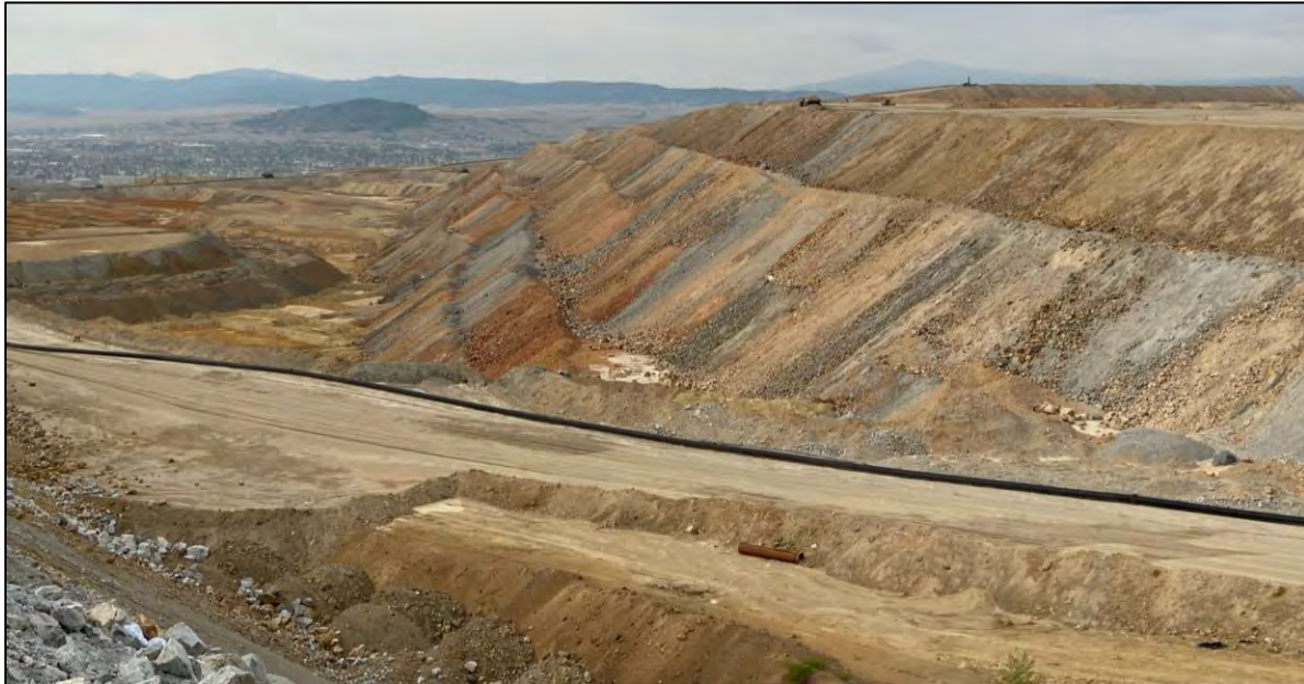
PHOTO 27 – North-South Embankment downstream side, looking southwest from New Reclaim Water Pipeline ramp.
