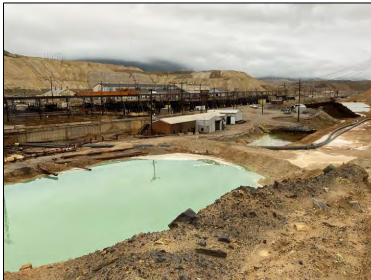
Photo 3.1 Water ponding within the upper HsB Area
