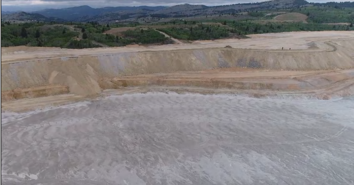
PHOTO 21 – West Embankment upstream interface north of Rocky Knob, by discharge location RK-2 (temporarily disconnected during drone survey), facing west near the Extraction Pond.
