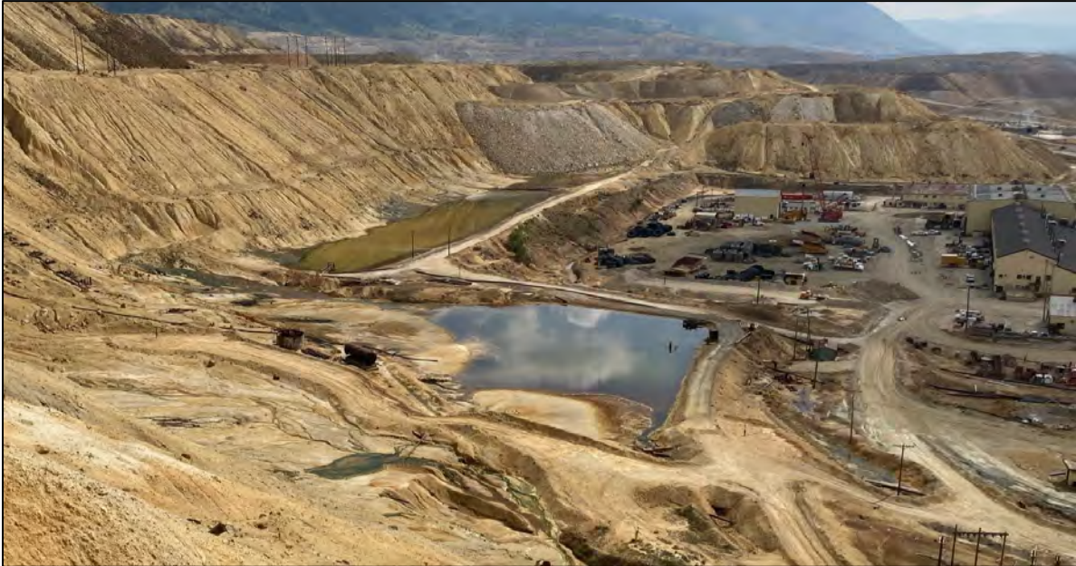
PHOTO 55 – Holding Pond and Surge Pond in the HsB Area, looking southeast from Number 10 Seep Bench.
