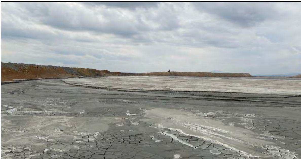
PHOTO 32 – Tailings beach near tailings discharge locations NS-2 and NS-3 along North-South Embankment, facing south.
