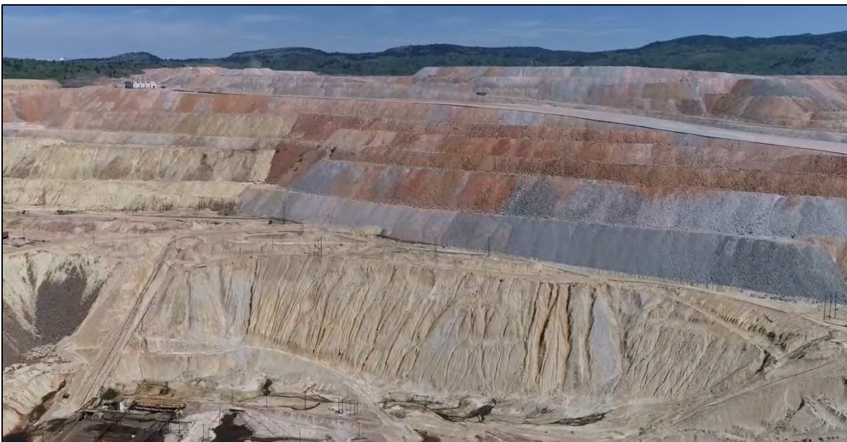
PHOTO 10 – East-West Embankment downstream slope and Number 10 Seep bench area, looking north.
