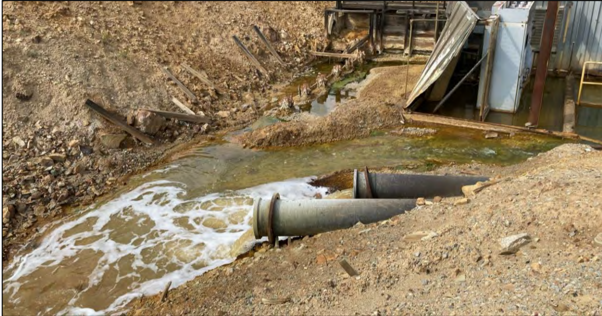
PHOTO 67 – Precipitation Plant overflow pipelines outflow, south of Cell 10 Pump facing north.
