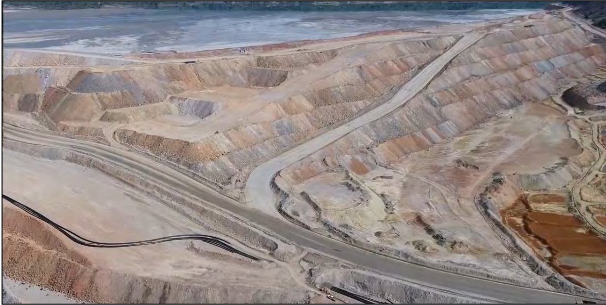
PHOTO 1 – North-South Embankment downstream shell, looking northwest from southeast end of YDTI.
