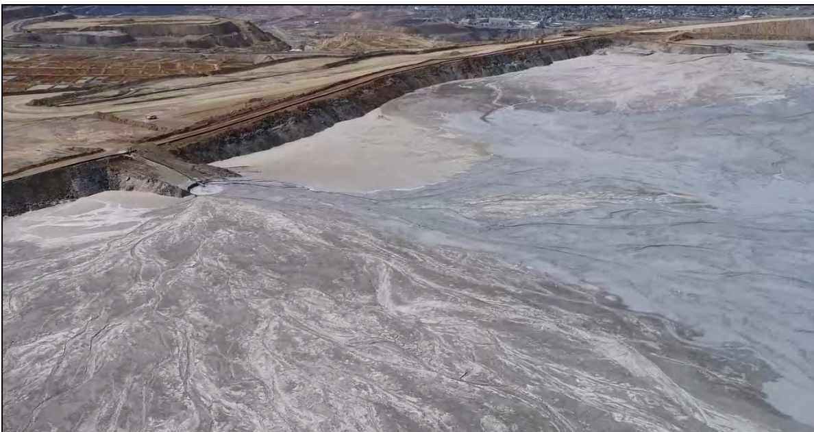
PHOTO 8 – Upstream side of the North-South Embankment between discharge locations NS-2 (left side) and NS-1 (right side), looking south.
