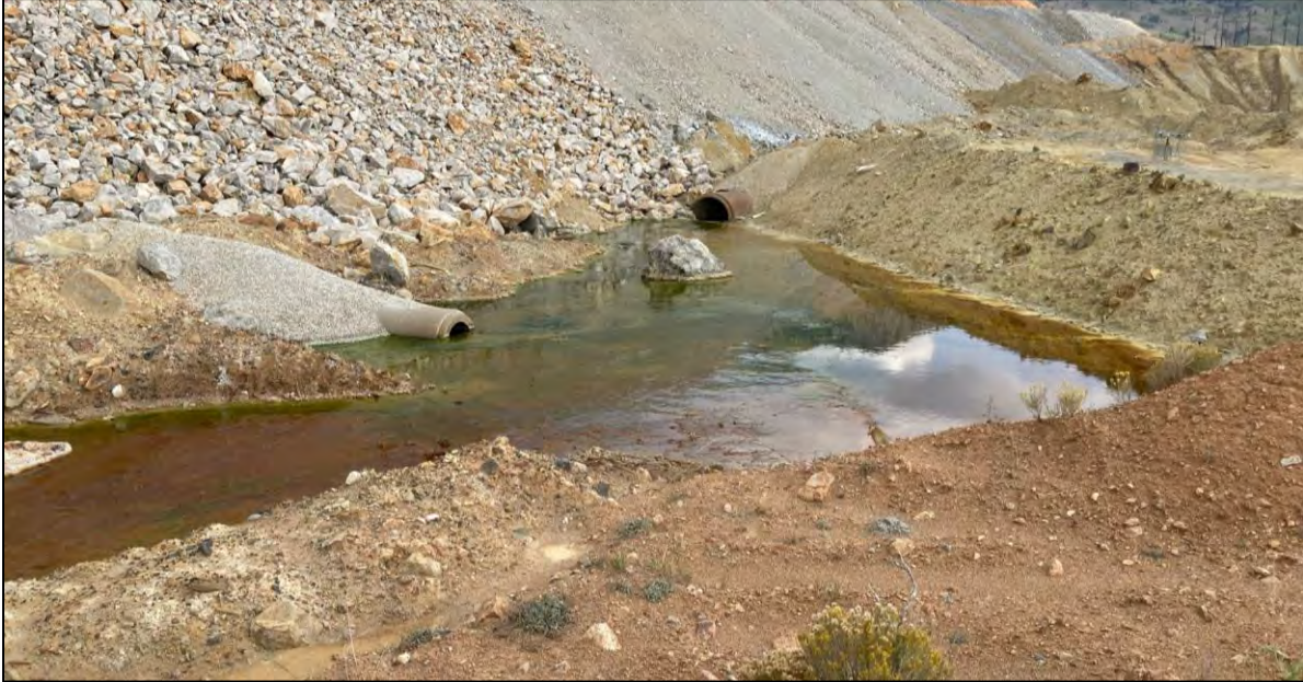
PHOTO 69 – Seepage at the Number 10 Seep bench area, looking east.
