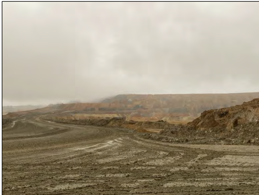
PHOTO 16 – North-South Embankment – EL. 6,250. EL. 6,300 ft Zone U construction progress
