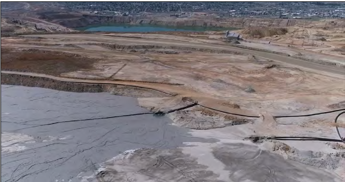
PHOTO 16 – East-West Embankment upstream face at discharge location EW-1 facing south.
