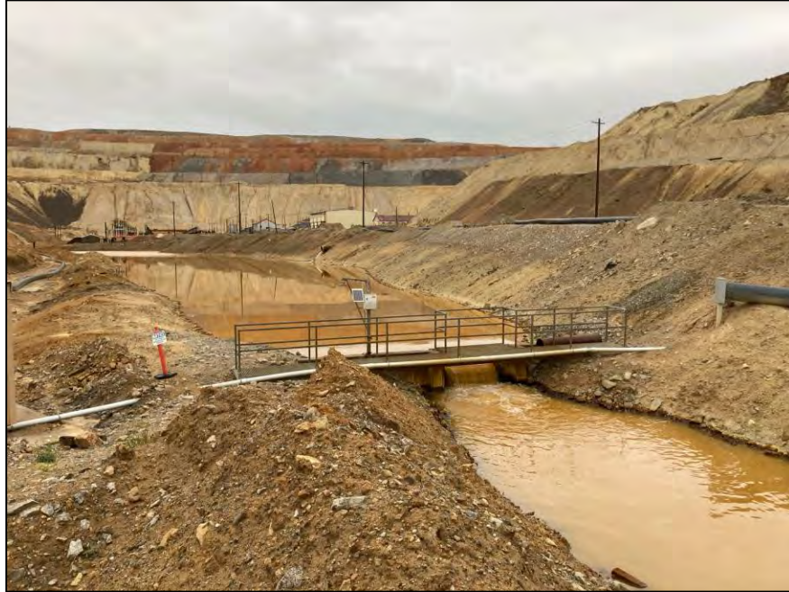
PHOTO 1 – HsB Weir and Pond facing North
