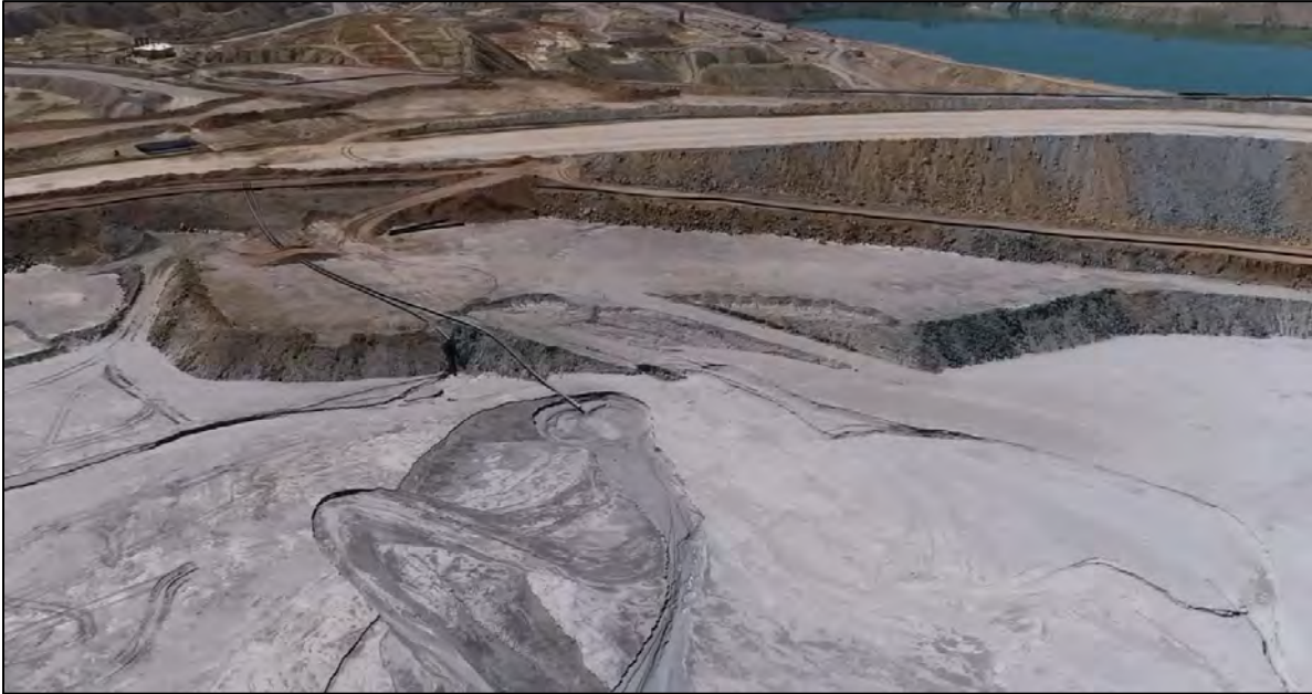
PHOTO 9 – Discharge location NS-1 along the North-South Embankment facing southeast.
