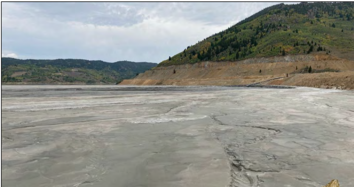
PHOTO 30 – Tailings beach by tailings discharge location NS-4 and New Reclaim Water Pipeline Ramp hillside cut, facing north.
