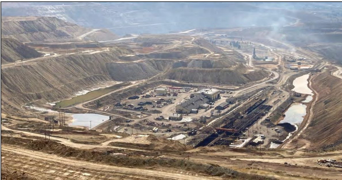
PHOTO 54 – Horseshoe Bend overview from East-West Embankment EL. 6,350 ft, facing southeast.
