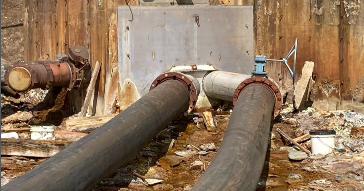
PHOTO 63 – Bulkhead replacement for discharge lines from the #5 and #6 Cells.
