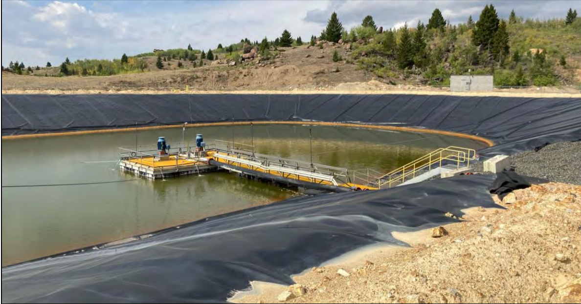
PHOTO 45 – WED Extraction Pond facing northwest.
