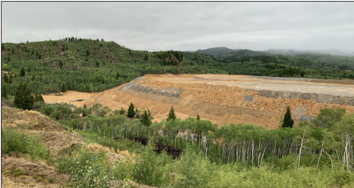
PHOTO 8 – West Embankment – EL. 6,450 ft Zone D1 construction at the Bumtown area
