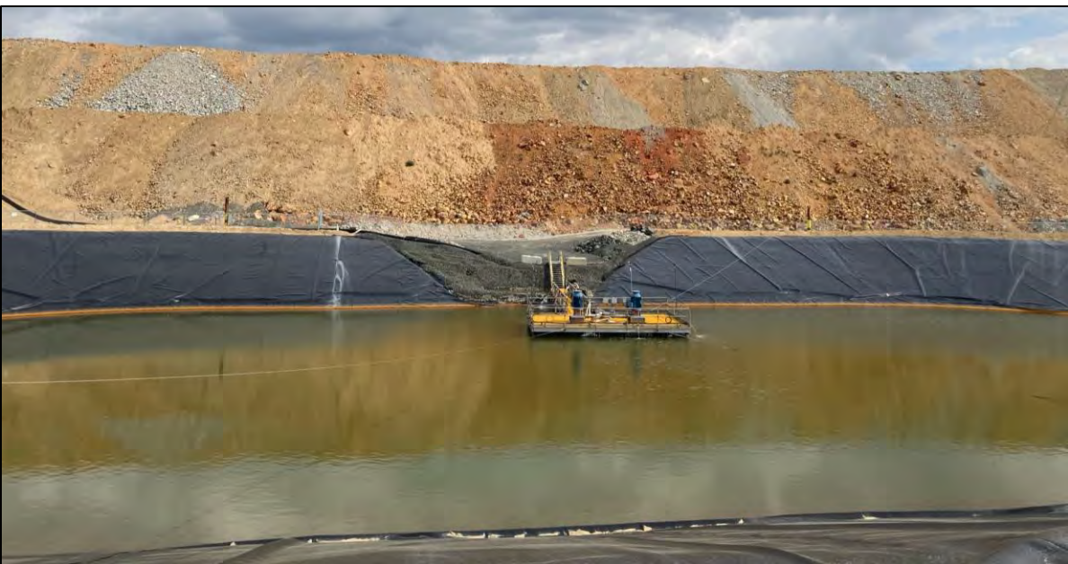
PHOTO 46 – WED Extraction Pond facing northeast.
