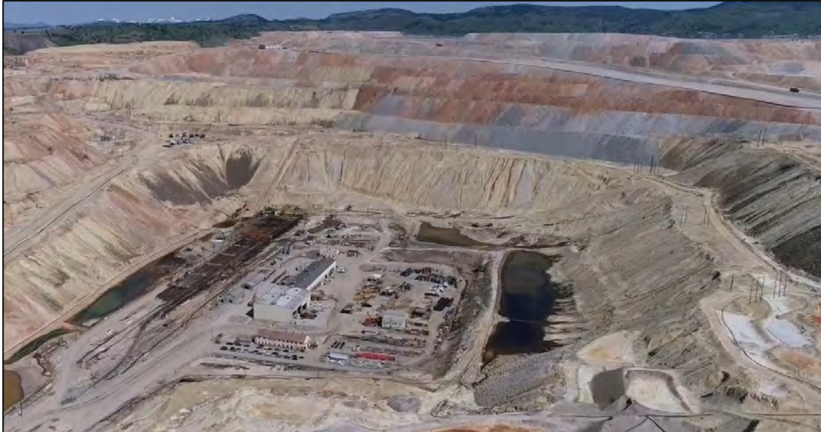
PHOTO 11 – Overview of Central Pedestal Area of the East-West Embankment, Seep 10 Bench, and HsB Area, looking north.
