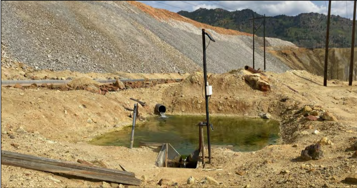
PHOTO 73 – Overview of Number 10 Seep stilling pond.
