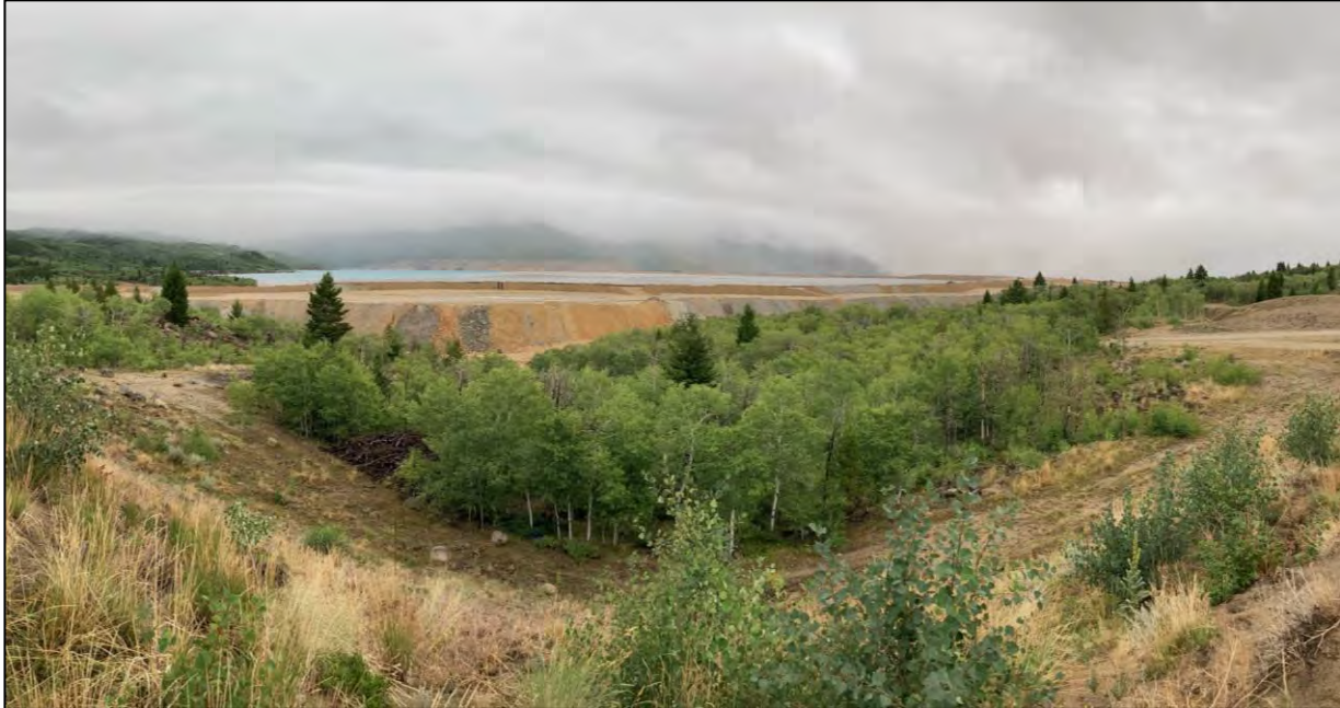
PHOTO 7 – West Embankment – EL. 6,450 ft lift, viewed from the topsoil stockpile along the West Ridge
