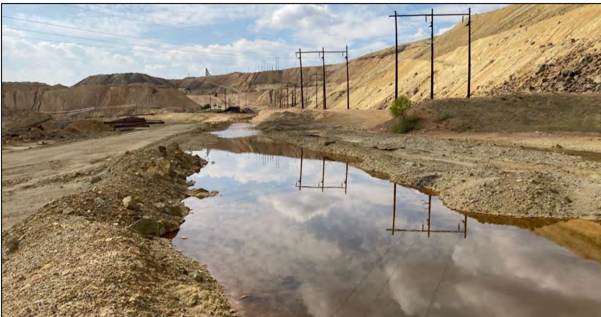
PHOTO 68 – Seepage at the Number 10 Seep bench area, looking west.
