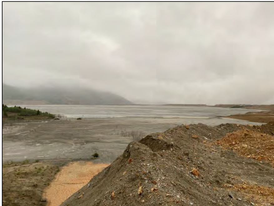
PHOTO 10 – West Embankment – Tailings beach, viewed from the old tailings discharge corridor near discharge location RK-4
