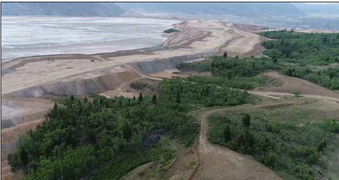
PHOTO 24 – West Embankment downstream shell, looking southeast.
