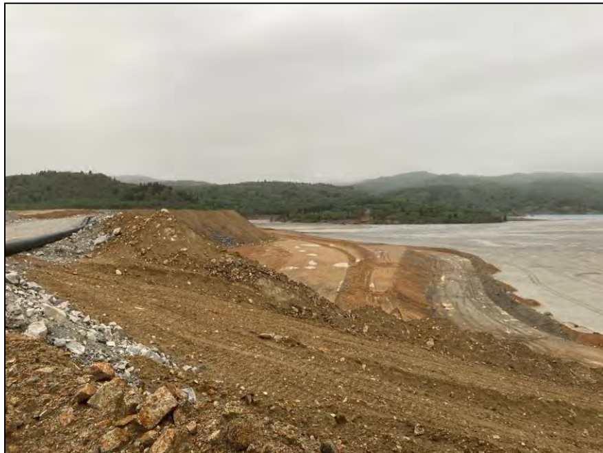
PHOTO 12 – West Embankment – EL. 6,450 tailings discharge corridor looking North
