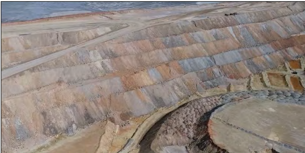
PHOTO 2 – North-South Embankment downstream shell, looking northwest towards the top of the mine haul ramp at EL. 6,400 ft
