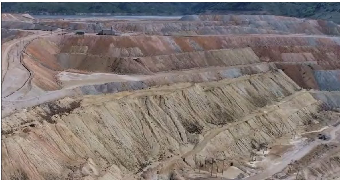
PHOTO 12 – Central pedestal area of the East-West Embankment, looking northeast.
