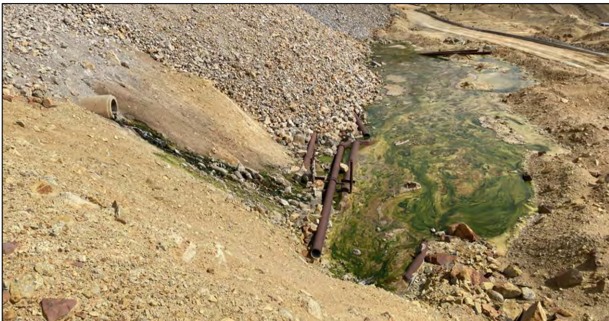
PHOTO 70 – Seepage at the Number 10 Seep bench area, looking east.
