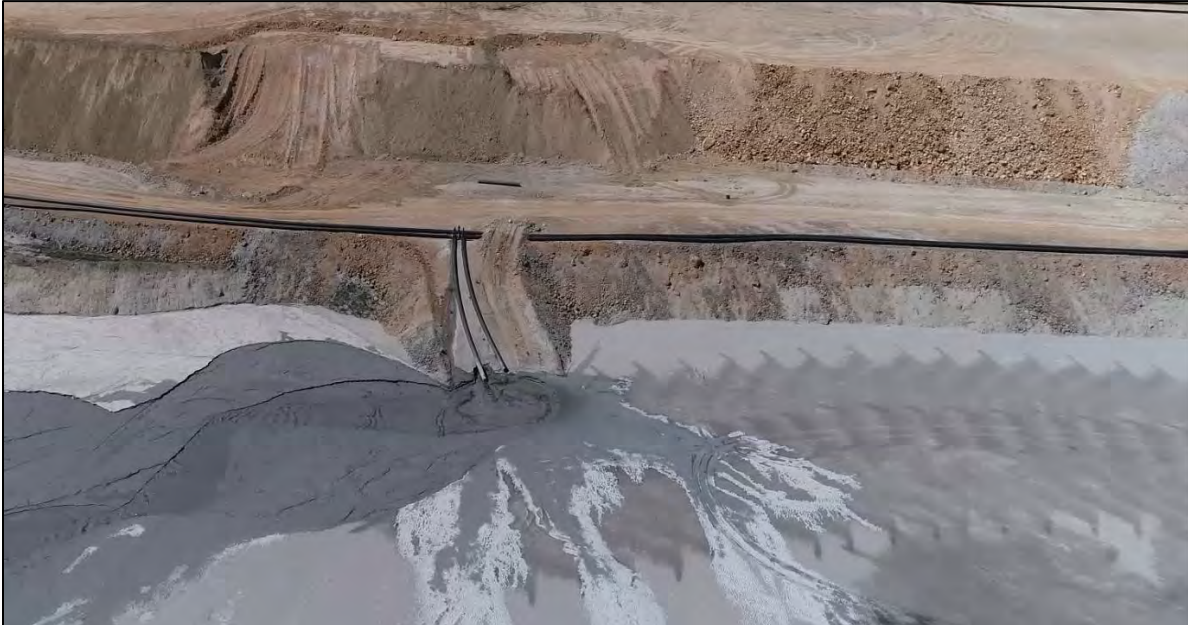
PHOTO 19 – East-West Embankment upstream side at discharge location EW-2, facing southwest.
