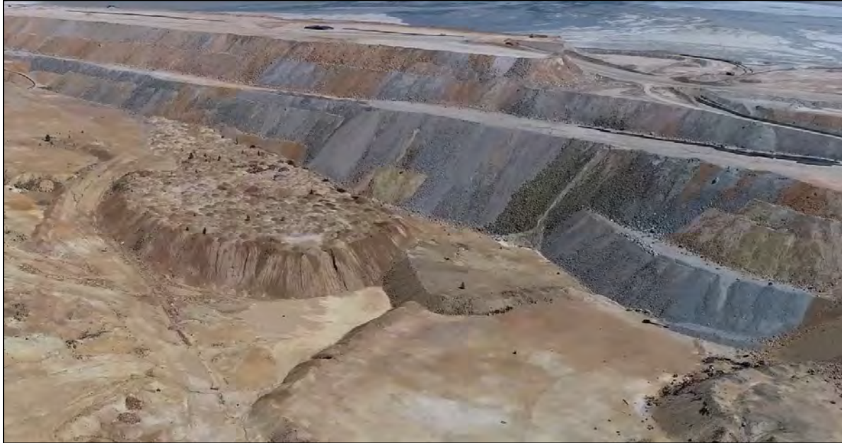
PHOTO 17 – East-West Embankment downstream slope along the northwest dumps area.
