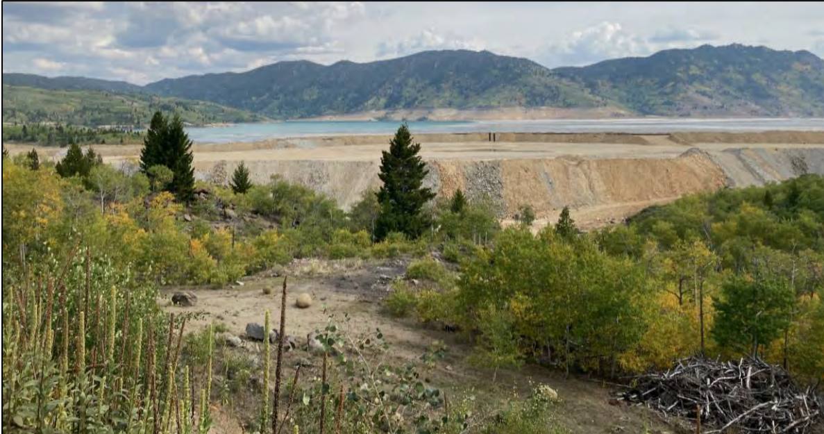
PHOTO 51 – Downstream side of the West Embankment, facing east from West Ridge topsoil stockpile.
