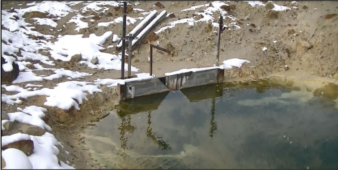
PHOTO 56 – Number 10 Seep V-notch weir and automated level sensor connected to the RMS.
