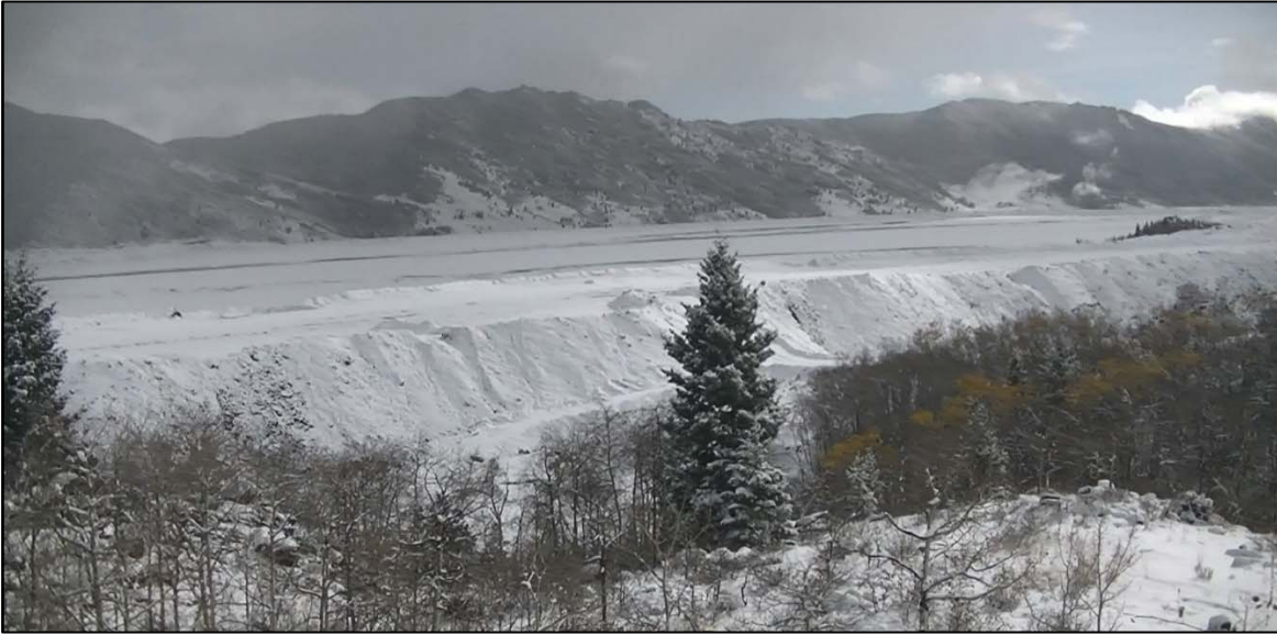
PHOTO 40 – Overview of the snow-covered West Embankment from the West Ridge topsoil stockpile.
