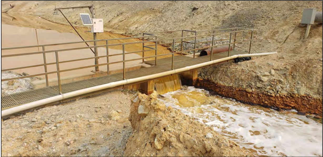
PHOTO 27 – HsB Area – HsB Weir
