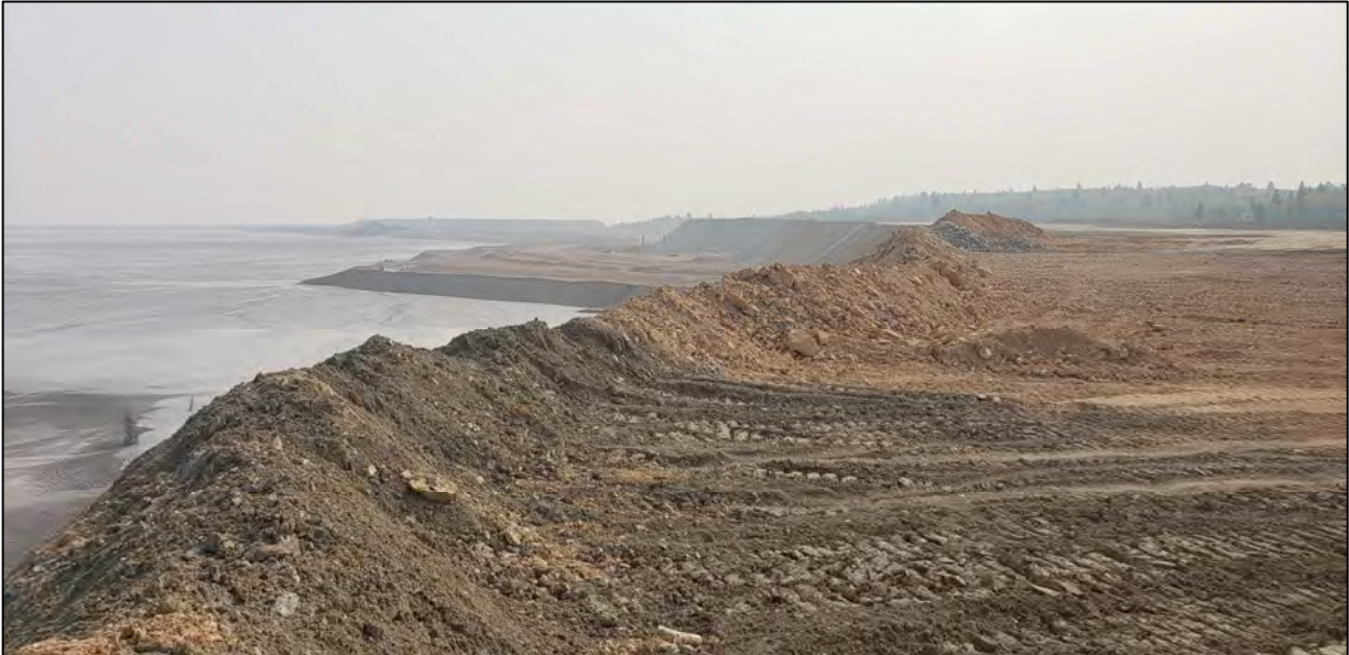
PHOTO 13 – West Embankment – EL 6,450 ft construction progress
