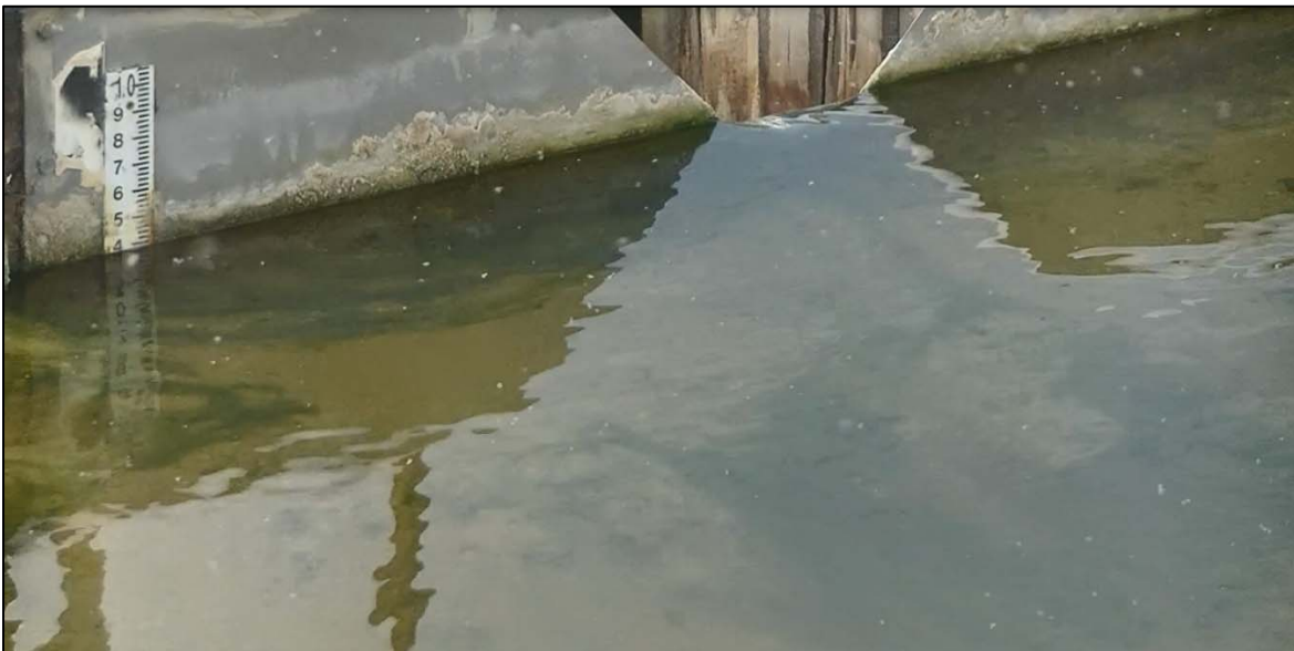
PHOTO 57 – Number 10 Seep V-notch weir staff gauge reading slightly below 0.4.
