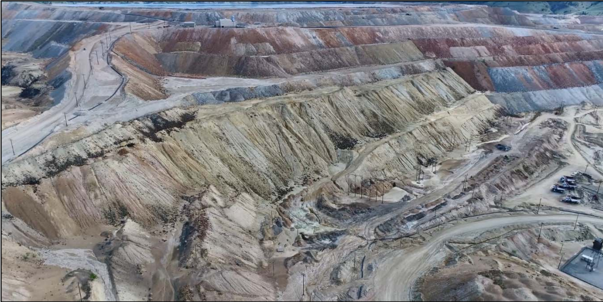
PHOTO 9 – Central pedestal area of the East-West Embankment, looking northeast.
