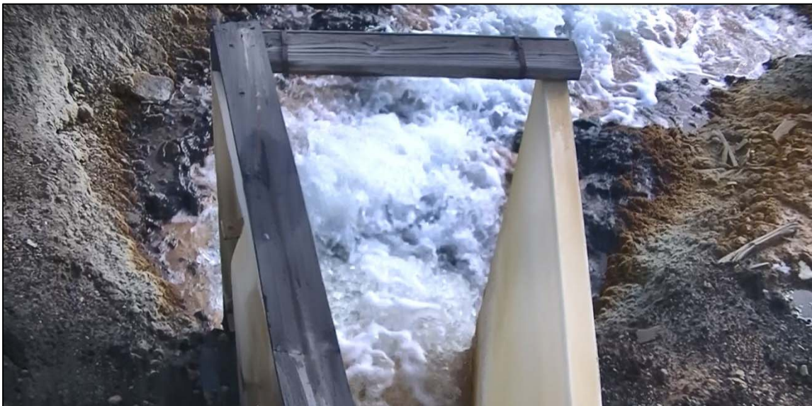
PHOTO 71 – Outlet of Parshall flume providing measurement of Cell 10 discharge flow.
