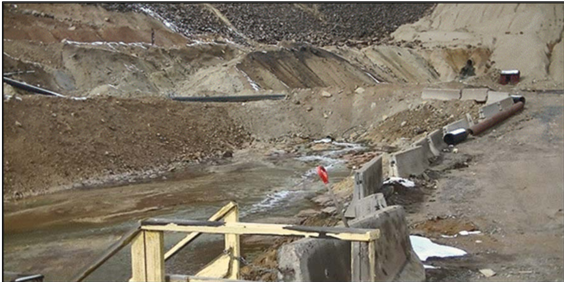
PHOTO 69 – Culvert discharging flow from Upper HsB area to Cell 10 pump area.
