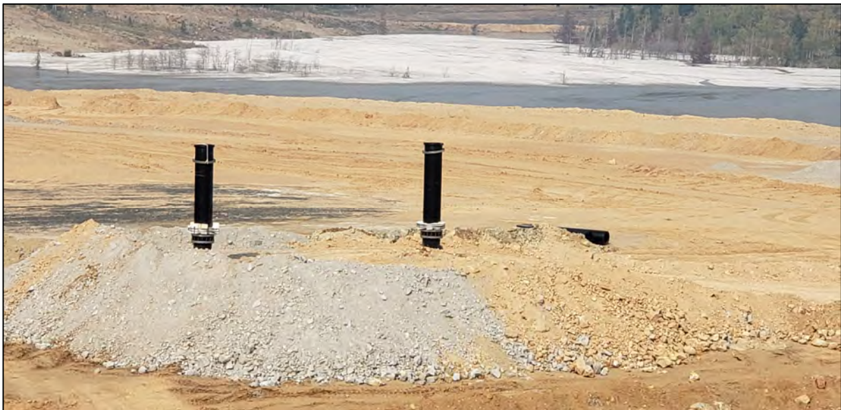
PHOTO 12 – West Embankment – Extraction Basin well risers
