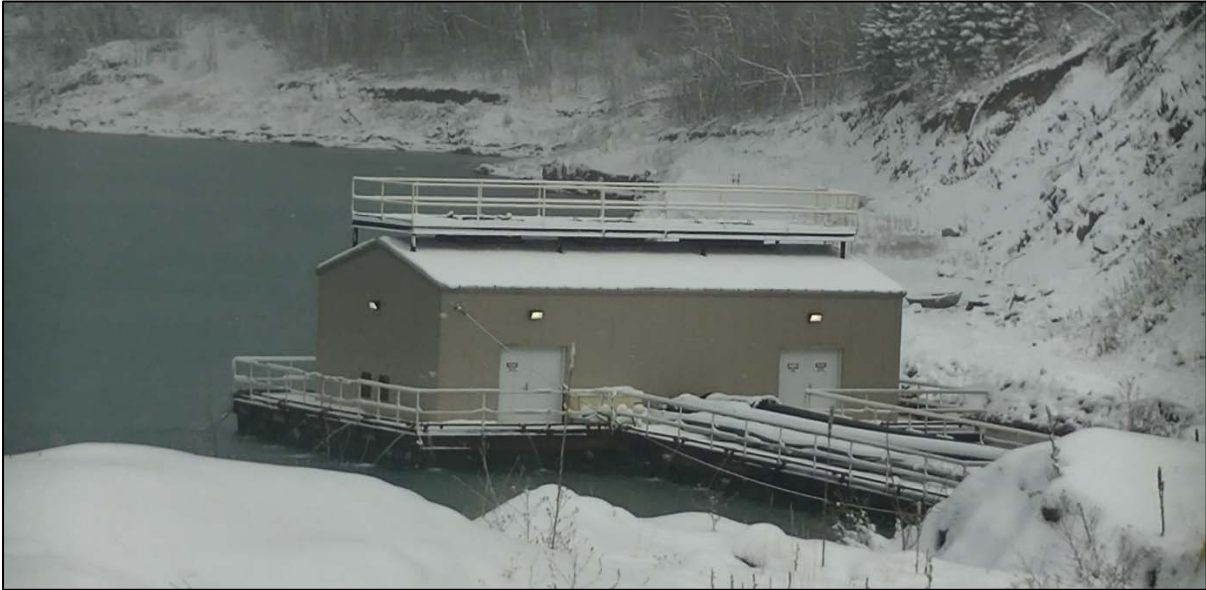
PHOTO 24 – Newer Reclaim Barge.
