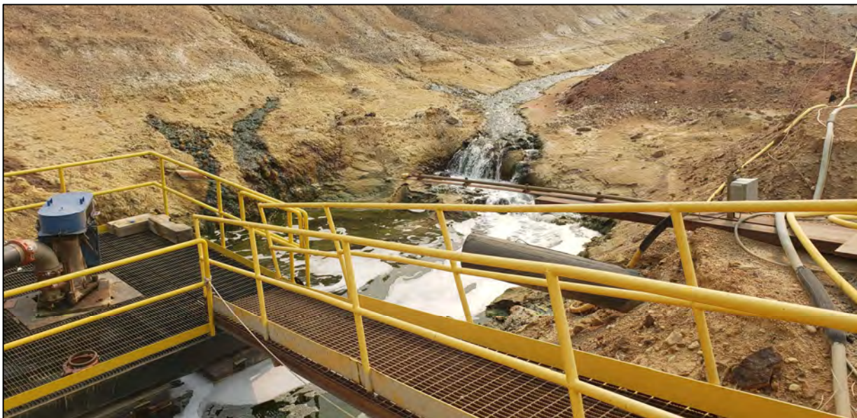
PHOTO 30 – HsB Area – Muddler Pump and overflow pipeline
