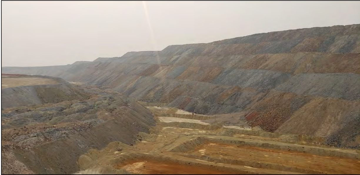
PHOTO 1 – North-South Embankment – Downstream step-out overview
