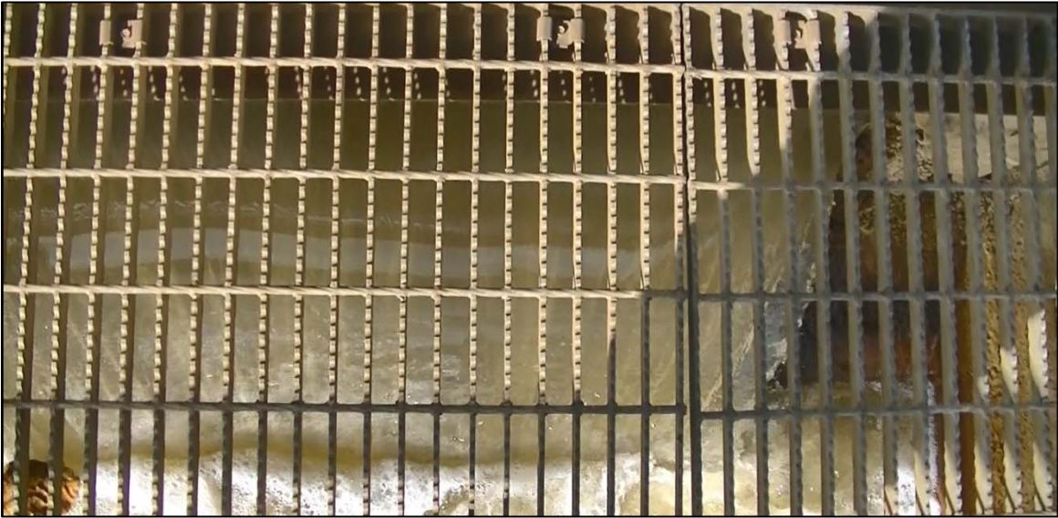
PHOTO 74 – Flow through the HsB Weir.
