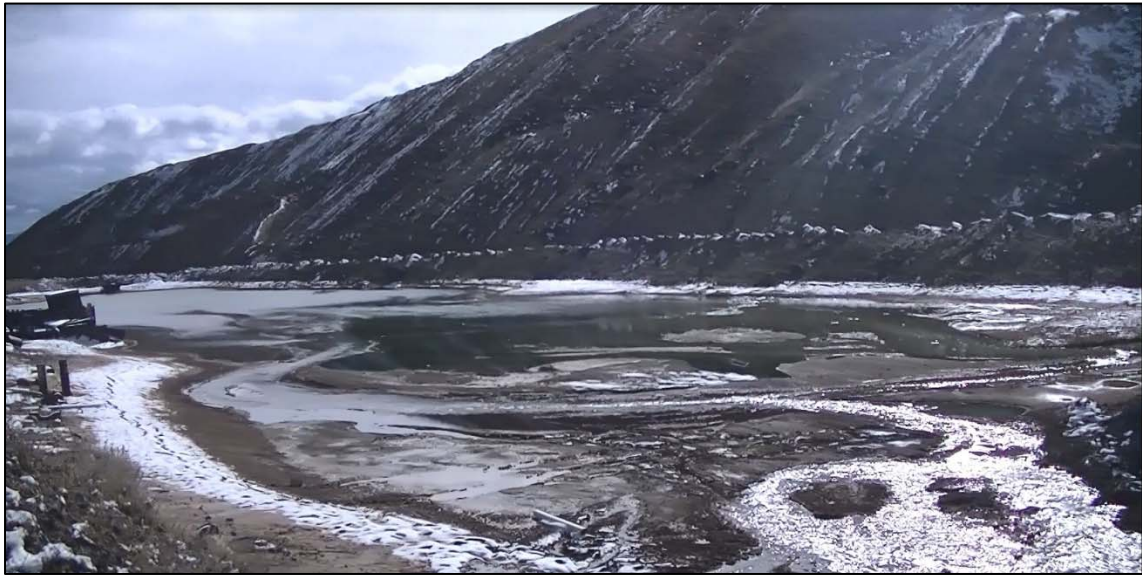
PHOTO 72 – West side of the Upper HsB Pond.
