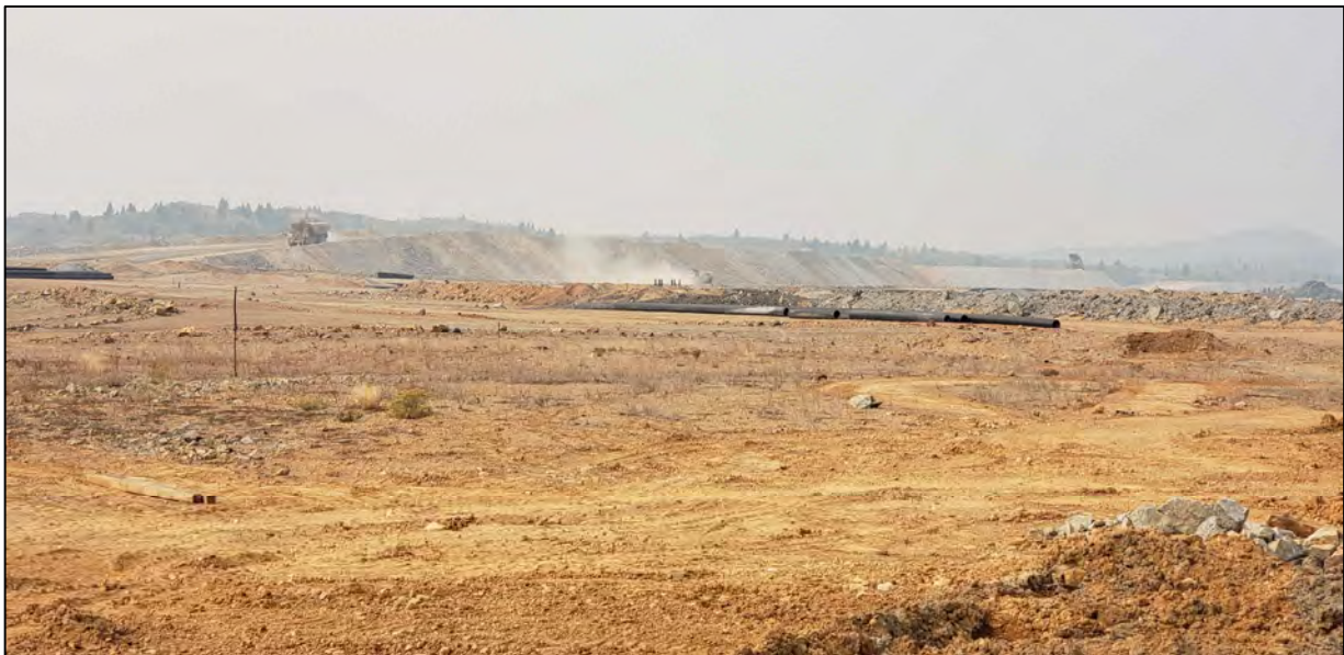
PHOTO 6 – East-West Embankment – EL 6,450 ft construction progress
