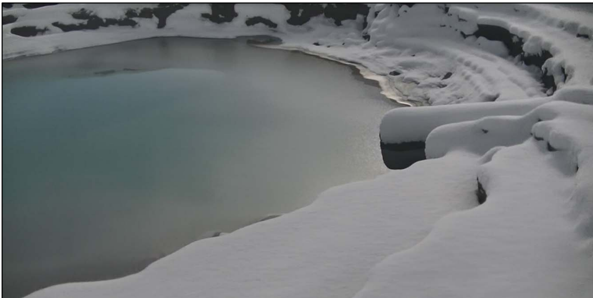
PHOTO 39 – Discharge location RK-4.
