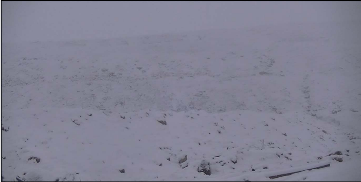
PHOTO 22 – Snow-covered slope of North-South Embankment downstream side, looking north.
