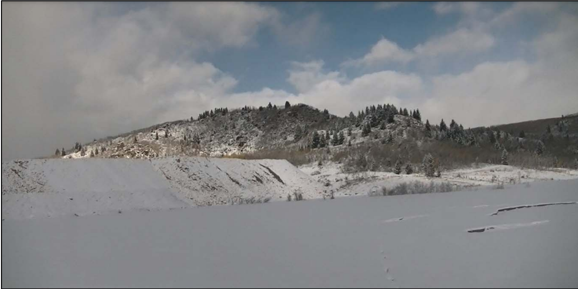
PHOTO 38 – Recently constructed EL. 6,450 ft lift at northern end of West Embankment.
