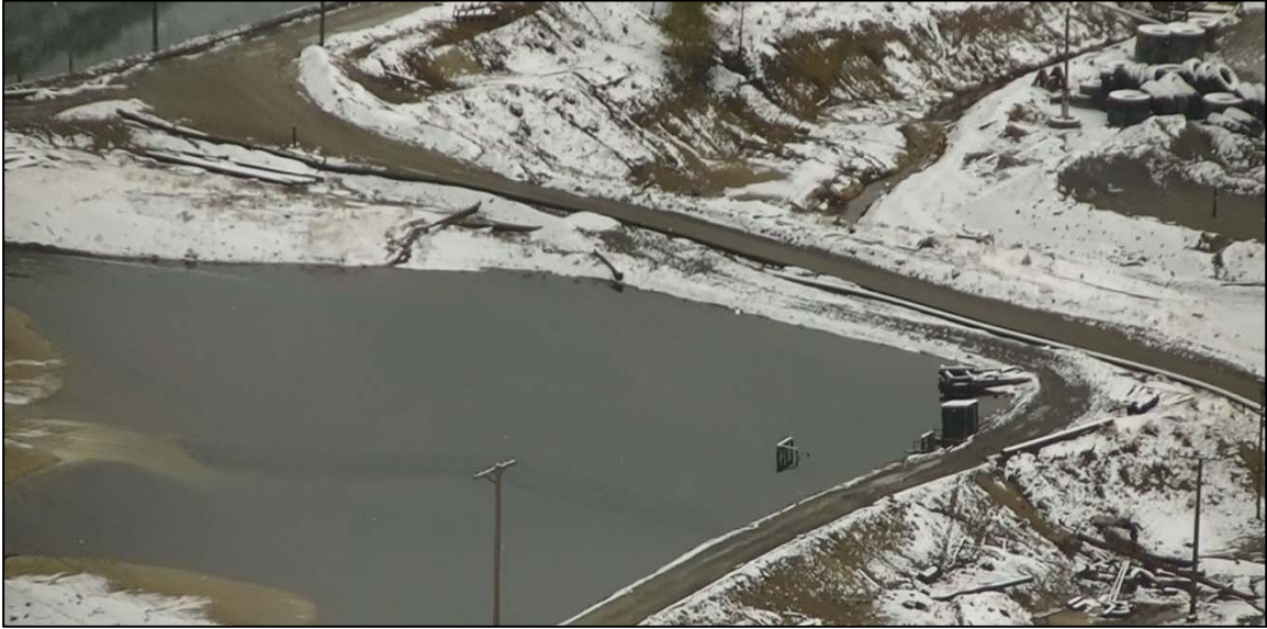
PHOTO 48 – Surge Pond in the HsB Area, looking southeast from No. 3 (Tailings) Booster Pump House viewpoint.
