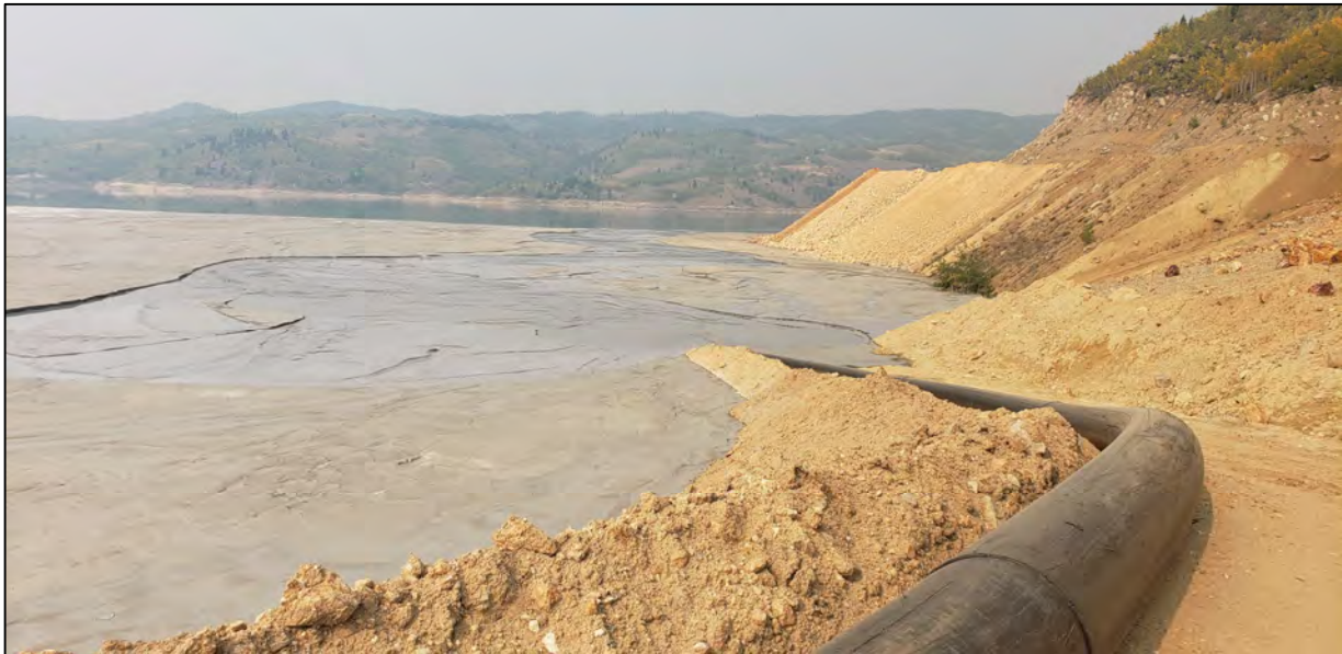
PHOTO 2 – North-South Embankment – Tailings discharge NS-4 and supernatant pond location
