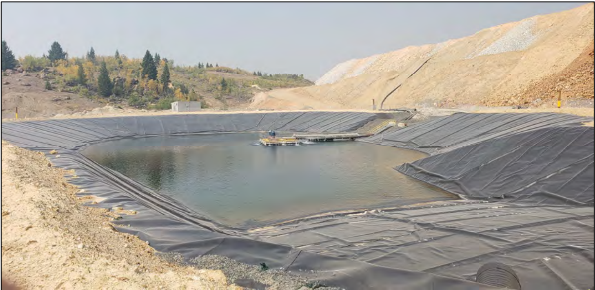
PHOTO 14 – West Embankment – Extraction Pond
