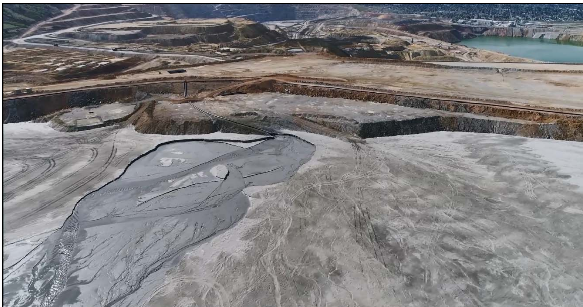
PHOTO 8 – Discharge location NS-1 along the North-South Embankment facing southeast.
