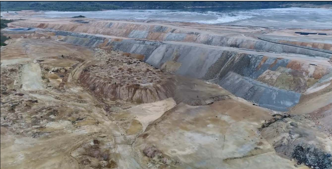
PHOTO 12 – East-West Embankment downstream slope along the northwest dumps area.
