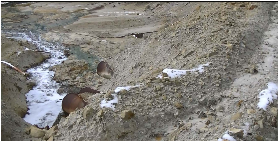
PHOTO 31 – Combined seepage (leach seeps) going towards Precipitation Plant in HsB Area at downstream toe of East-West Embankment maximum section, looking west.
