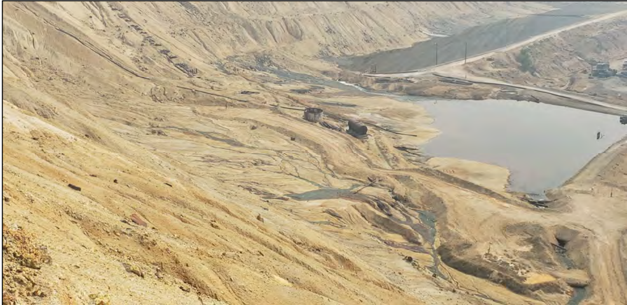
PHOTO 17 – HsB Area – Leach seeps along toe of East-West Embankment viewed from Seep 10 bench
