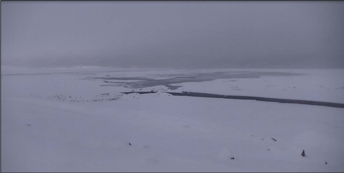
PHOTO 28 – Tailings flow over snow-covered tailings beach between the North-South and East-West Embankments.
