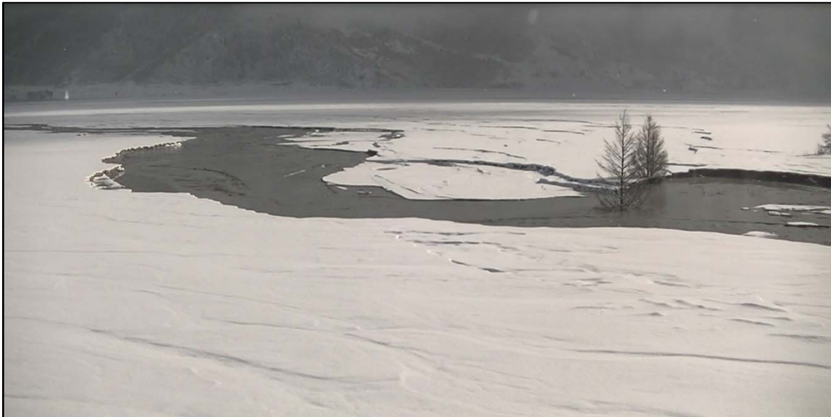
PHOTO 35 – Tailings flow from discharge location RK-1 over snow-covered tailings beach.
