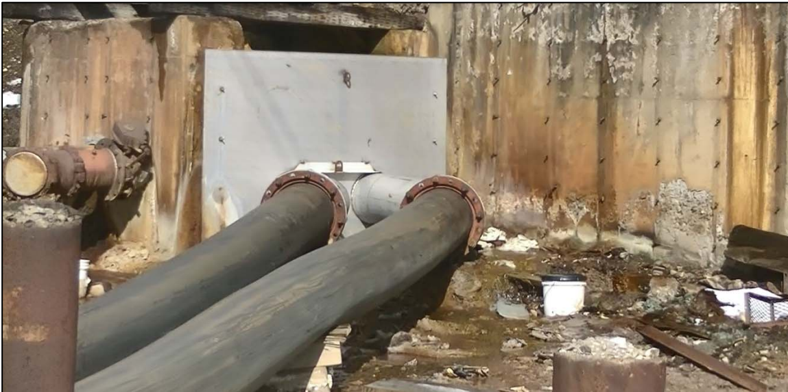
PHOTO 65 – Bulkhead replacement for discharge lines from the #5 and #6 Cells.
