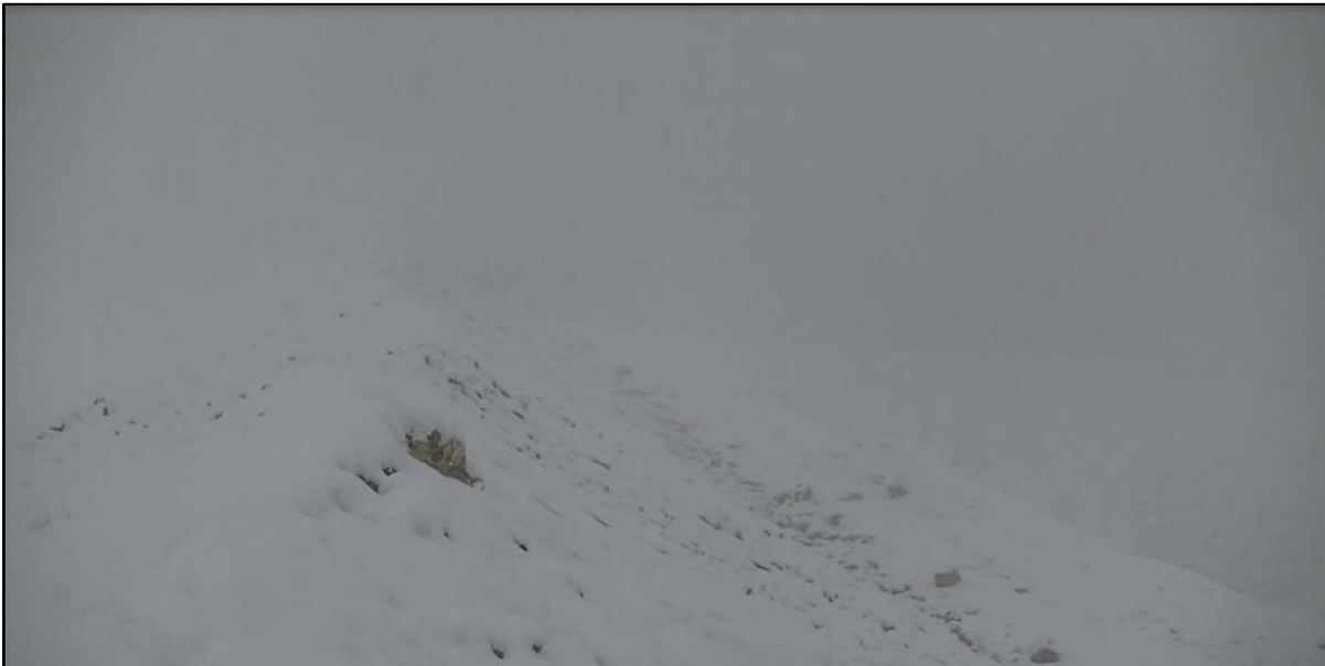
PHOTO 23 – Snow-covered North-South Embankment at step-out, looking north.
