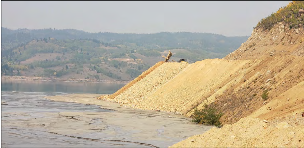
PHOTO 3 – North-South Embankment – Road widening to accommodate realignment of the Reclaim Water Pipeline
