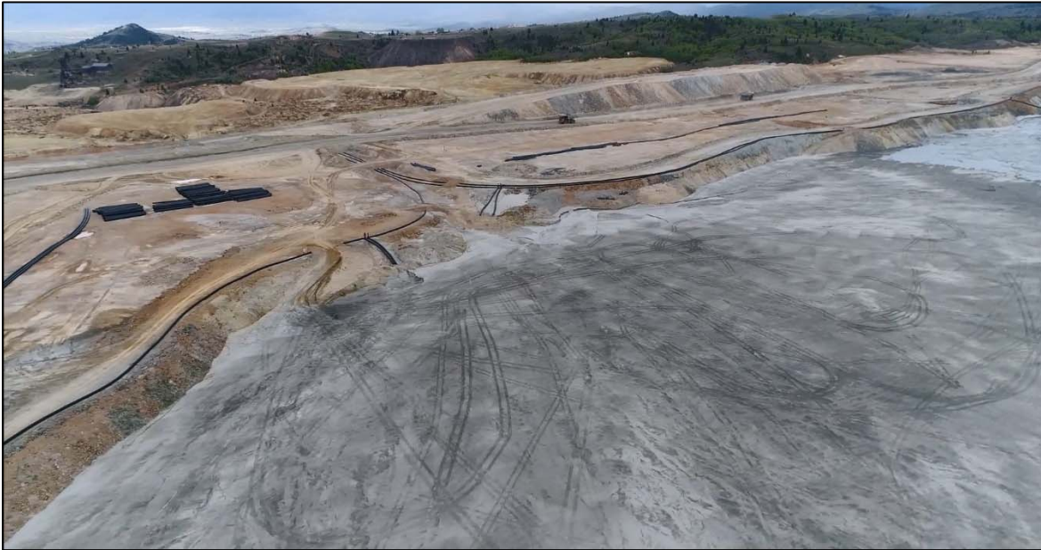
PHOTO 13 – East-West Embankment upstream face at discharge location EW-1 facing west.
