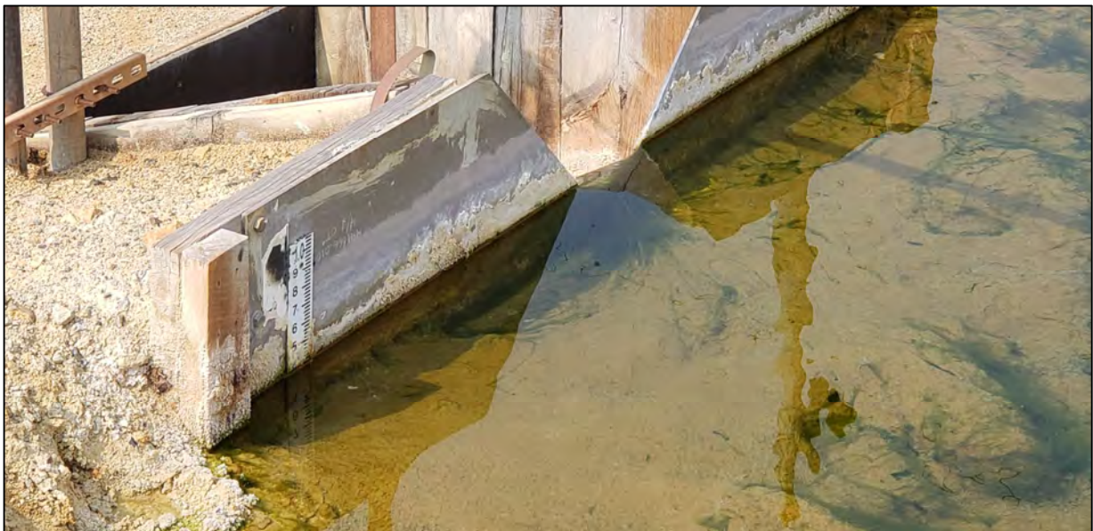
PHOTO 22 – Seep 10 Weir Staff Gauge reading approximately 0.4
