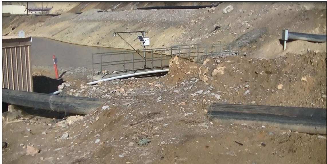
PHOTO 73 – HsB Pond and Weir.
