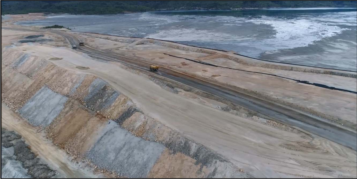
PHOTO 11 – East-West Embankment and rockfill surcharge near discharge location EW-2, looking north.
