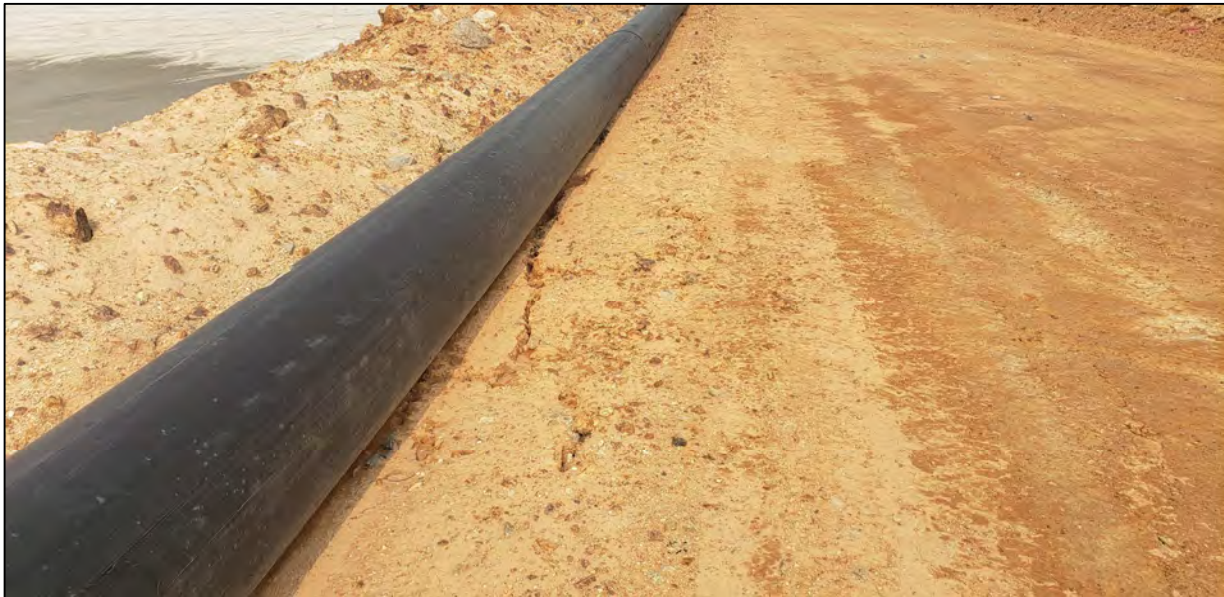
PHOTO 4 – North-South Embankment – Example of cracking along the upstream edge of the tailings discharge corridor
