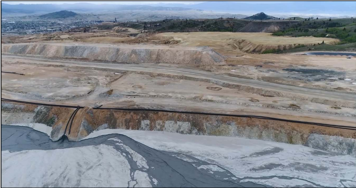
PHOTO 15 – East-West Embankment upstream side at discharge location EW-2.
