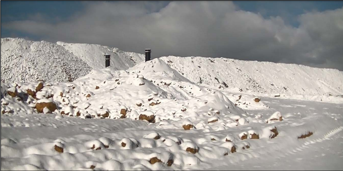
PHOTO 36 – Riser pipes from the Extraction Basin along the West Embankment, EL. 6,450 ft lift construction in the background.
