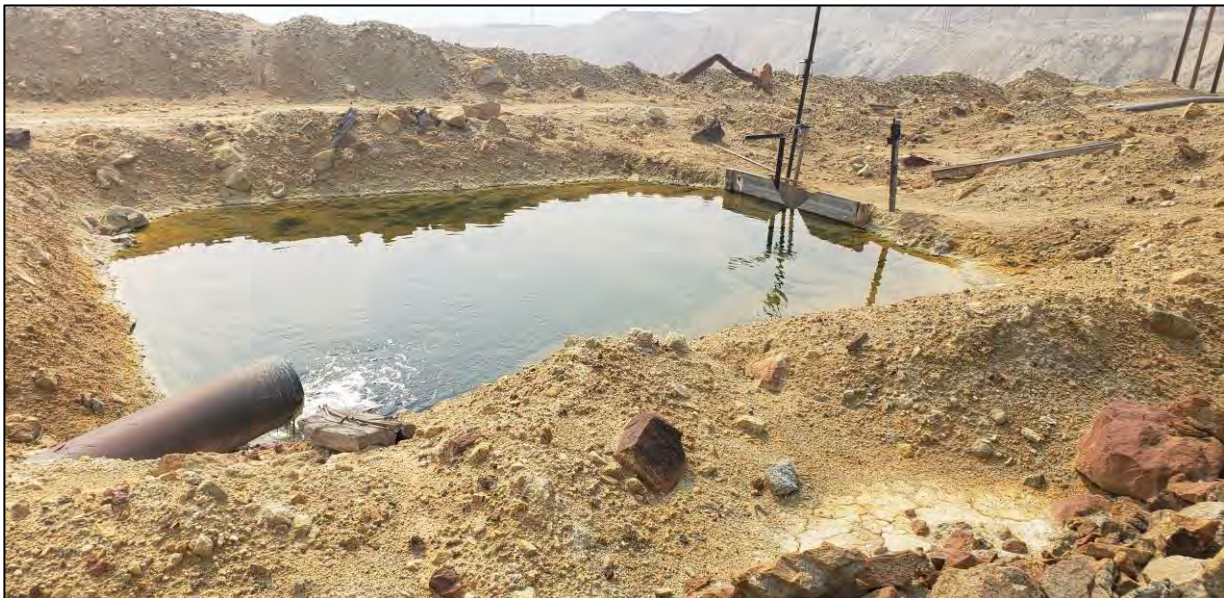
PHOTO 2 – Sep 16, 2020 – Seep 10 Stilling Pond.
