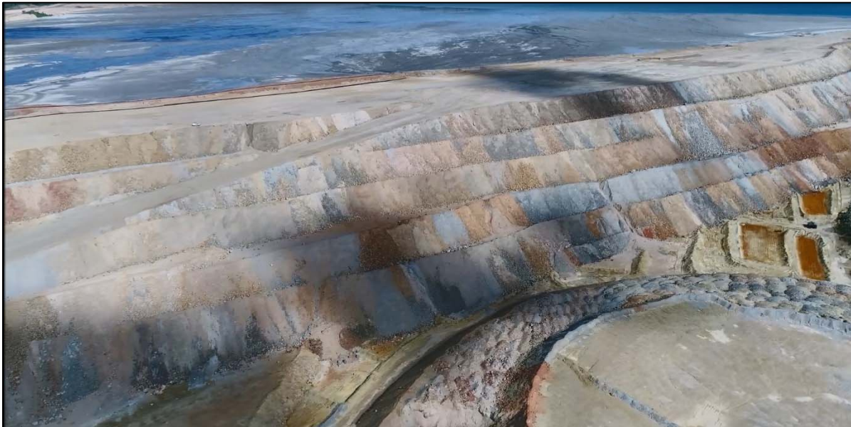
PHOTO 2 – North-South Embankment downstream shell, looking northwest towards the top of the new mine haul ramp at EL. 6,400 ft
