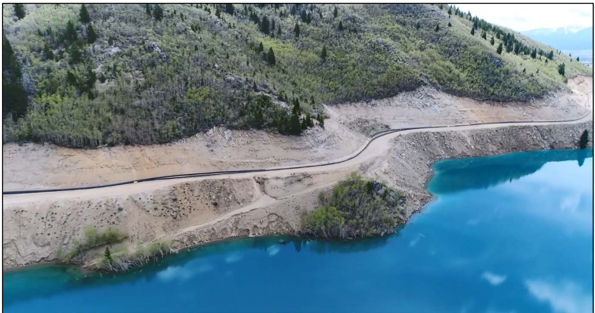
PHOTO 4 – Reclaim water pipeline road.
