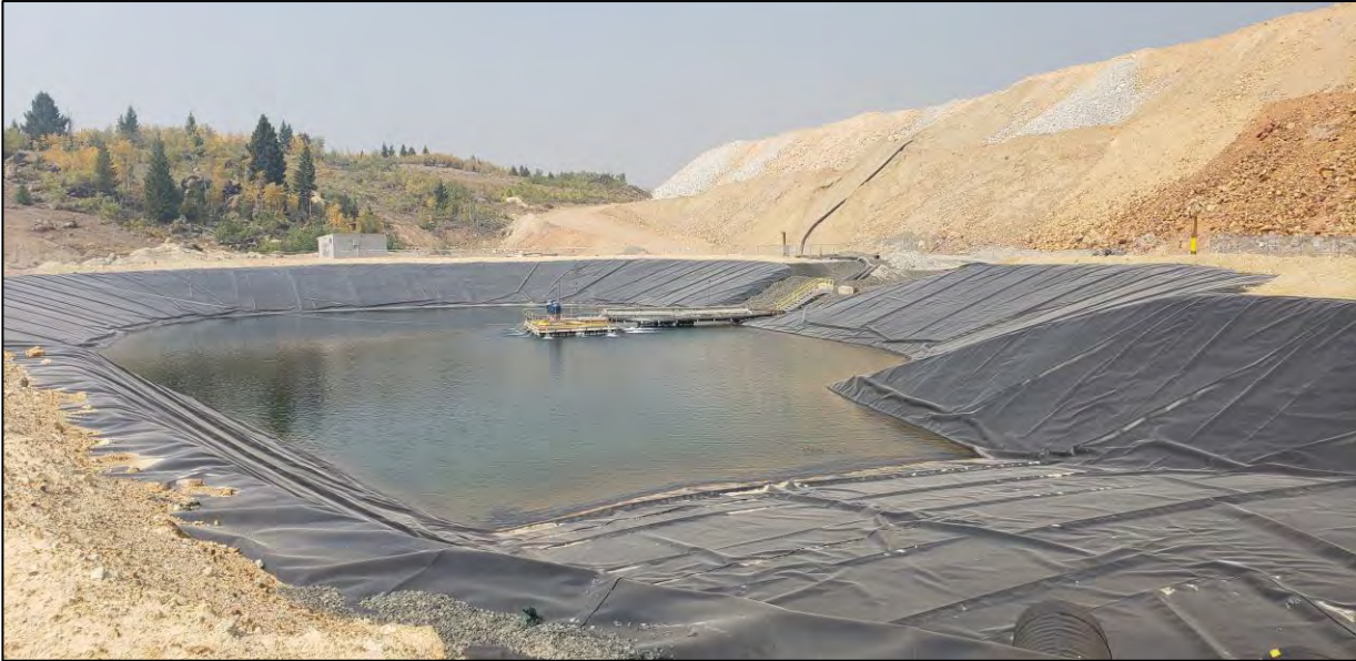
PHOTO 13 – Sep 16, 2020 – WED Extraction Pond and Dewatering System.
