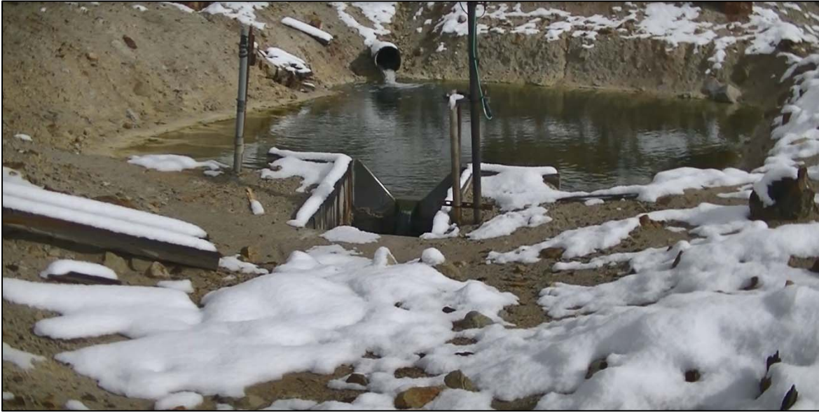
PHOTO 58 – Overview of Number 10 Seep stilling pond.
